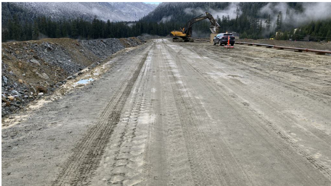
Photograph 10: Crest of South Arm looking west – Crest raise to El. 378 m complete, including capping layer to 378.5 m. Safety berm in place on downstream
