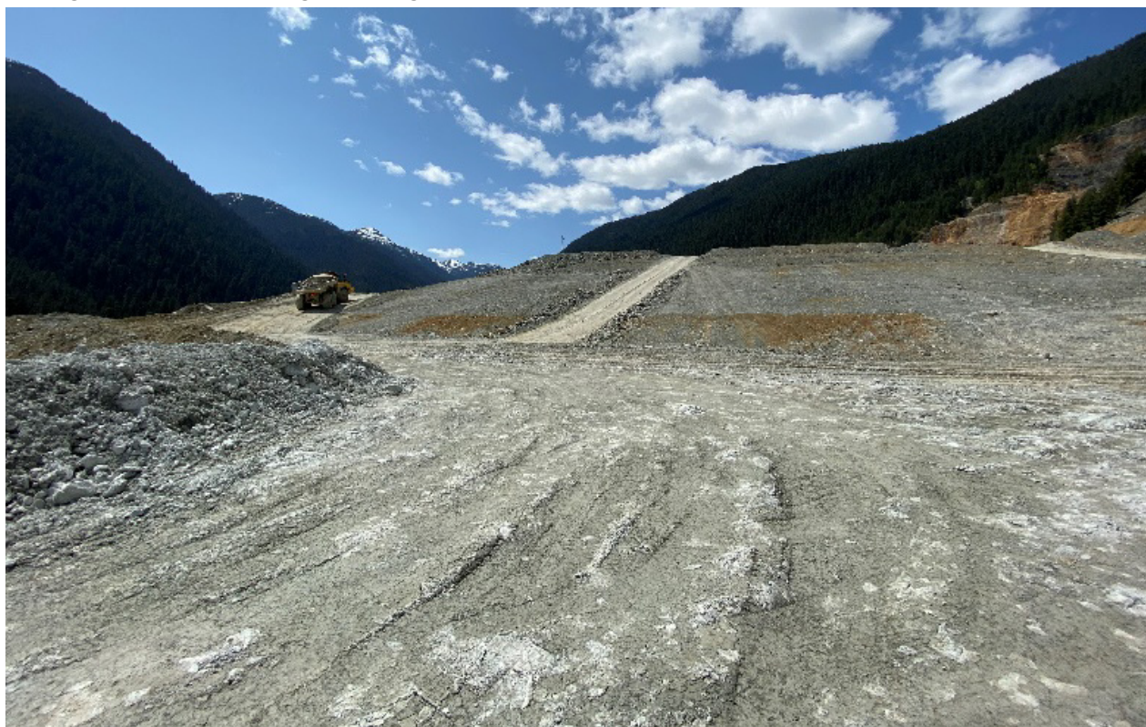
Photograph 4: Downstream slope of 4H:1V east arm downstream slope, looking west. Truck hauling Zone A for raising of south arm downstream shell
