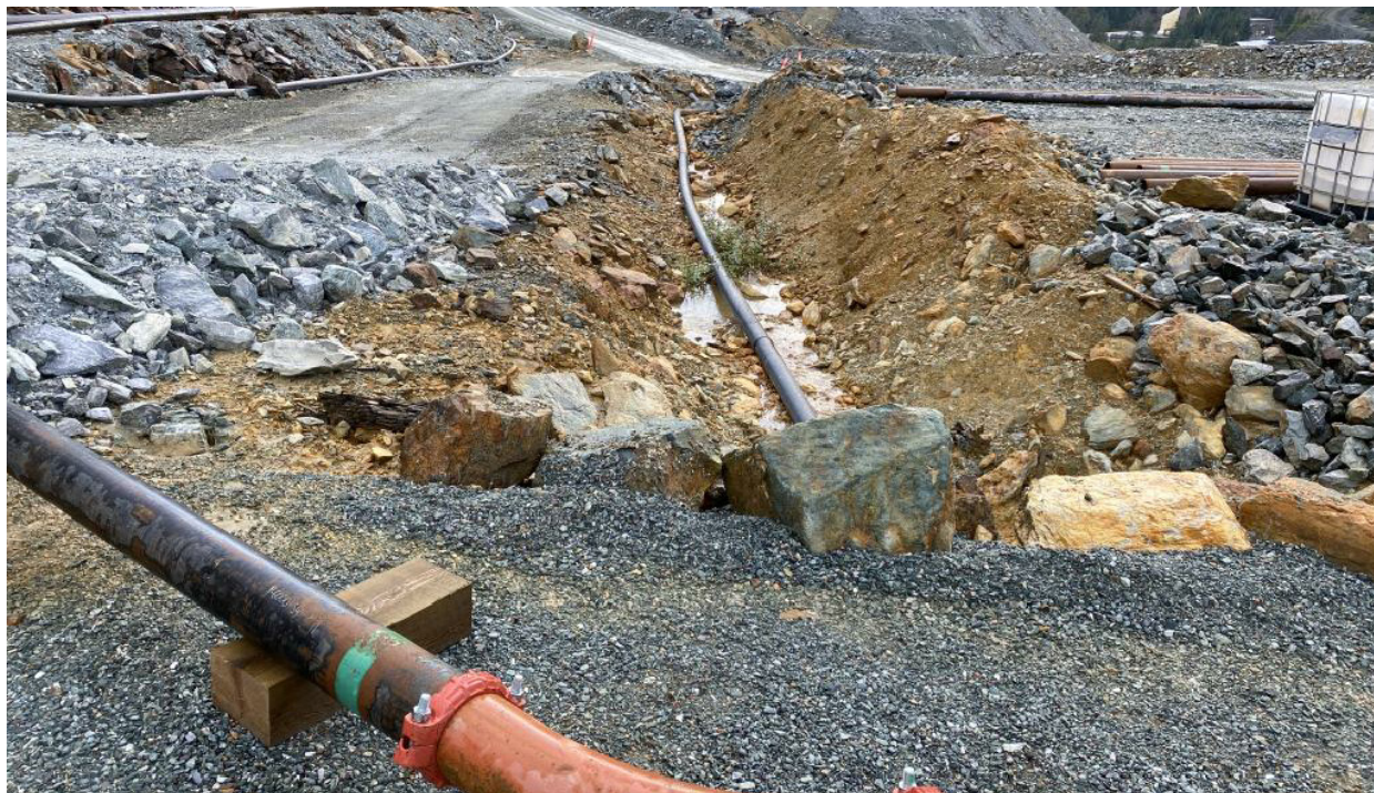
Photograph 6: Run-off water from WRD2 being directed over crest near East Arm abutment, looking east
