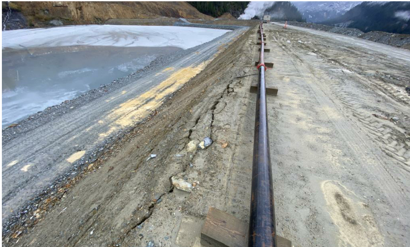
Photograph 9: Cracking in Temporary upstream slope on South Arm looking east
