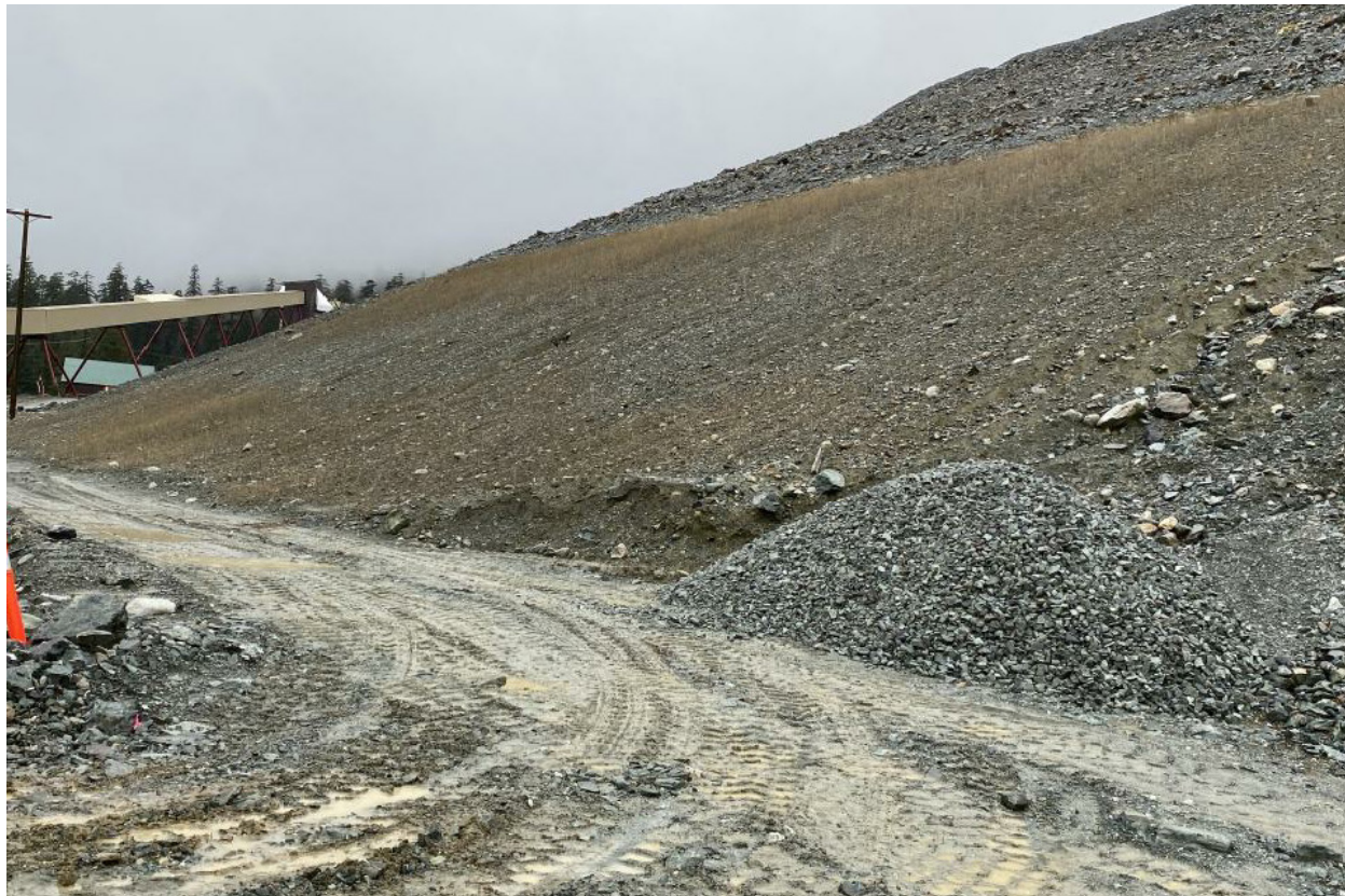
Photograph 5: Cover Trials on Downstream Slope at southwest corner of facility, looking northwest
