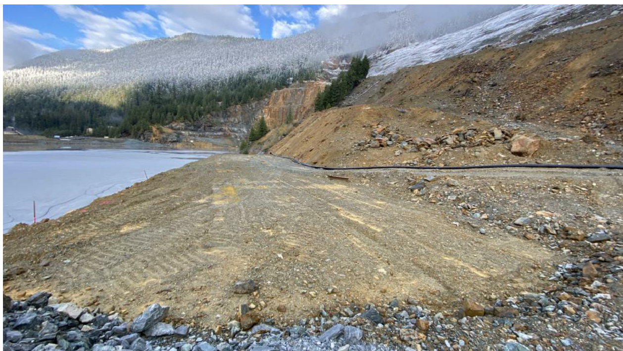
Photograph 12: North Abutment WRD1 Zone J filter at El. 378. Looking west.
