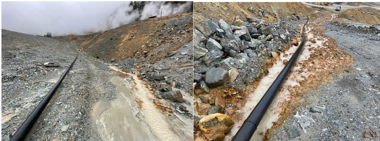
Photograph 7: Run-off water from WRD2 flowing down toe of 4H:1V East Arm and WRD1
