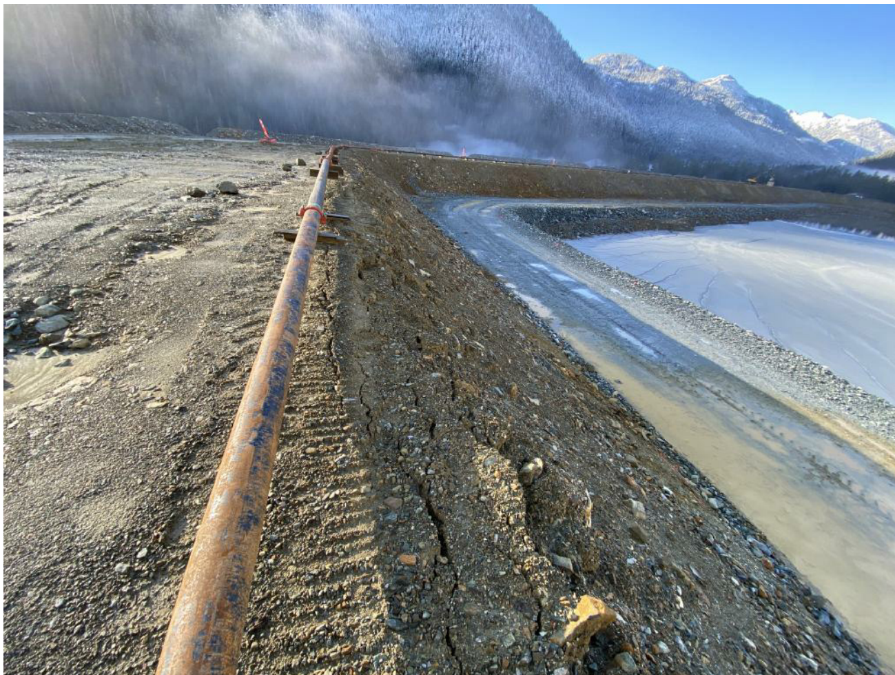
Photograph 8: Cracking in Temporary upstream slope on East Arm looking south
