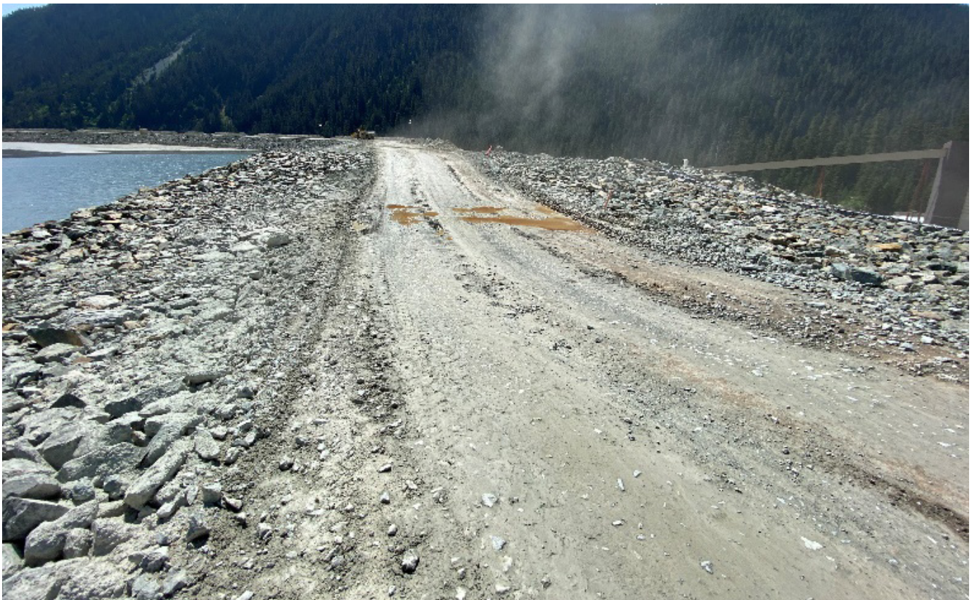
Photograph 2: Operational spillway across 373.5 m crest of west arm dam, looking south
