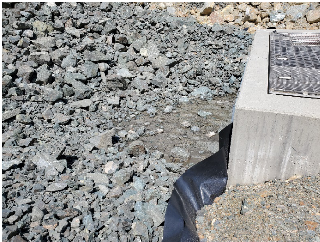
Photograph 5: Clear seepage flow entering Lynx Springs Drain
