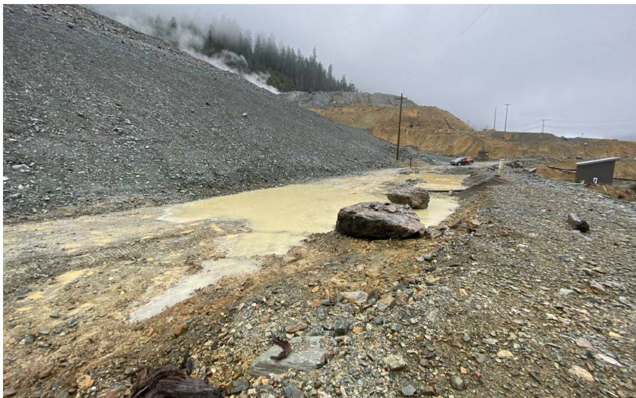
Photograph 4: Water ponding at southeast toe of dam, looking east
