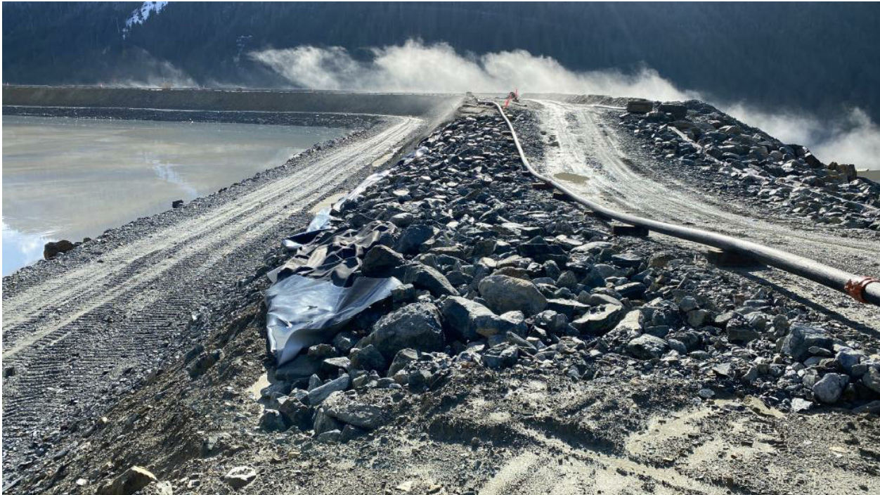
Photograph 17: Spillway invert across West Arm crest, looking south. Upstream push out not complete
