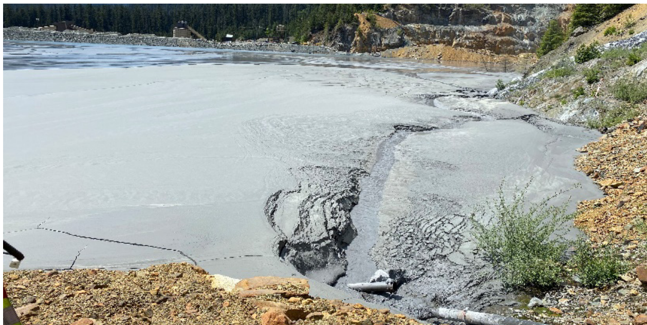
Photograph 3: Point discharge of tailings off of WRD1 filter upstream of east arm abutment
