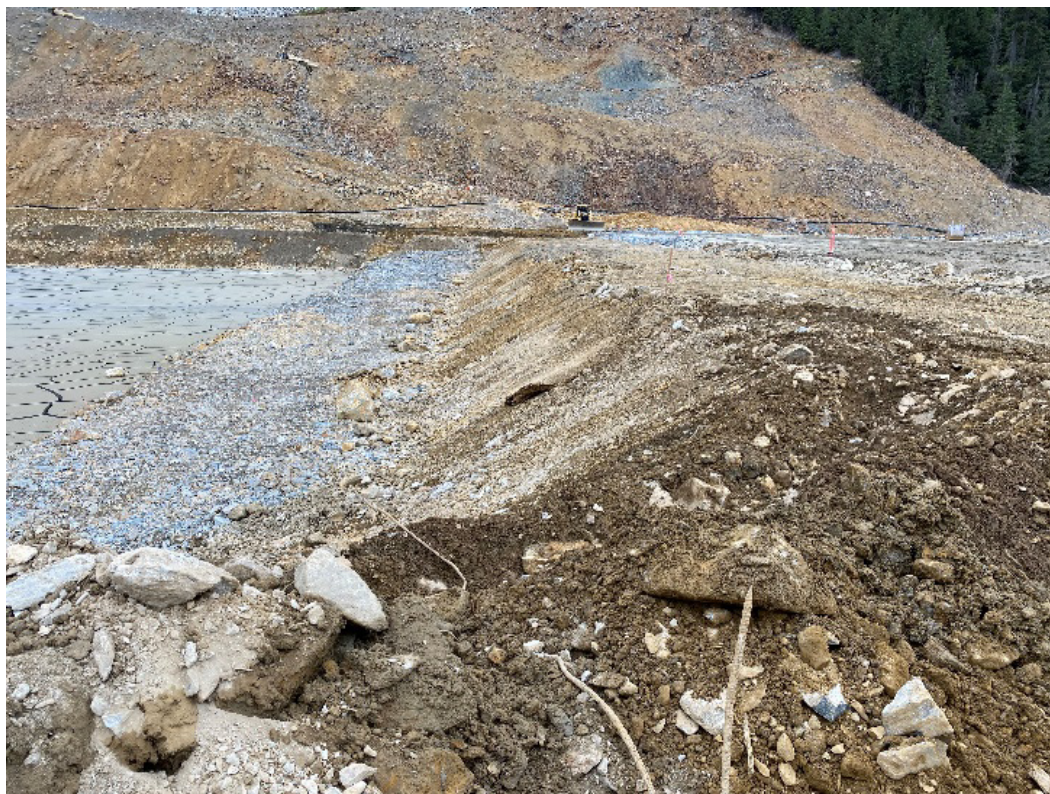
Photograph 5: Temporary over steepened upstream slope constructed to facilitate crest raise to El. 378 m ahead of constructing shell push out over tailings. Initial lift of push out complete
