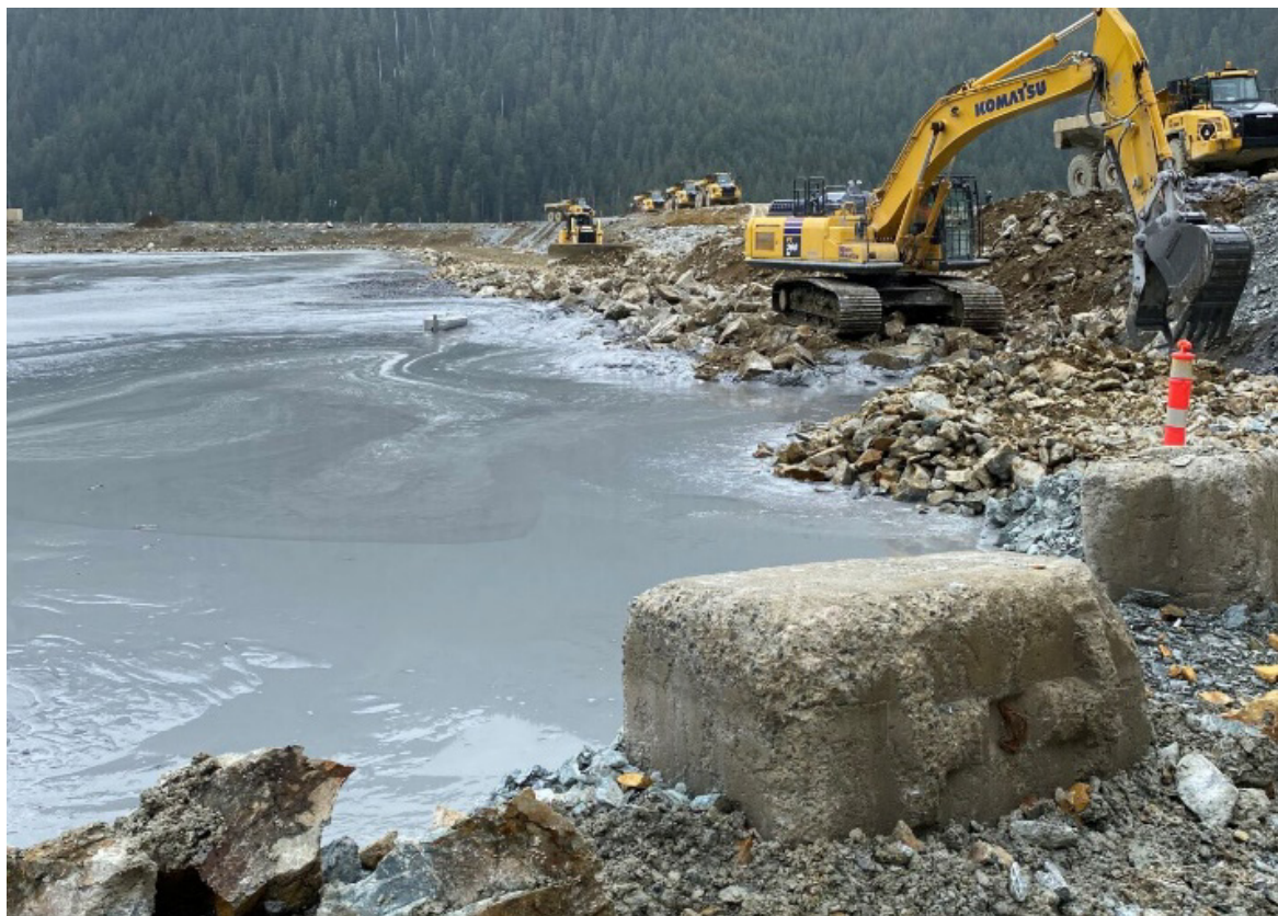
Photograph 1: Excavator placing boulders for initial lift of push out on tailings, looking south from upstream side of west arm abutment. D6 dozer in background placing Zone A rockfill over material initially placed by excavator
