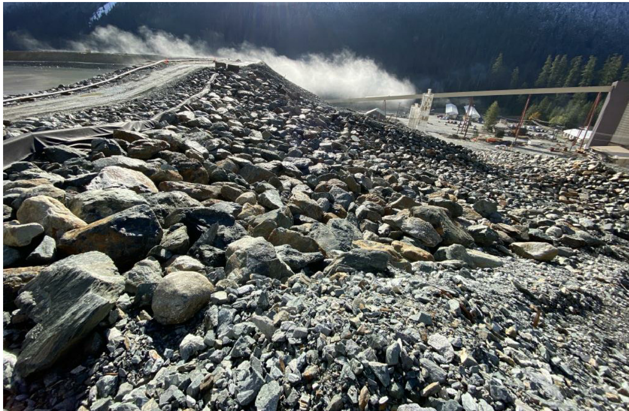
Photograph 19: Spillway channel on downstream slope of West Arm, looking south
