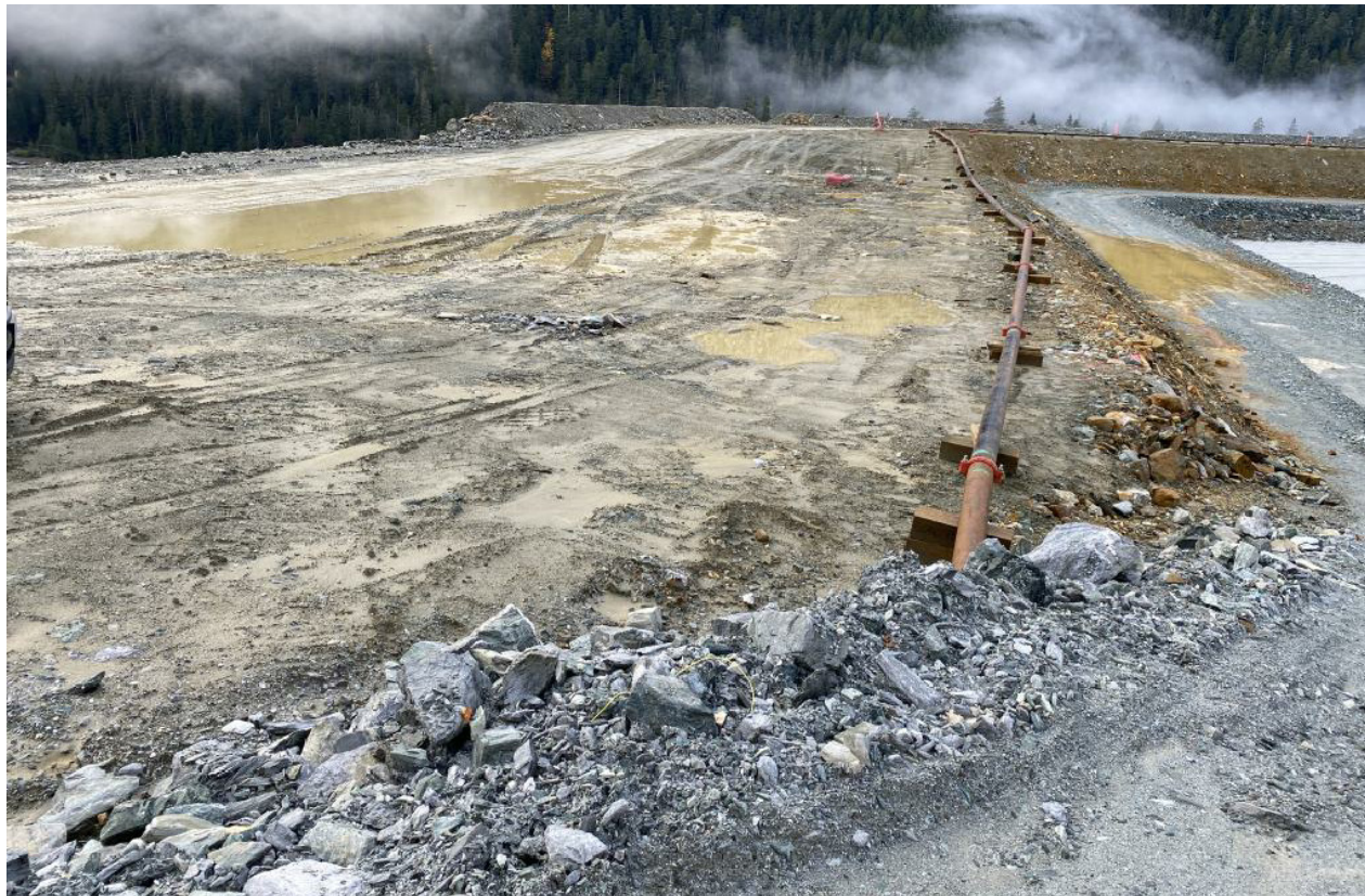
Photograph 11: Auxiliary Swale on East Arm looking south. Minor ponding within swale
