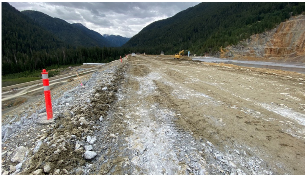
Photograph 4: Crest of south arm dam looking west. Crest raise to El. 378 m in progress
