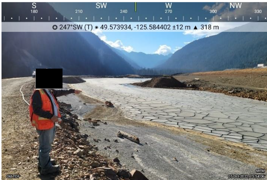
Photo 15: East Strip of the Old TDF continues to be filled with tailings. Tailings should be removed prior to onset of wet weather. (October 5, 2022)
