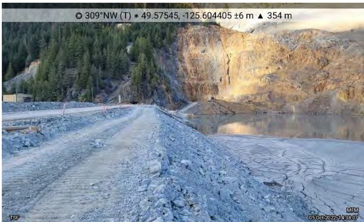
Photo 2: Lynx TDF looking northwest. Crest elevation is at 373.5 m.
