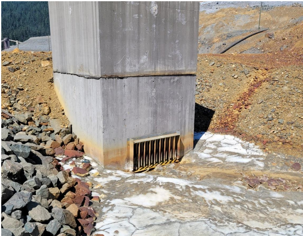
Photo 13: East decant structure with approximately half of the bottom 2 cm's of the vertical grating bars being dissolved. (July 26, 2022)
