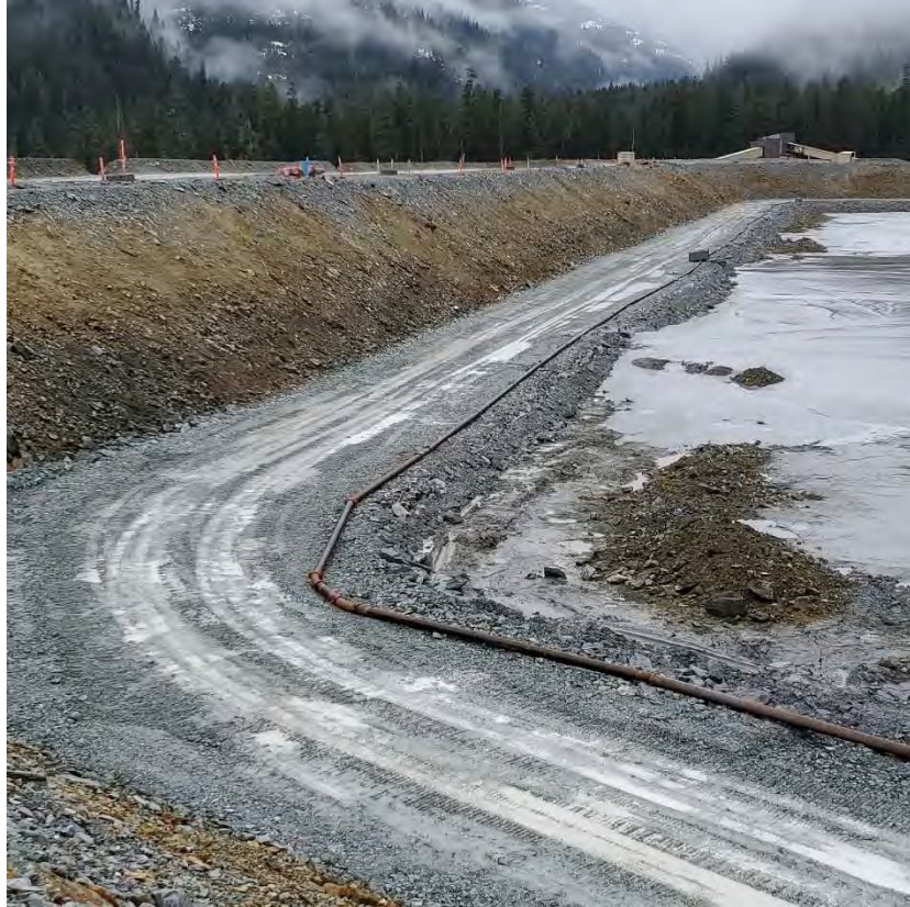
Photo 7: South-east corner of Lynx TDF, looking west. Crest Elevation at 373.5m. Active tailings deposition was observed from a spigot located at the east end of the TDF. (March 22, 2022)
