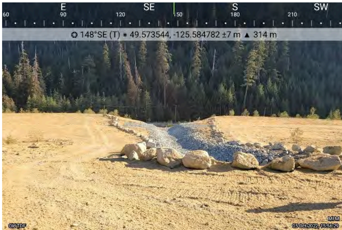
Photo 14: Old TDF Channel 1 looking downstream. The riprap is stable and in good condition.
