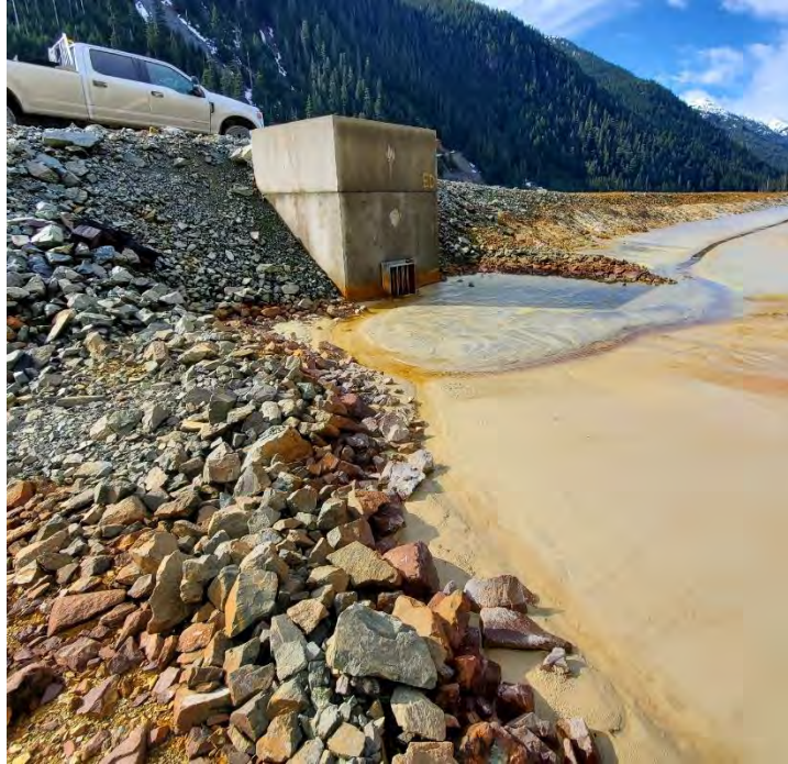
Photo 17: East Decant structure. Grating decant needs to be replaced due to acidic dissolution of lower portion of the vertical grating. (March 23, 2022)
