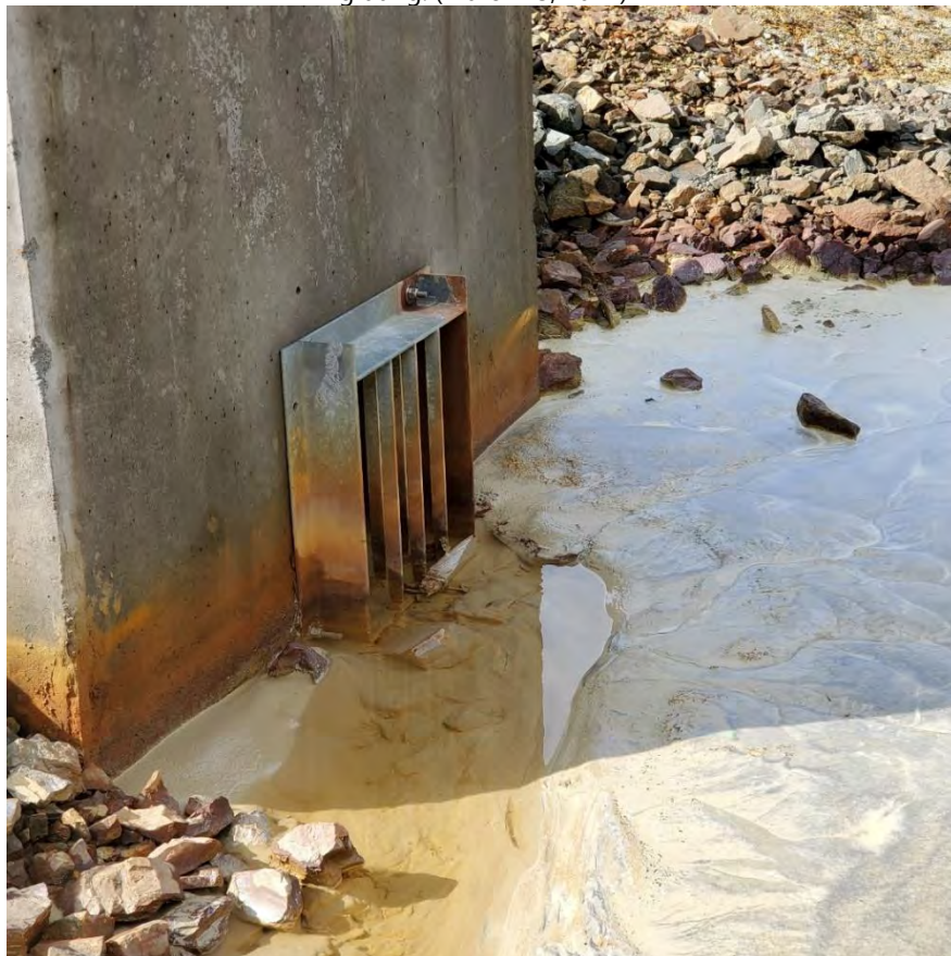
Photo 18: Grating decant needs to be replaced due to acidic dissolution of lower portion of the vertical grating. (March 23, 2022)
