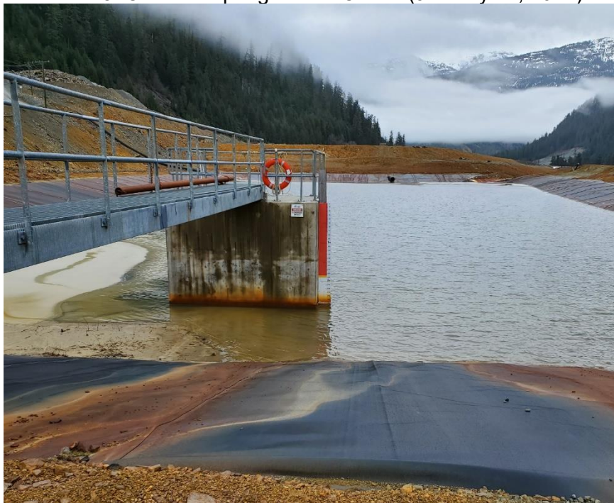
Photo 6: Surge Pond looking east. Sediments from paste plant run off to the left of the control structure seen in photo 6. (March 23, 2022)
