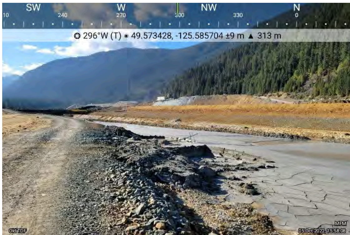
Photo 12: East Strip of the Old TDF continues to be filled with tailings. This conduit needs removal of tailings before the wintertime.
