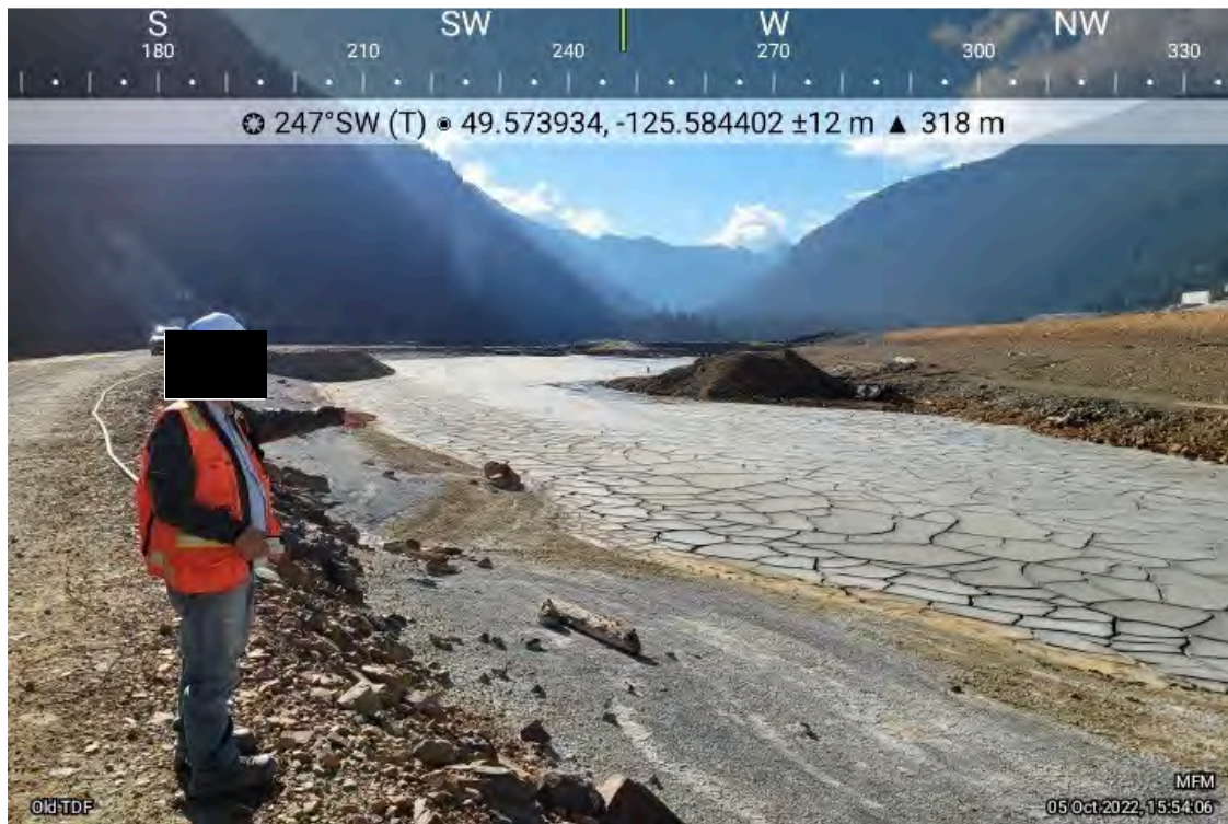
Photo 11: East Strip of the Old TDF continues to be filled with tailings. This conduit needs removal of tailings before the wintertime.
