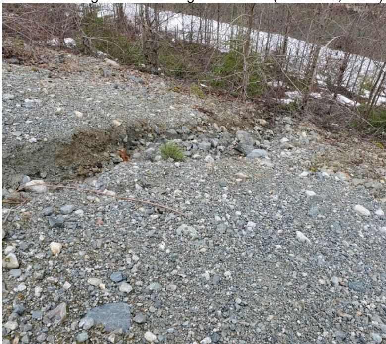
Photo 8: Erosion gullies observed on downstream of SUB to be addressed in 2022 Closure Phase 1 Construction. (March 22, 2022)
