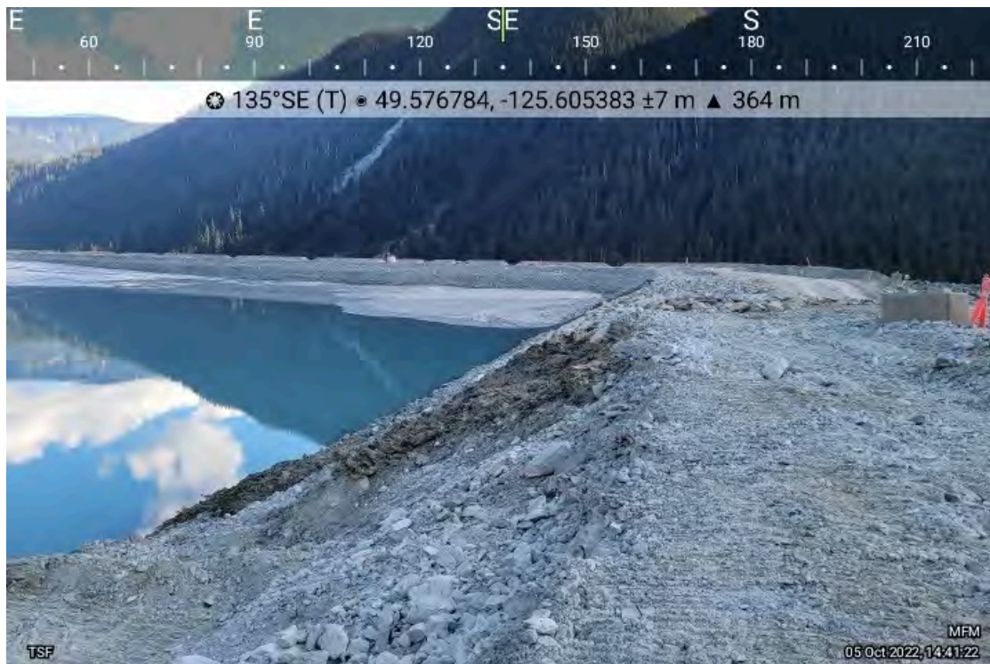
Photo 4: Lynx TDF looking southeast with the boundary of the tailings pond at the west end of the TDF covering about 2/3 of the tailings surface.
