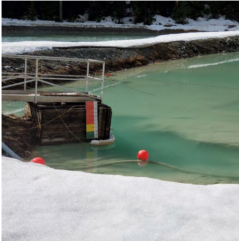
Photo 25: Polishing Pond 2A staff gauge in green zone. (March 23, 2022)
