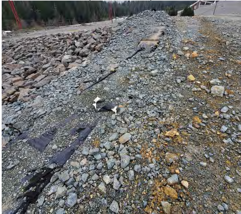
Photo 20: Geotextile/geomembrane over the buried lock blocks in the APA spillway observed to be damaged. (March 22, 2022)
