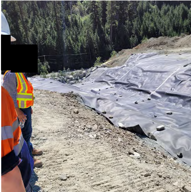
Photo 7: Liner system of the Old TDF spillway
