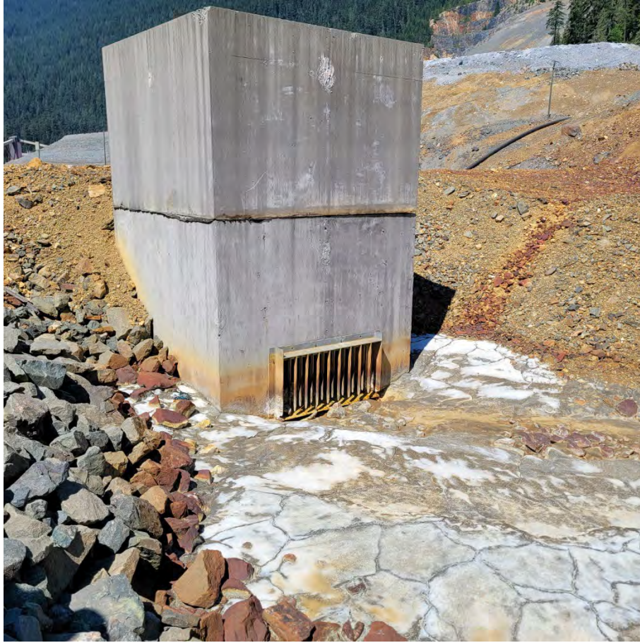
Photo 13: East decant structure with approximately half of the bottom 2 cm's of the vertical grating bars being dissolved.
