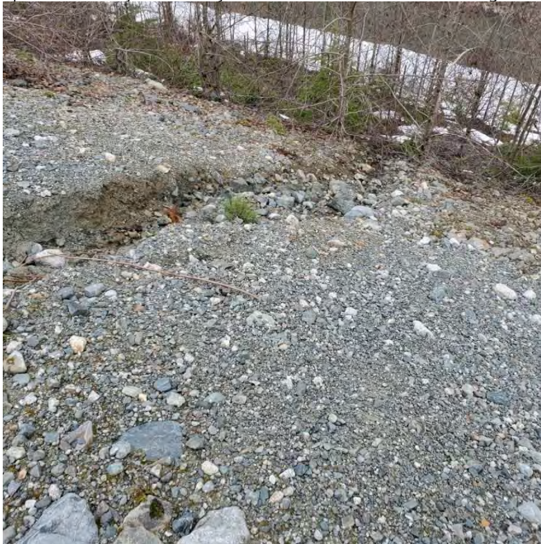
Photo 12: Erosion gullies observed on downstream of SUB to be addressed in 2022 Closure Phase 1 Construction. (March 22, 2022)
