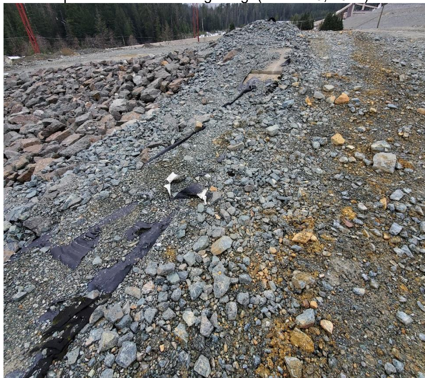
Photo 10: Geotextile/geomembrane over the buried lock blocks in the APA spillway observed to be damaged. (March 22, 2022)
