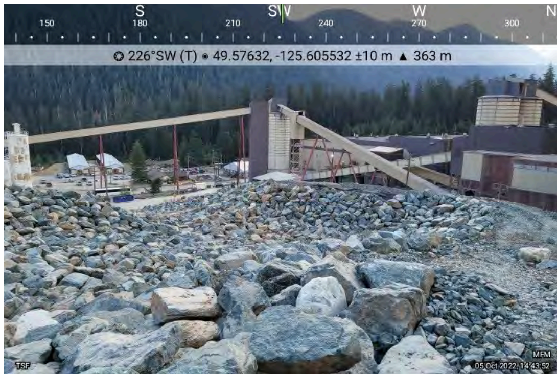
Photo 5: Lynx TDF spillway looking downstream to the mill and camp sites. Riprap was stable with no evidence of deterioration or segregation of sizes. Riprap stones are angular to subangular.
