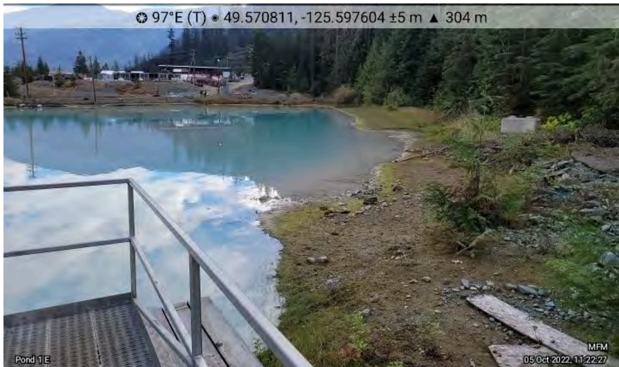
Photo 30: Polishing Pond 1 looking East. No unusual performance was observed. The lateral containment of the south end needs to be assessed against design flows.
