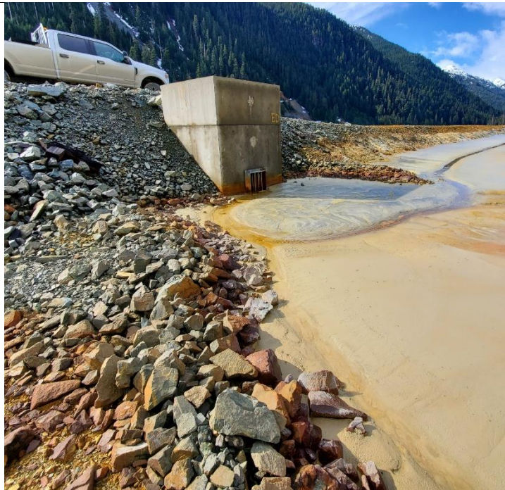
Photo 9: East Decant structure. Grating decant needs to be replaced due to acidic dissolution of lower portion of the vertical grating. (March 23, 2022)
