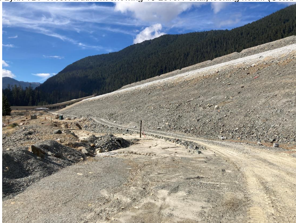
Photo 20: Lynx TDF 2H:1V Downstream dam shell looking north west October 5, 2022)
