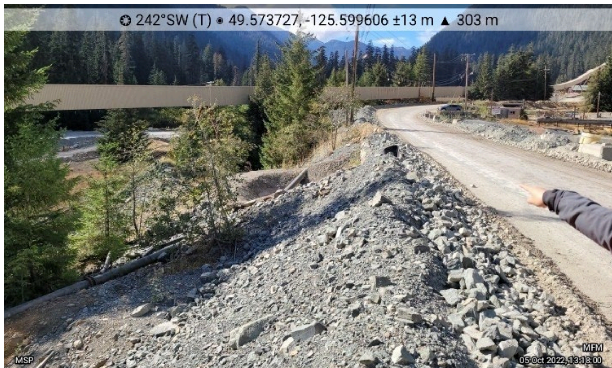
Photo 19: Super Pond looking at the downstream slope and the crest of the south retention berm of Super Pond. No unusual performance was observed.
