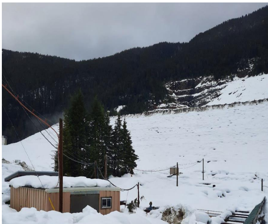
Photo 3: Lynx TDF south-west portion of downstream 2H:1V shell (January 14, 2022)
