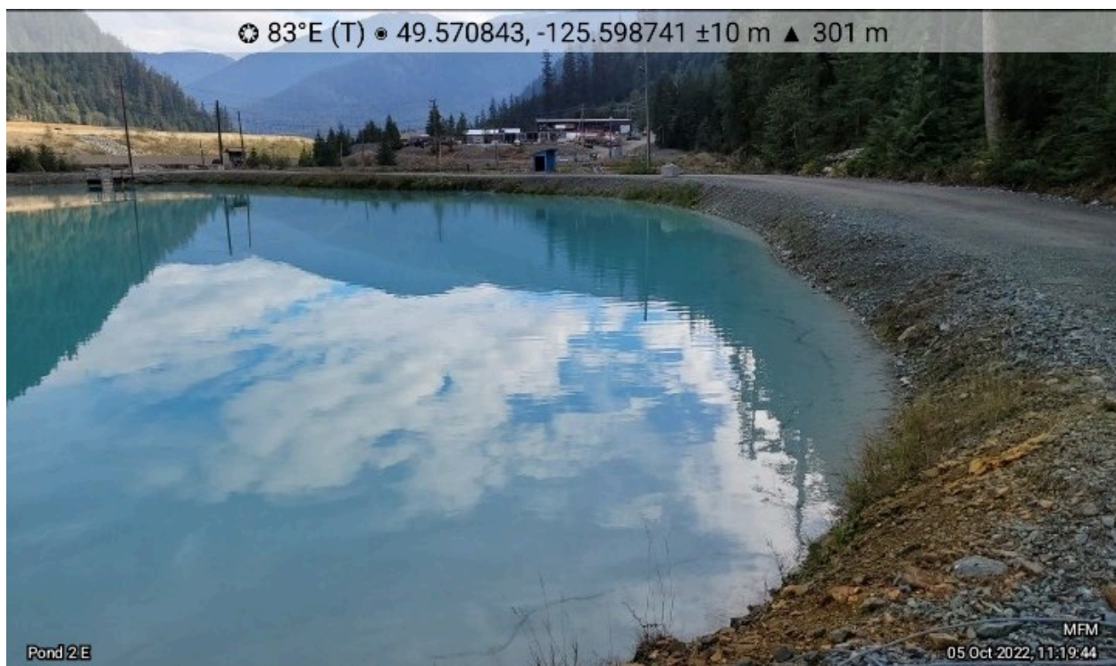
Photo 29: Polishing Pond 2 looking East. No unusual performance was observed.
