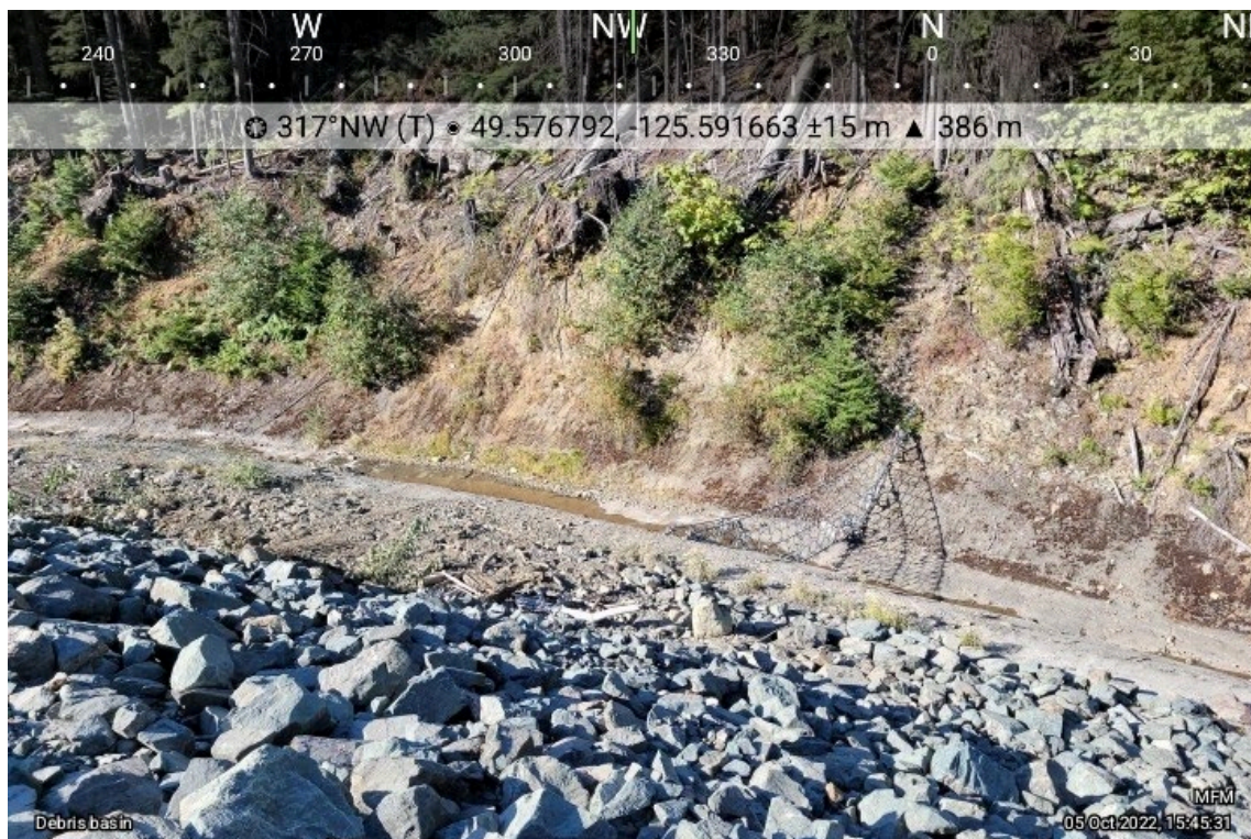
Photo 22: West end of the Lower Lynx Diversion Ditch at the location of the interim debris retaining net
