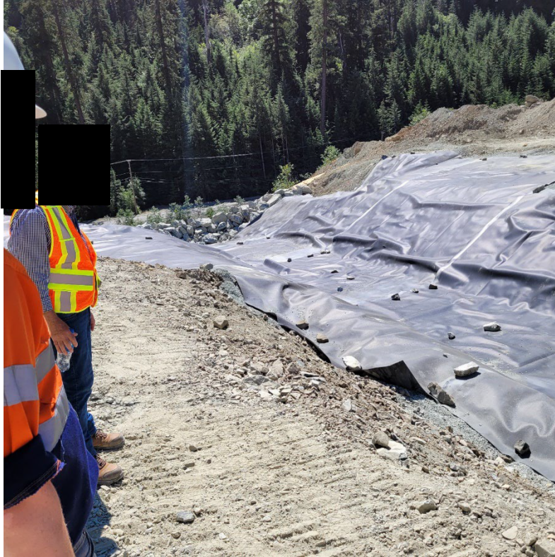
Photo 7: Liner system of the Old TDF spillway
