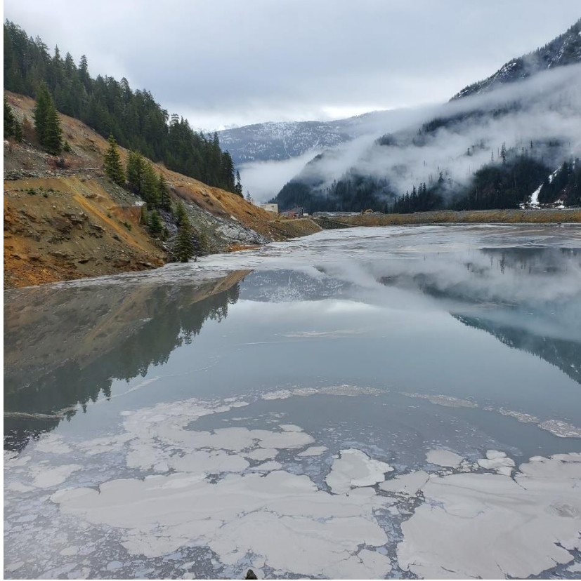
Photo 5: Lynx TDF, looking east with tailings pond covering about 2/3 rd of the tailings surface. (March 22, 2022)
