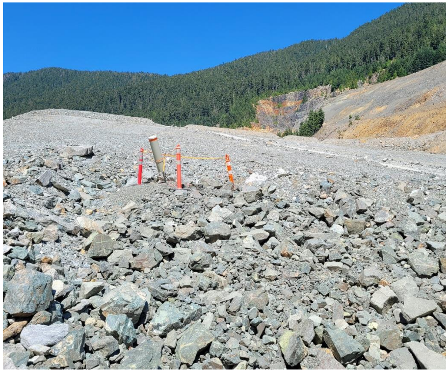
Photo 11: Lynx TDF 4H:1V sloped Downstream East side portion of dam. Shown also is RSTAR data logger DT2055-6. (July 26, 2022)
