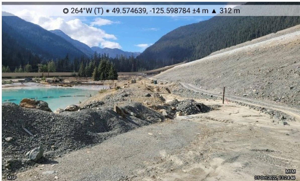
Photo 20: Super Pond looking upstream to the top of the pond and the berm that separates Super Pond from the downstream toe of Lynx TDF. No unusual performance was observed.
