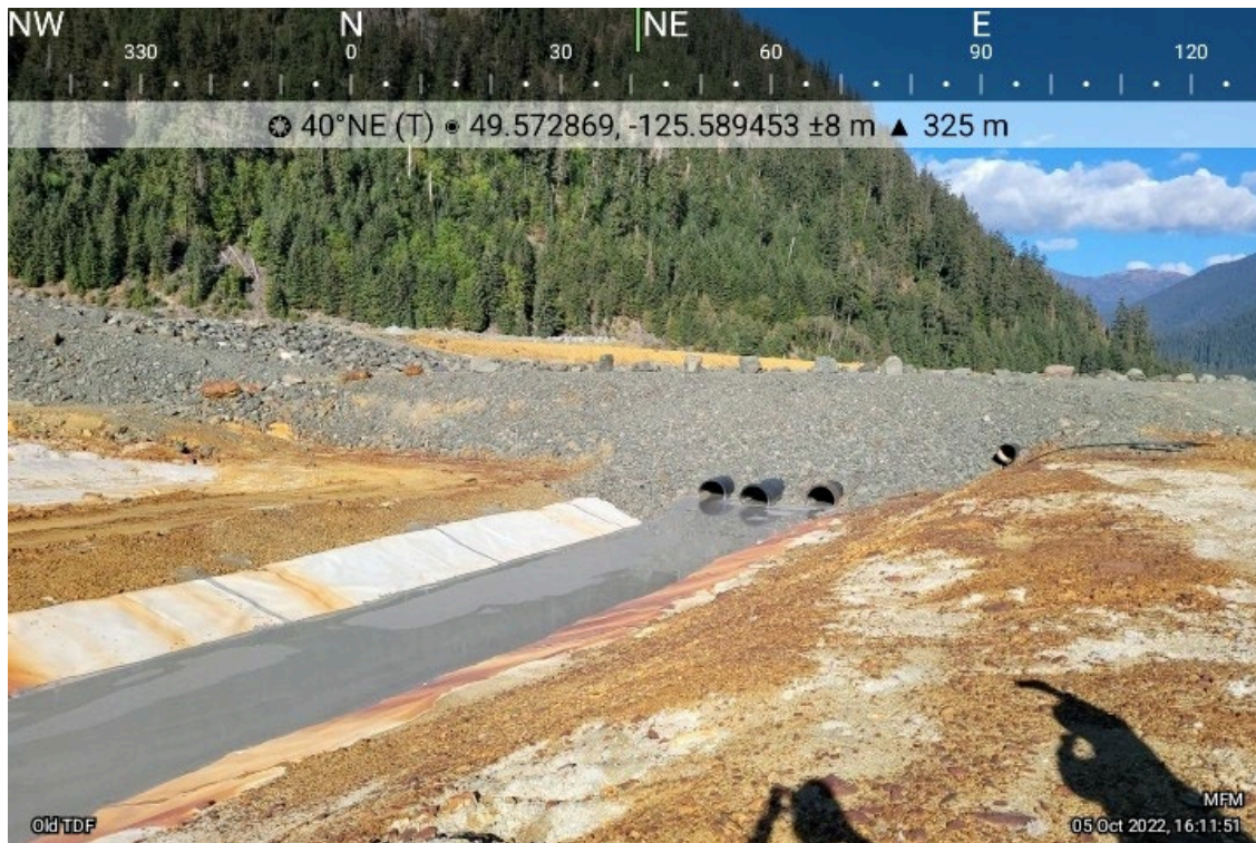
Photo 13: The West Strip of the Old TDF was filled with tailings obstructing the flow capacity of the spillway culvert pipes. This condition needs immediate attention before the wintertime.
