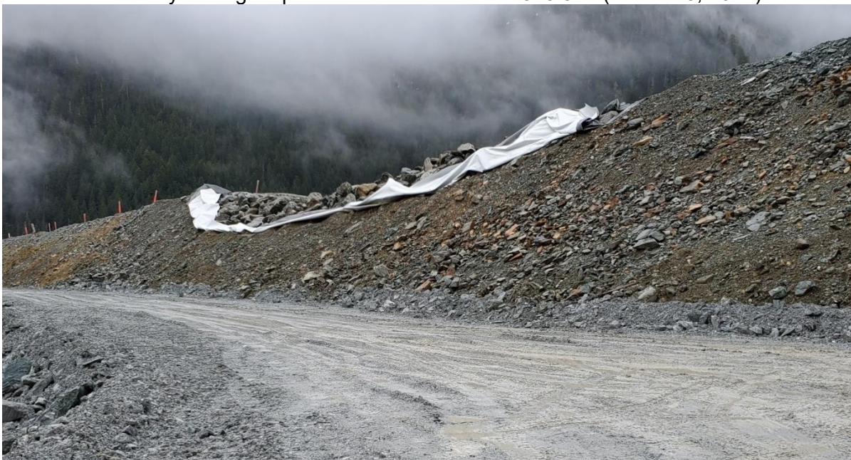
Photo 8: Lynx TDF dam crest (looking north-west). Shown is the uncompleted portion of the spillway invert which needs to be extended across the upstream bench -photo taken standing upstream bench. (March 25, 2022)
