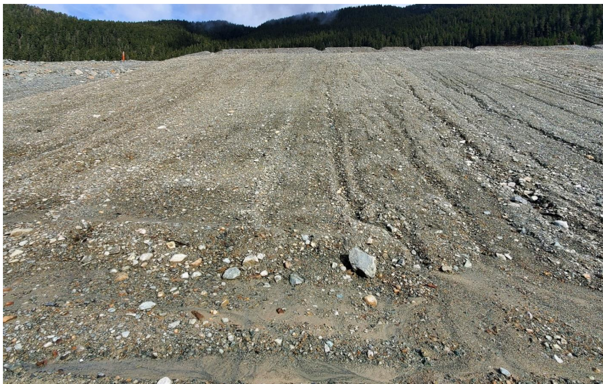
Photo 5: Lynx TDF downstream toe which was used for Closure Cover Trials in 2021. Erosion gullies observed in the clean cover for this area. (March 25, 2022)
