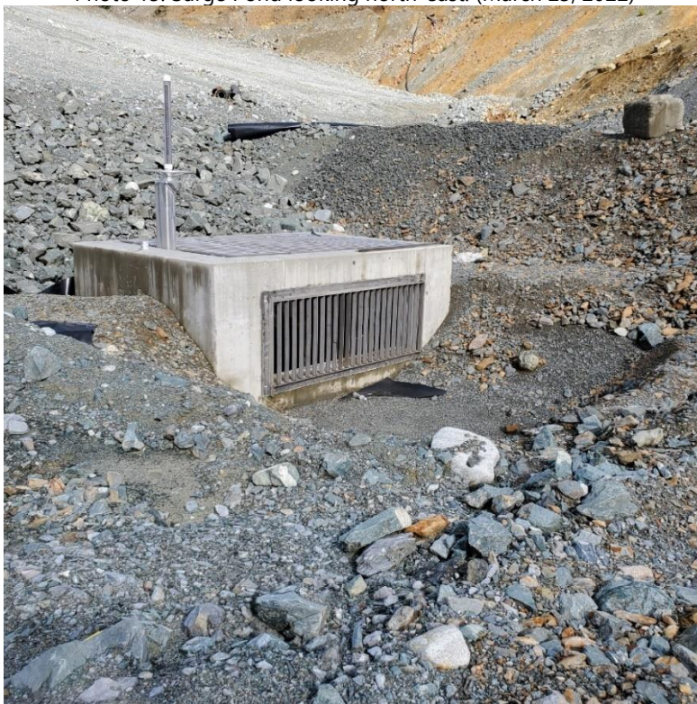
Photo 16: Temporary Lynx Spring Drain Sump. Functioning as intended with discharge observed to be clear. (March 23, 2022)
