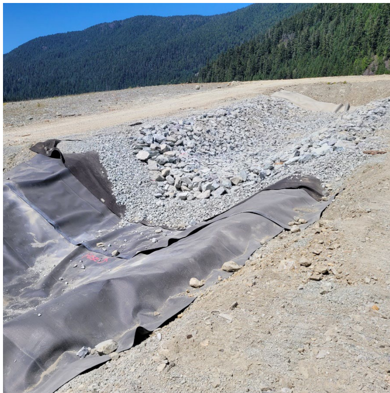
Photo 6: Geomembrane and geotextile liner along the spillway of Old TDF
