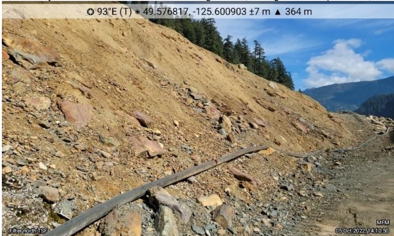
Photo 18: Lynx TDF East Abutment at WRD1, looking southeast. Pipe shown carries tailings from Paste Plant. (October 5, 2022)
