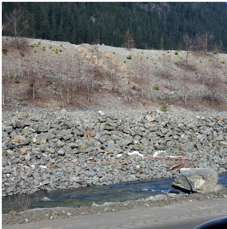
Photo 34: Gully erosion observed on downstream end of Seismic Upgrade Berm of the Old TDF, gully erosion to be addressed during Phase 1 Closure of Old TDF in 2022 construction season (March 23, 2022)
