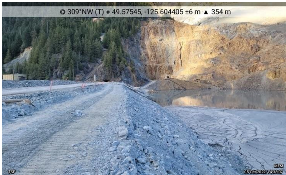
Photo 13: Lynx TDF looking northwest. Crest elevation is at 373.5 m. Photo taken from Upstream bench which was under construction to be raised to 373.5m. (October 5, 2022)
