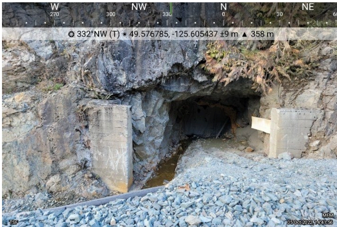
Photo 8: Lynx TDF West Abutment showing 10 Level East Portal, looking north. Ongoing drainage flows from the portal. The portal is to be plugged and sealed before next dam raise construction.
