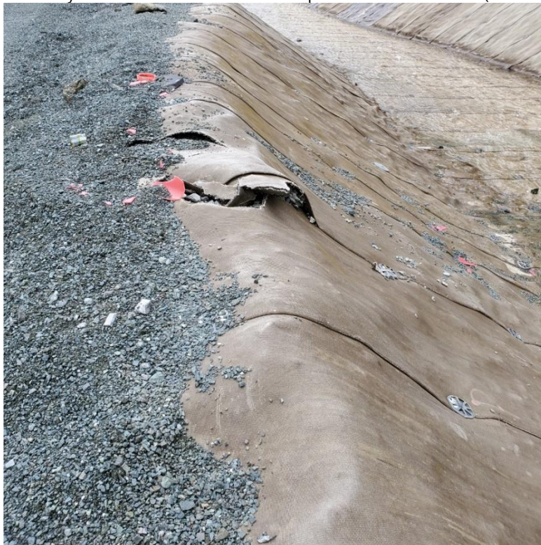
Photo 10: Lower Lynx Diversion Ditch damage to concrete cloth observed. (March 22, 2022)
