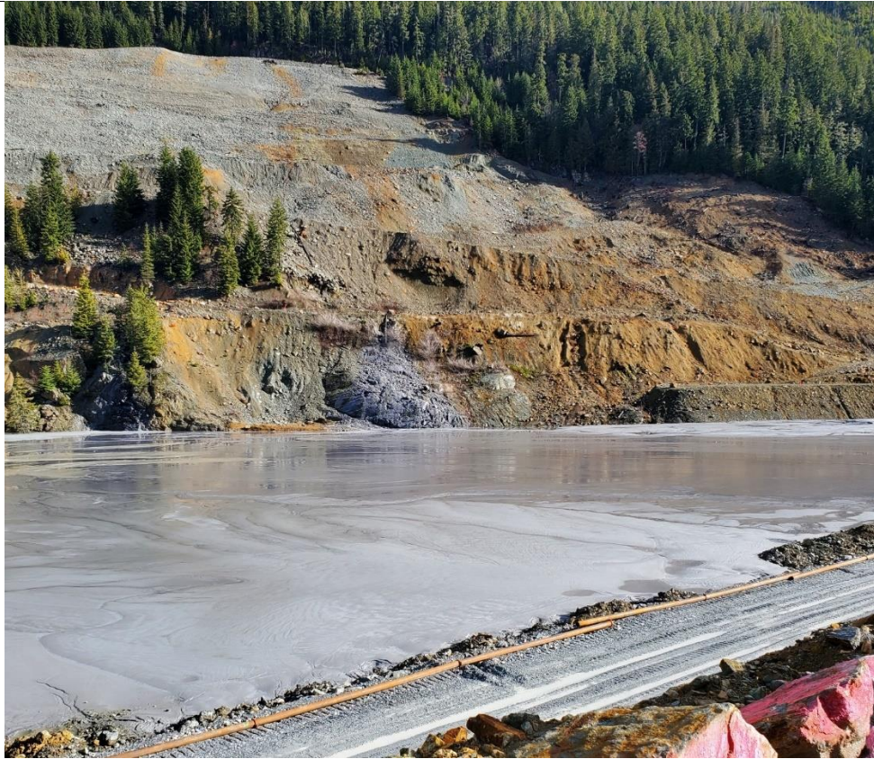
Photo 7: Lynx TDF, looking north-east. Standing on the crest. It can be observed that the upstream bench has not yet caught up to the crest elevation of 373.5m. (March 25, 2022)
