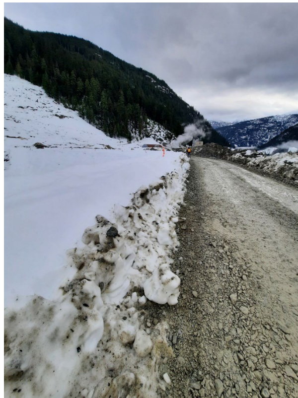
Photo 3e: Lynx TDF dam crest showing well maintained running surface with minimal pooling
