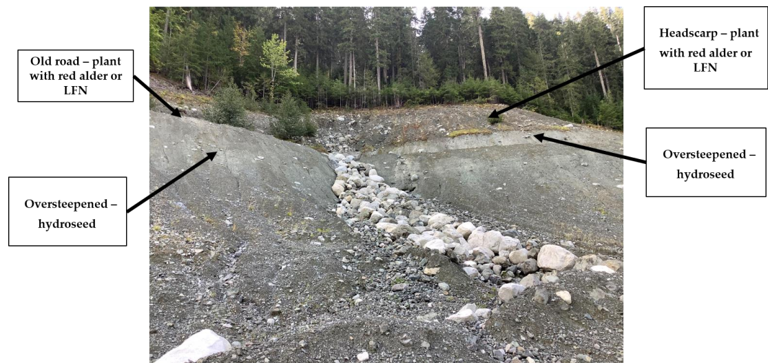
Figure 7. Core Rack Area Borrow. Options for reclamation in this area include hydroseeding oversteepened areas with an aggressive native seed mix, followed by planting the headscarp and old road areas with red alder or leaving for natural revegetation (LFN). Photo date: September 2019.
