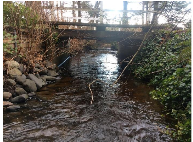
Photo 1 & 2. Views upstream of Reach 1 at km 0+122 (above left; Feb. 11, 2020) showing concrete retaining wall, historical counting fence structure (right of image), and riparian removal on right bank (left of image); and view downstream (above right; Feb. 11, 2020) showing riparian disturbances from driveway bridge installation, rock revetment (left bank) and English ivy encroachment (right bank).
