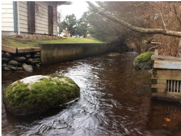
Photo 1 & 2. Views upstream of Reach 1 at km 0+122 (above left; Feb. 11, 2020) showing concrete retaining wall, historical counting fence structure (right of image), and riparian removal on right bank (left of image); and view downstream (above right; Feb. 11, 2020) showing riparian disturbances from driveway bridge installation, rock revetment (left bank) and English ivy encroachment (right bank).
