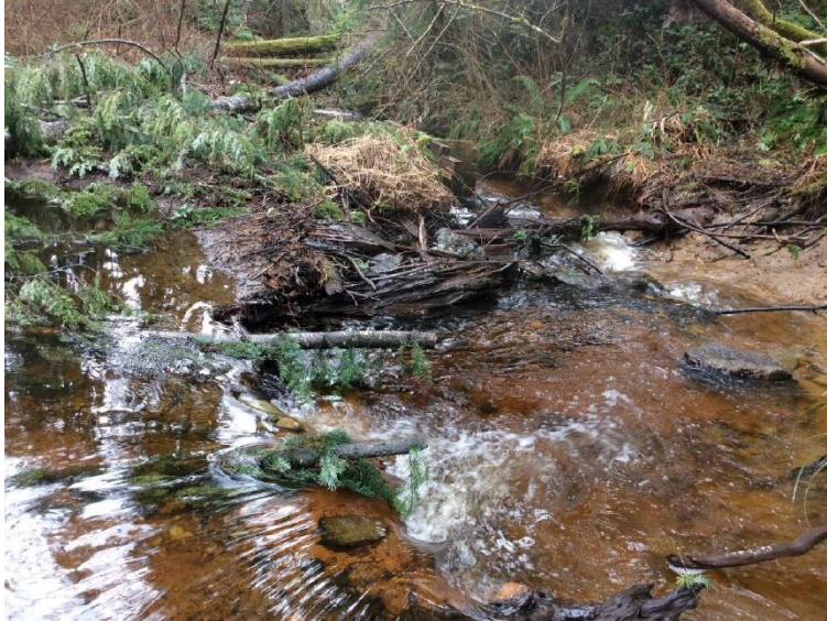
View downstream J- Wood weir 1999 avulsion on right bank (background) and control level provided by hardpan (foreground).
