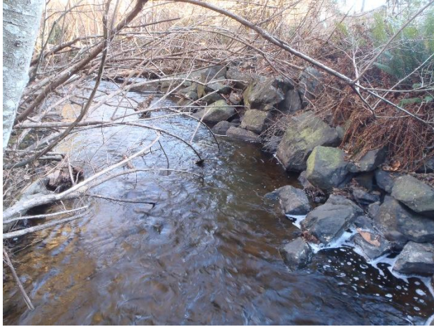
Photo 13. Ad hoc bank revetment structure composed of angular rock present near 1+160 km, providing evidence of erosive forces combined with anthropogenic bank modifications including native riparian vegetation removal affecting this section of Reach 2.
