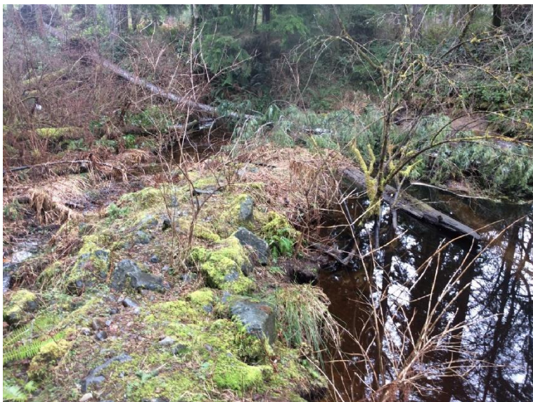
Rock berm on left bank (foreground) used to tie in original wood weir (hidden under fallen tree; background) remains intact and can be used to tie in a new rock weir/riffle K - Rock Weir structure to replace failed wooden weir.
