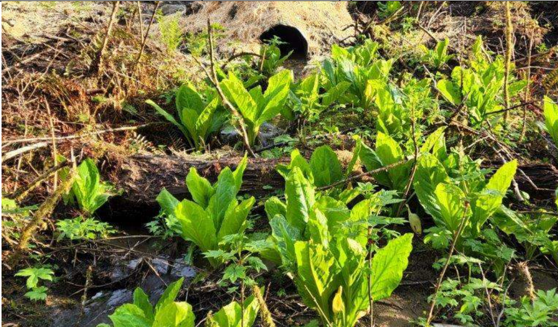
Plate 7. Logging road crossing using a corrugated steel pipe. Note ESC measures (straw and coastal reclamation seed mix) Stream 1 – Reach 1. (April 2022)
