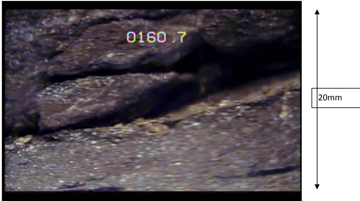
Photo 5.5: DH Qu10-17 48m depth. Dilated aquiclude zone. Open bedding plane fractures.
