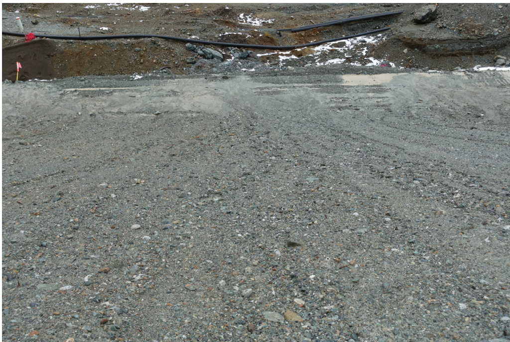
Figure 6. Erosion fans (background) at the toe of the Lynx TDF closure cover trial.
