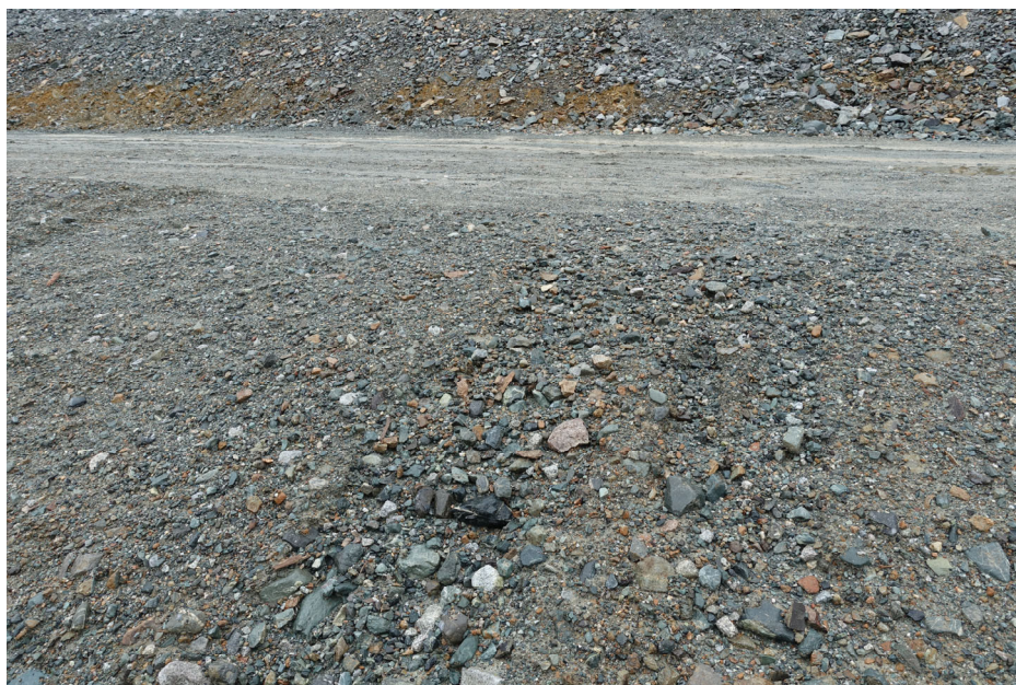
Figure 8. Erosion initiating at the top of the Lynx TDF closure cover slope, likely caused in part by run-on water flowing off the bench and on to the slope crest.
