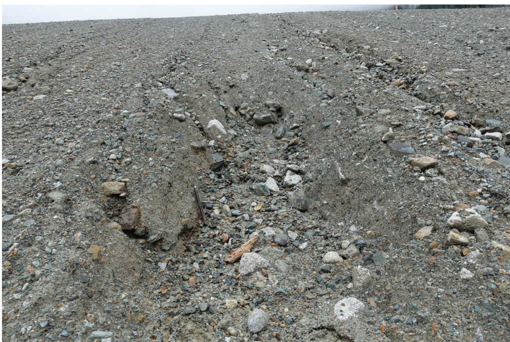
Figure 7. Erosion hole in cover, 40-cm deep (20-cm multi-tool for scale).
