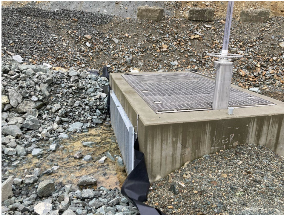
Photo 9: Lynx TDF Springs Drain Sump box culvert, clear inflow (November 17, 2021)
