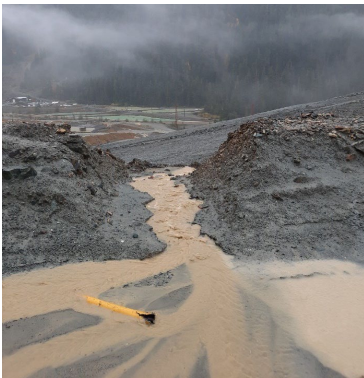
Photo 7: Lynx TDF punch-out in dam crest berm during precipitation event. (October 27, 2021)
