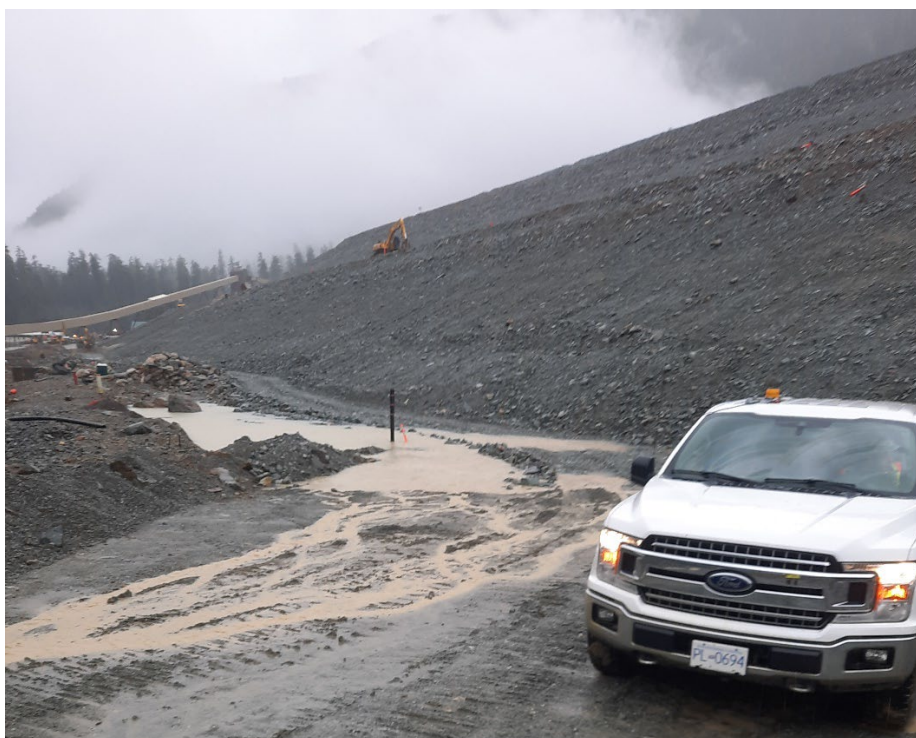
Photo 8: Lynx TDF – Water ponding around standpipe near the Panel 15 drain (October 21, 2021)
