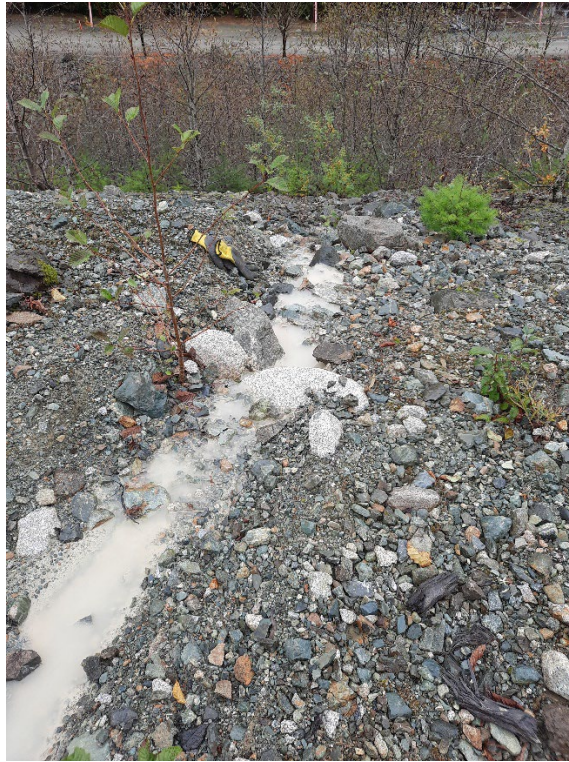
Photo 19: Old TDF Seismic Upgrade Berm – location of erosion, view looking south. (October 27, 2021)
