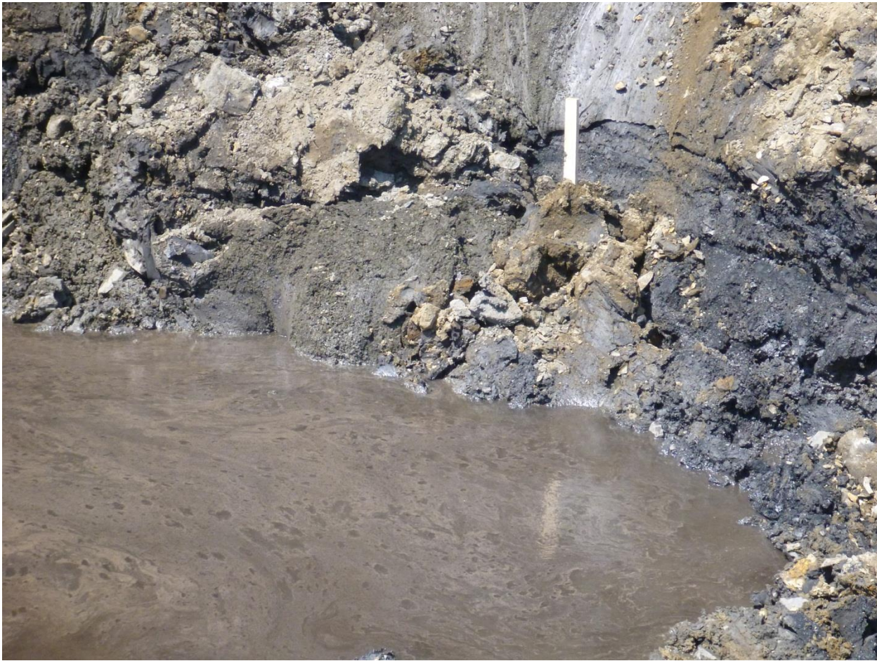
Figure 5 – Spill site after removal of fuel and the majority of contaminated soil. The wooden stake represents the approximate spot of the original drum. The water in the photo is ground water that has been exposed while digging out the contaminated soil. The film on the water appears to be coal dust.
