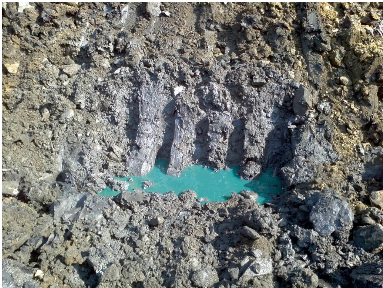
Figure 2 – Diesel fuel immediately after the drum was punctured by the excavator
