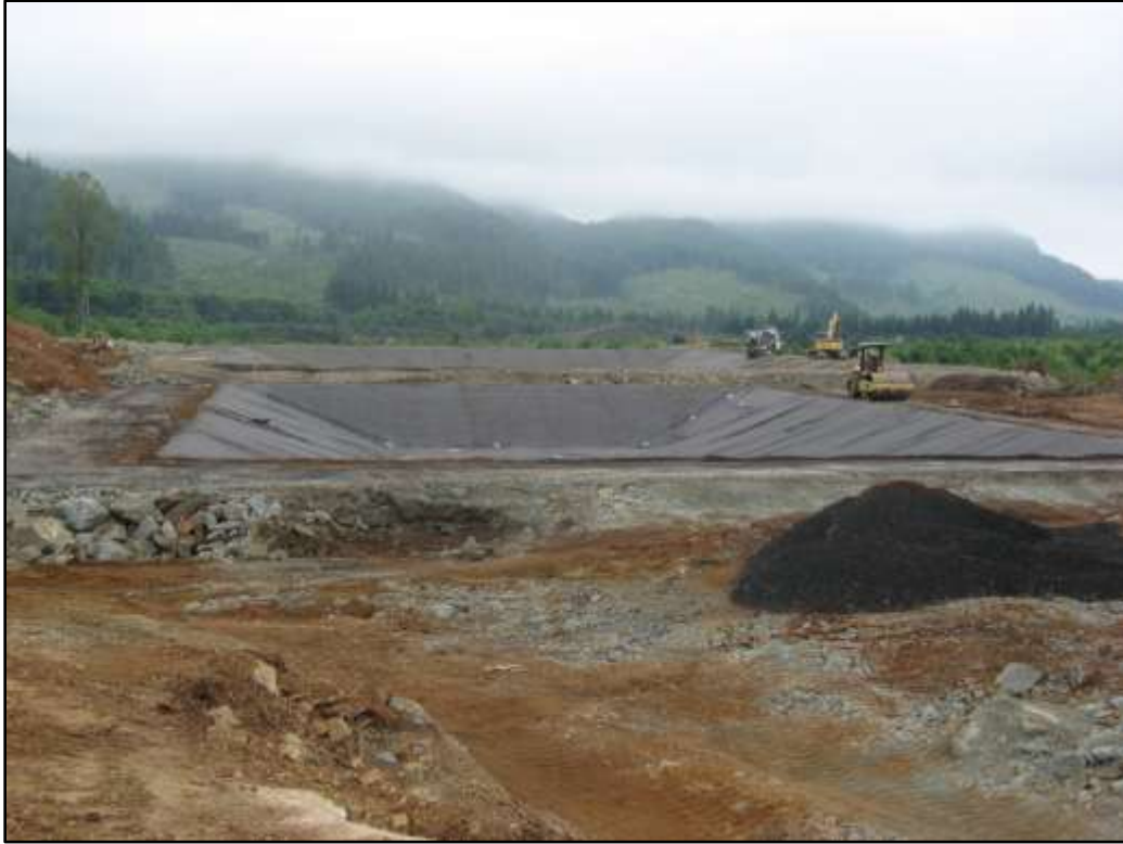
Photograph 9: Lined (geomembrane with a geotextile underlay and overlay) Sulphide Polish Cell (with the BCR Cell in the background)
