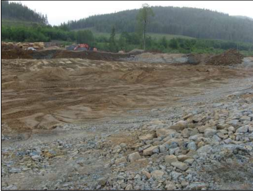
Photograph 7: Cut-and-Fill Construction for the BCR Cell
