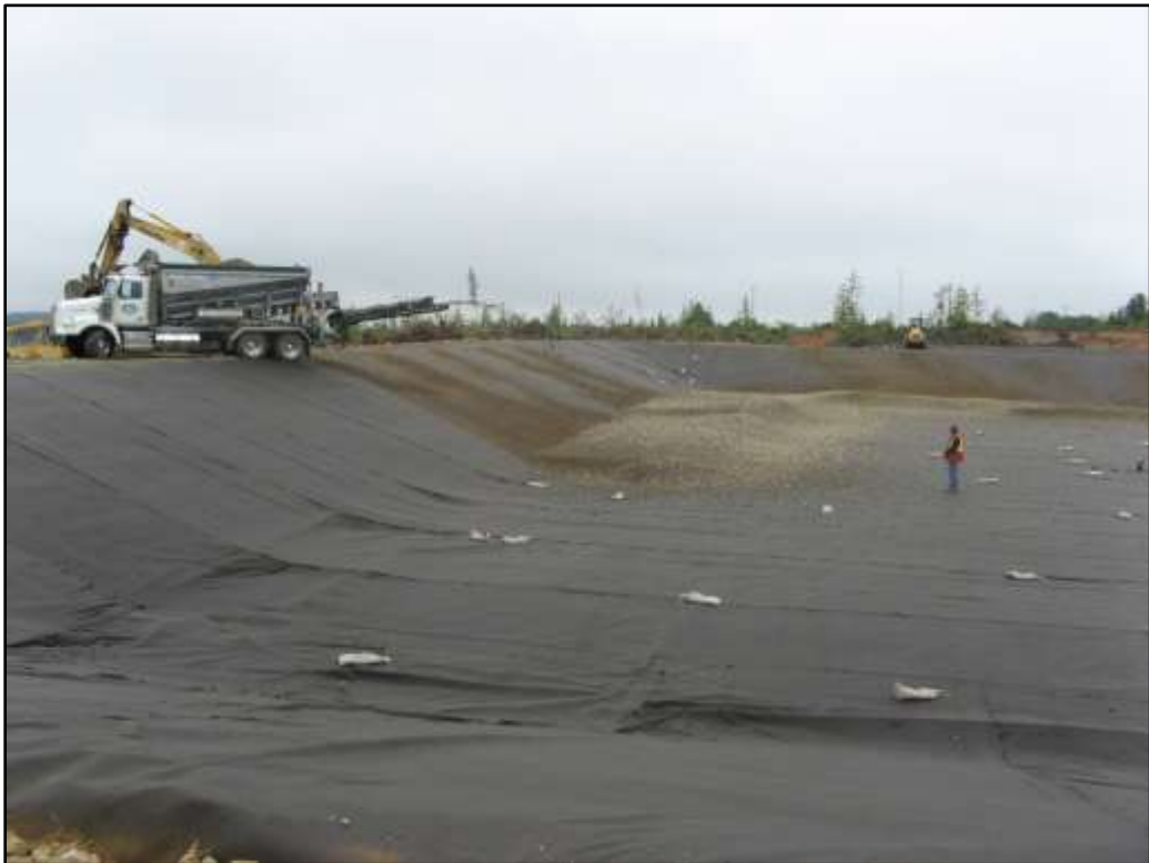
Photograph 10: Placing the Drain Rock into the BCR Cell
