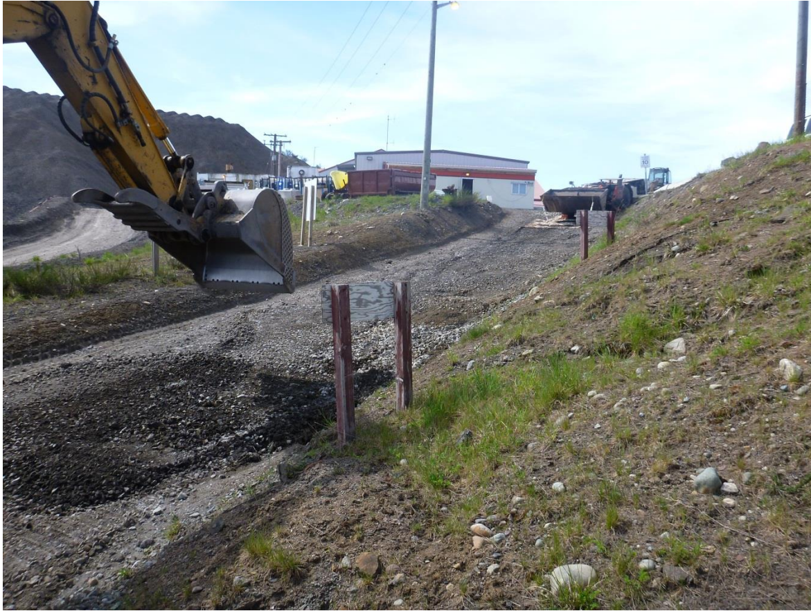
Plate 3. – After removing the oil-soaked absorbent pads into plastic spill drums, final cleanup involves an excavator to scrape and load contaminated soil into a truck which deposits the soil onto a plastic liner, for sampling and possible treatment, or removal to an approved contaminated waste disposal facility.
