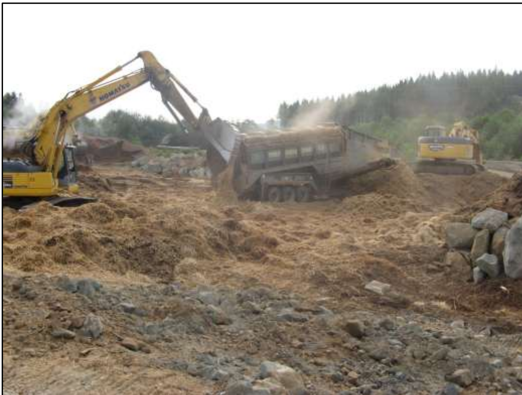
Photograph 12: Mixing Substrate (wood chips, hay and limestone) for the BCR Cell
