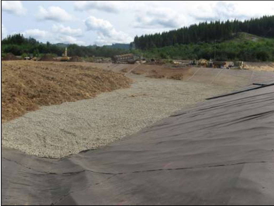
Photograph 13: Placing Substrate into the BCR Cell
