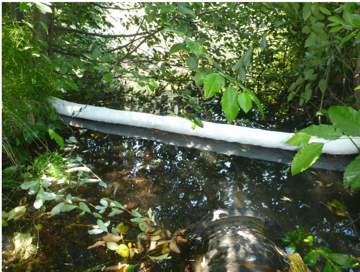
Figure 6 – Absorbent boom placed across the drainage ditch that leads from the 2 South Sump water collection to the 3 South Pit to prevent contaminants from moving further through the water system.
