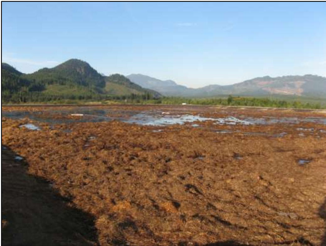
Photograph 14: BCR Fill filled with Substrate and Initial Charge of Water for Commissioning
