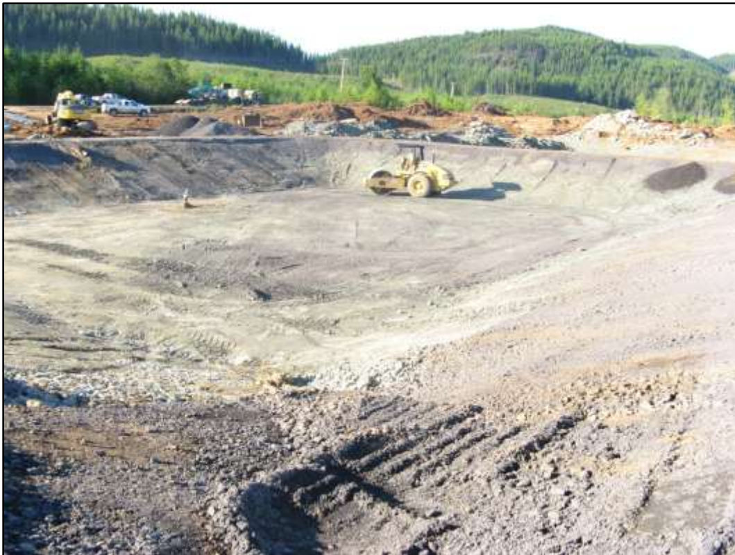
Photograph 4: Excavation (primarily in drilled and blasted rock) for the Settling Pond
