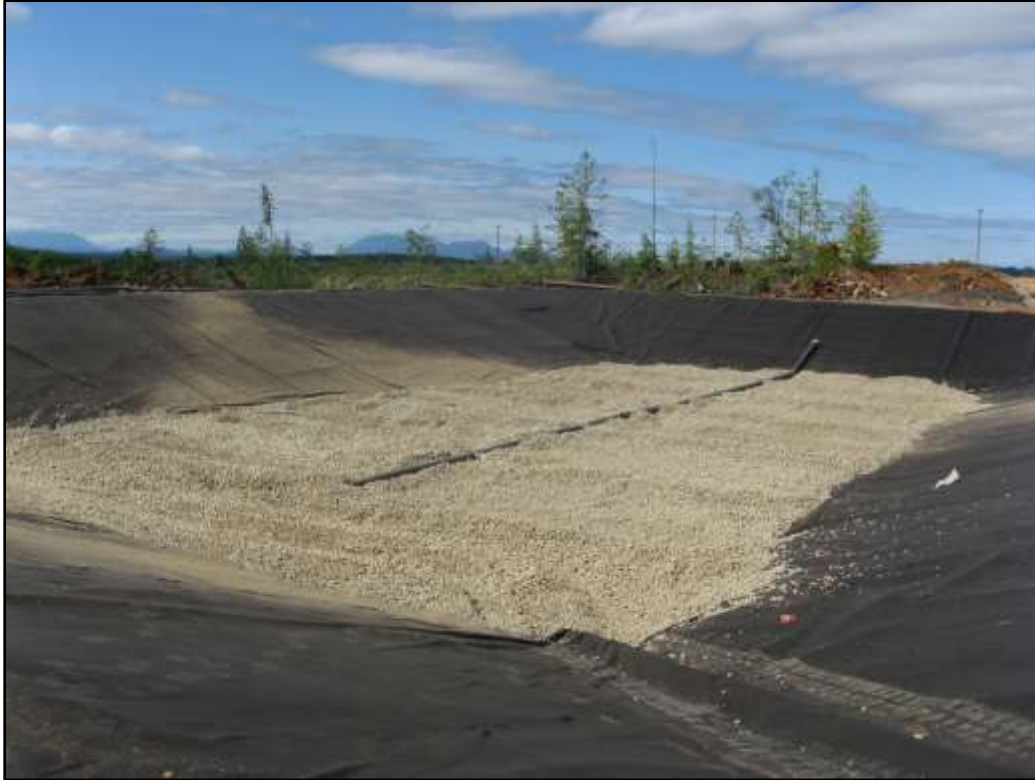
Photograph 11: Drain Gravel and Lower Piping in the Sulphide Polish Cell
