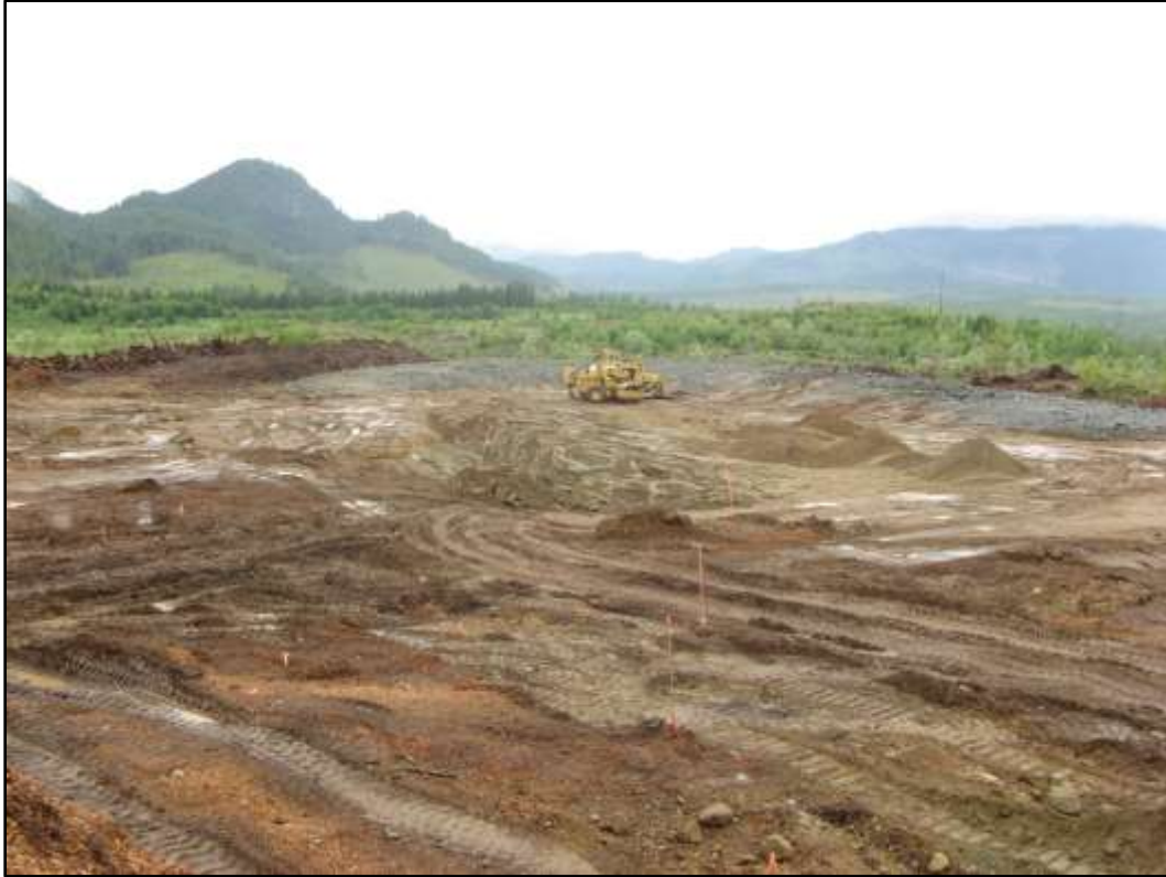
Photograph 3: Coversoil Salvage and Initial Excavation of the BCR Cell
