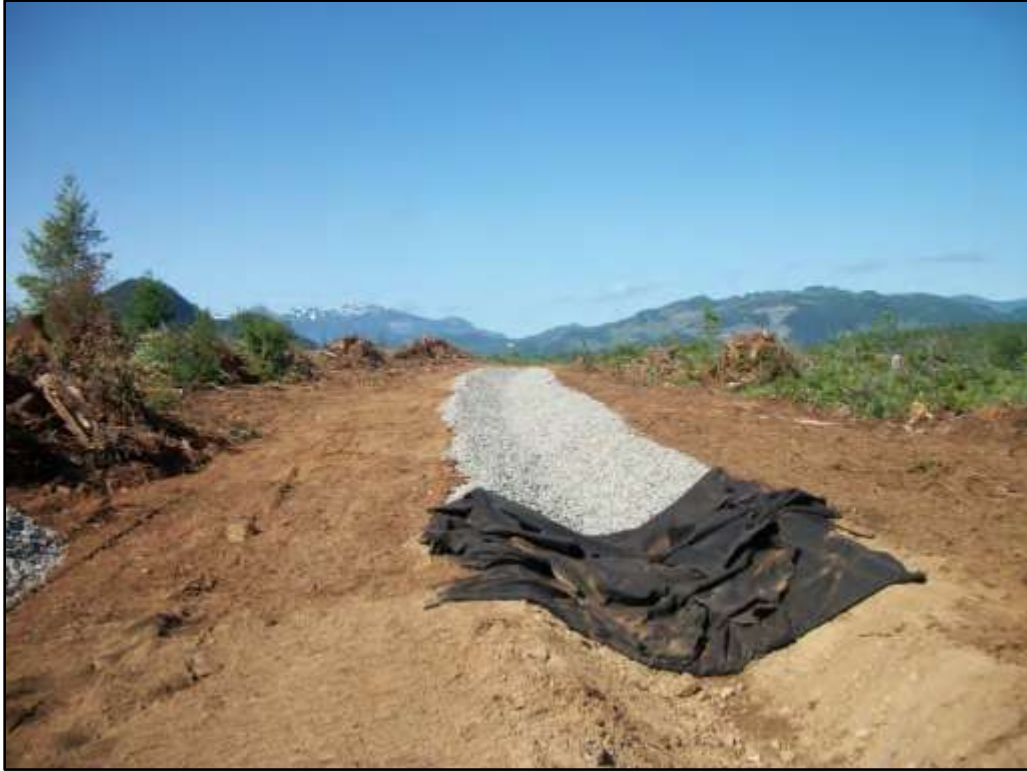
Photograph 17: Settling Pond Effluent Channel Construction
