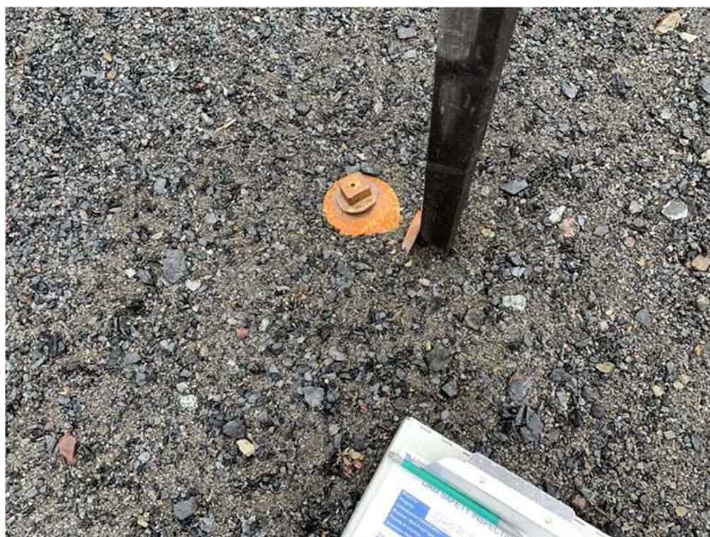
Photo 26: 2-North Pit TDF, Example of Survey Monument on dm crest.
