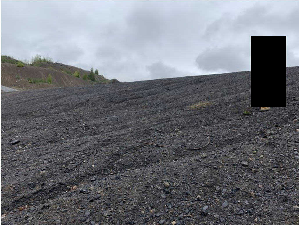
Photo 5: Old TDF, South Dam Downstream Slope with Erosion Rills Across Surface, Looking West.
