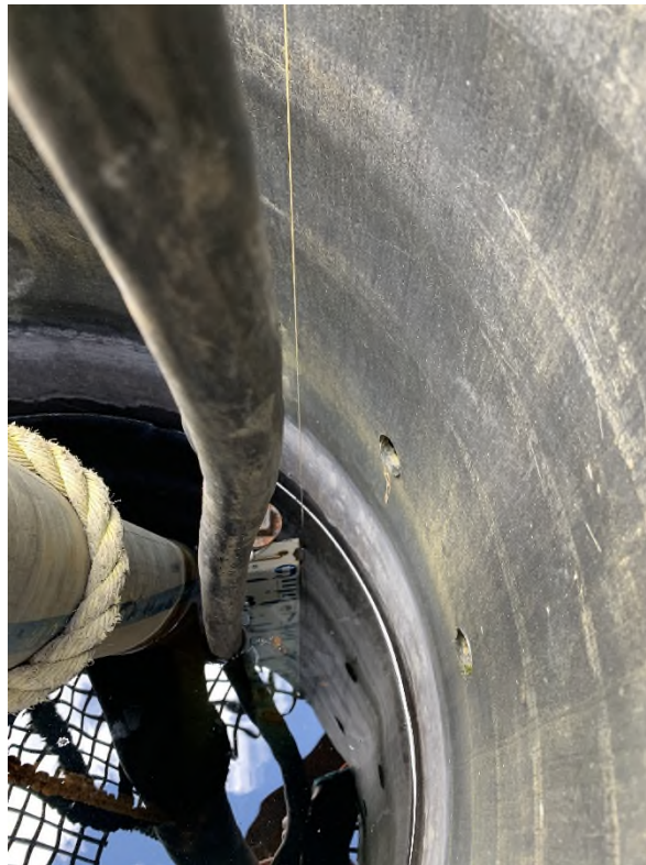
Photo 12: 2 South Pit Pond, Staff Gauge Installed in Vertical Culvert in Internal Dividing Dyke
