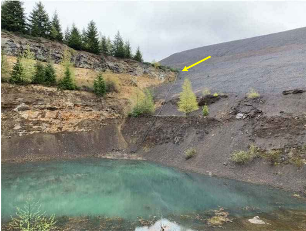
Photo 3: 2-North Pit TDF, North Embankment Downstream Toe and Abutment, Siphon Pipe From Northeast Corner of TDF identified by yellow arrow, Looking East.
