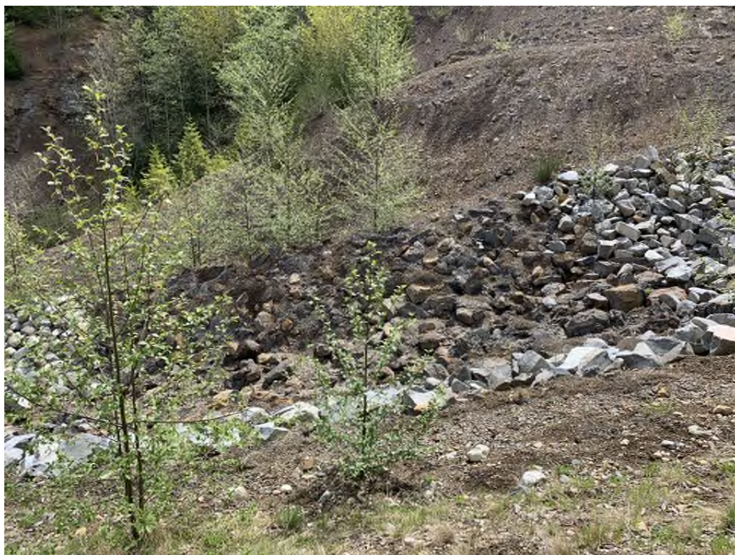
Photo 18: 2 South Pit Armoured Outlet Channel to 3 South Pit, Riprap is Weathered, Looking North
