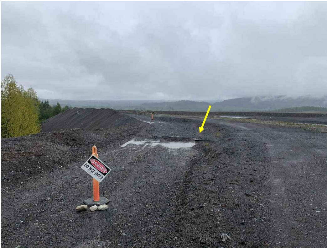
Photo 15: 2-North Pit TDF, Ponded Water on East Embankment Crest Drained by Pipe into TDF, Looking Southeast. Pipe identified by yellow arrow.
