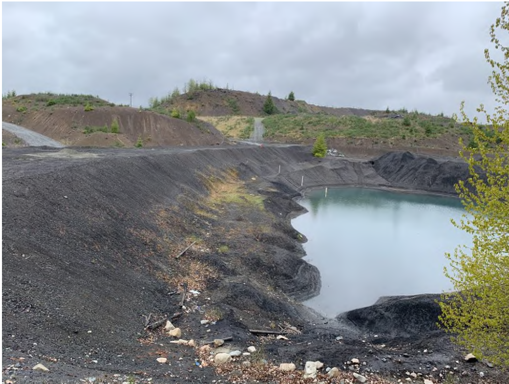
Photo 3: Old TDF, South Dam Upstream Slope, Slope Surface is Irregular, Looking West.
