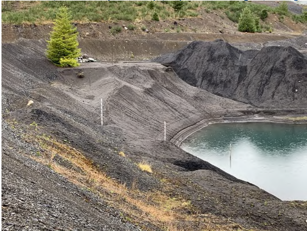
Photo 4: Old TDF, South Dam Upstream Slope, Showing the Three Staff Gauges and Tree on the West Abutment, Looking West.
