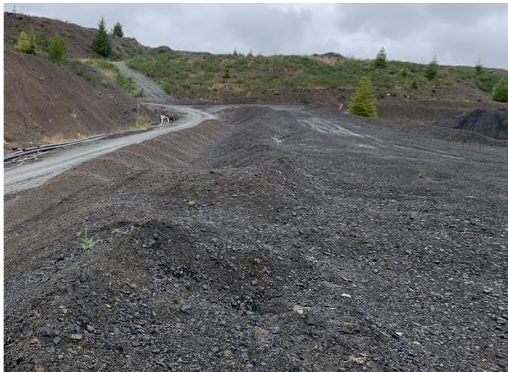
Photo 8: Old TDF, West Abutment of South Dam, has Water Ponding and Vehicle Ruts Along Surface, Looking North.
