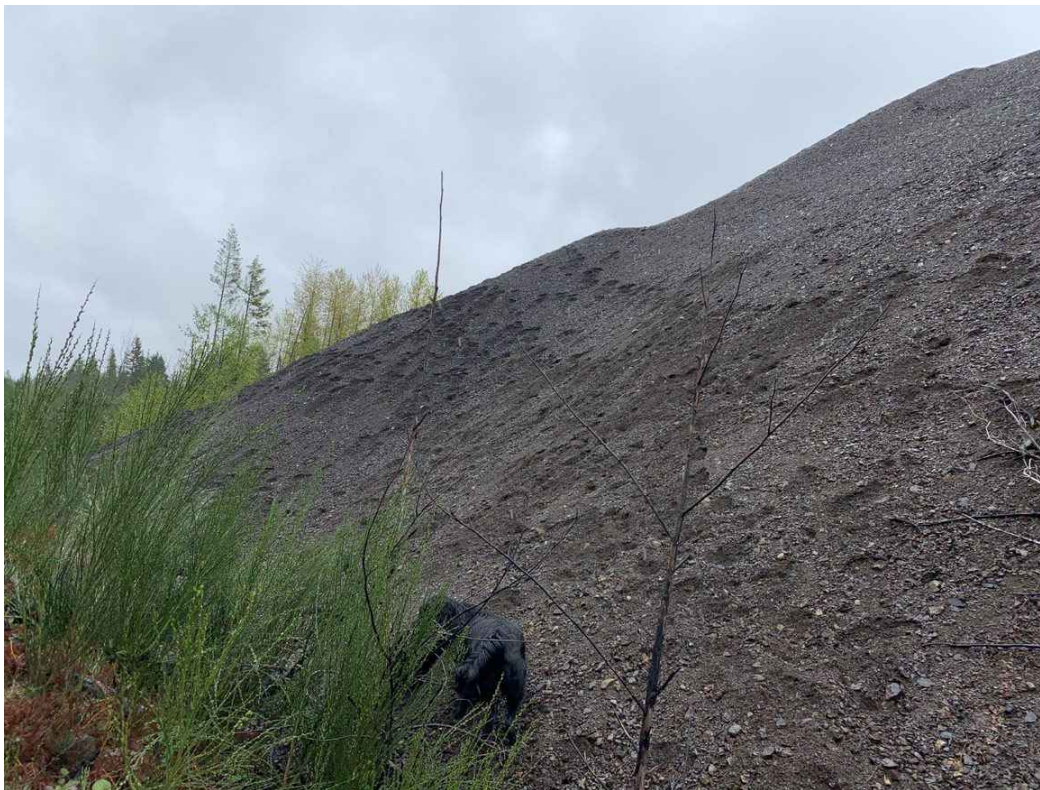
Photo 13: 2-North Pit TDF, East Embankment Downstream Slope With Animal Tracks, Looking Southeast.
