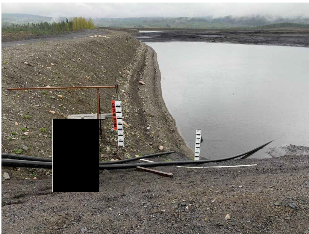
Photo 10: 2-North Pit TDF, East Embankment Upstream Slope and Freeboard Gauges, Looking South.
