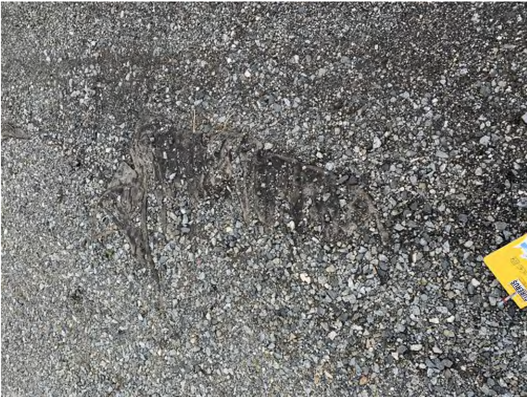
Photo 36: Settling Pond 4 Exposed Geotextile on crest, from 2004 Low Level Outlet Repairs.
