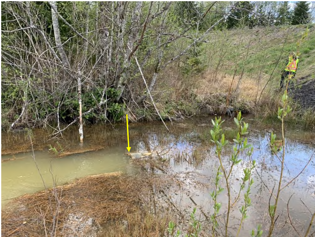
Photo 35: Settling Pond 4 Submerged Downstream Outlet, identified by yellow arrow.
