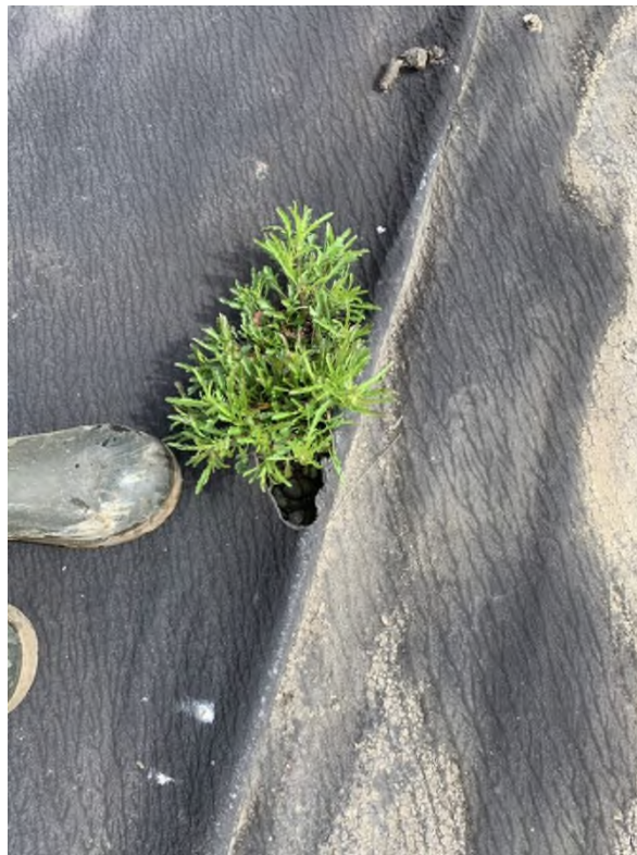
Photo 15: 2 South Pit Outlet Spillway, Small Tears in the Geomembrane.
