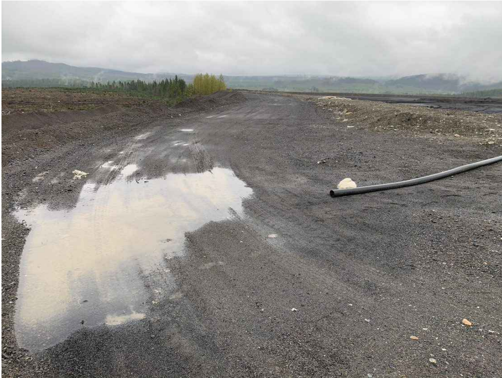
Photo 11: 2-North Pit TDF, East Embankment Crest with Pondered Water, Looking South.
