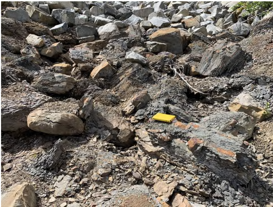
Photo 19: Close Up of Weathered Riprap in Channel between 2 South Pit and 3 South Pit.
