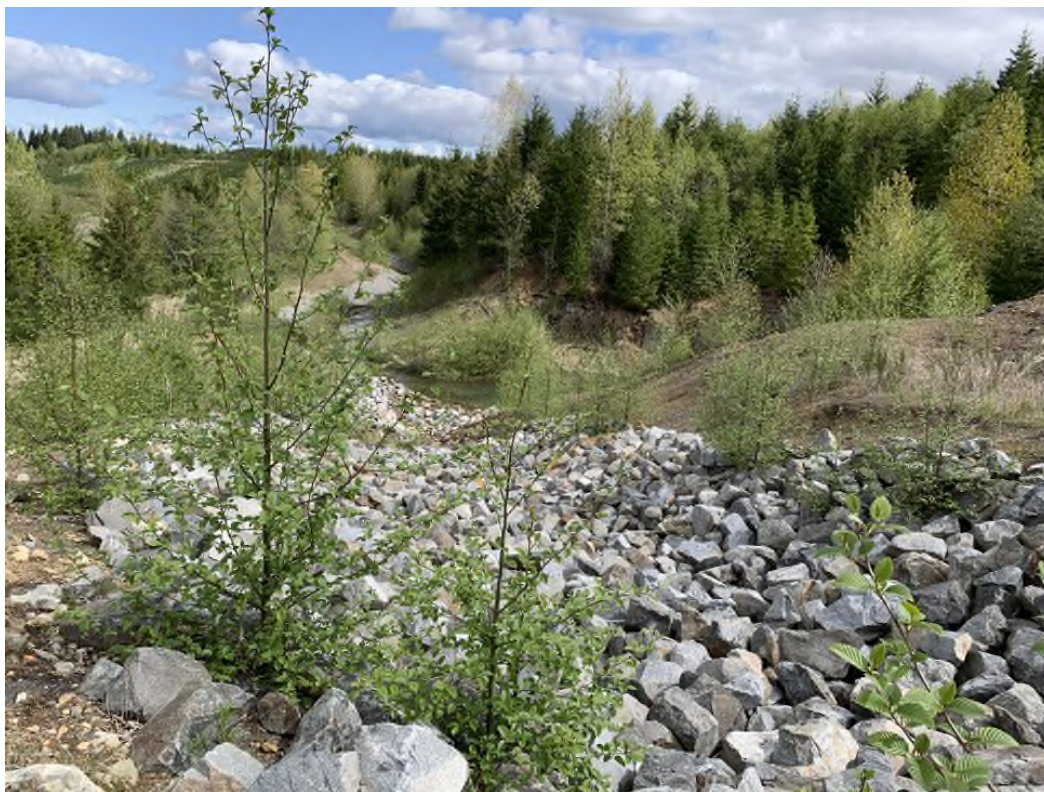
Photo 17: 2 South Pit Armored Outlet Channel, Looking Downstream.
