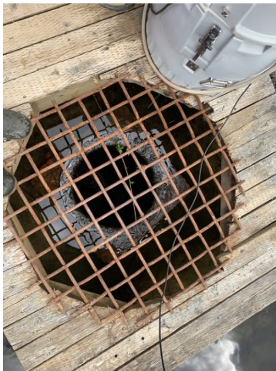
Photo 5: Settling Pond 1 Upstream Decant, Fencing is to Prevent Beavers Blocking Decant, Facing Northeast.
