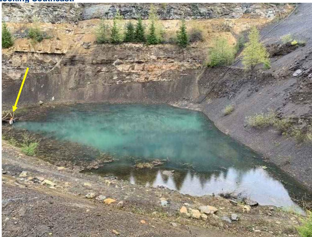
Photo 2: 2-North Pit TDF, Ponded Seepage at the Toe of the North Embankment Downstream Toe and Pumping Barge identified by yellow arrow, Looking East.
