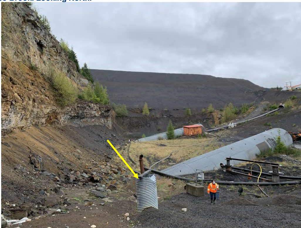
Photo 10: Old TDF South Dam, downstream toe. Corrugated Steel Pipe previous used for sampling identified by yellow arrow. Looking South.
