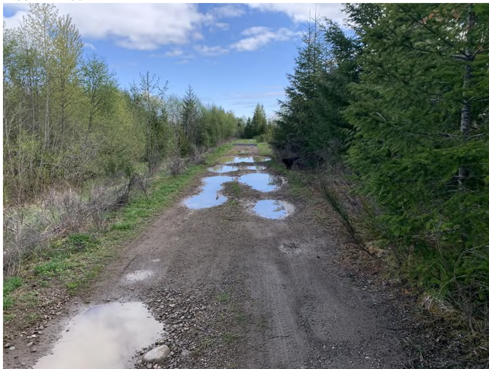
Photo 2: Settling Pond 1 Dam Crest, South End of the Dam with Deep Ruts and Ponding.
