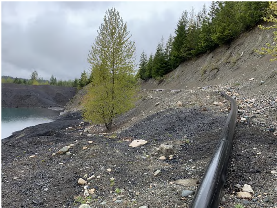
Photo 9: Old TDF, East Abutment of South Dam. Pipe Conveys Water from Underground Mine around Old TDF to Brinco Brook. Looking North.
