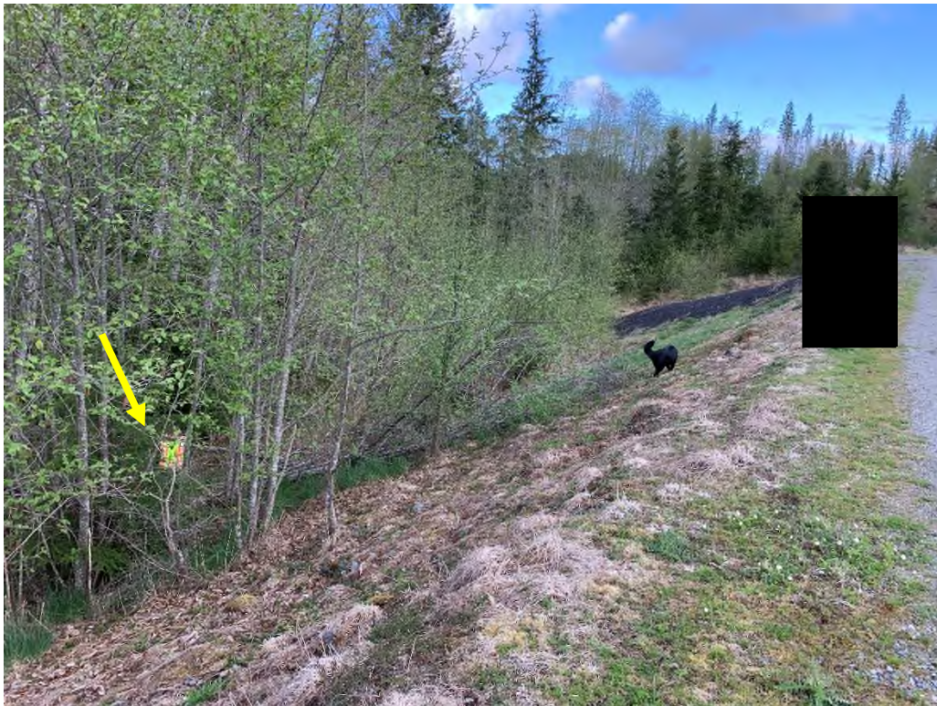
Photo 43: Settling Pond 4 Trees growing on South Side of Downstream Embankment. Dam Toe marked by yellow arrow, all trees upslope should be removed.
