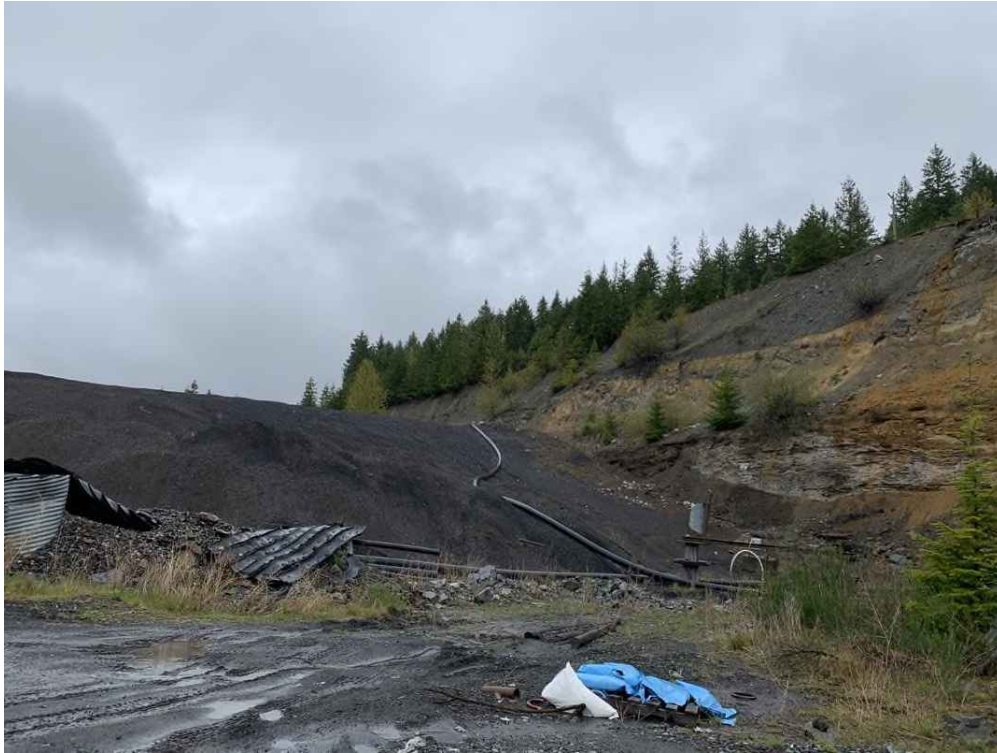
Photo 7: Old TDF, South Dam Toe, Pipe on Dam Conveys Water from Underground Mine around Old TDF to Brinco Brook. Looking North.
