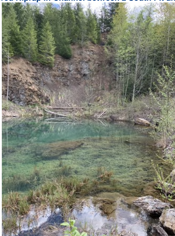
Photo 20: Water Ponded at the Toe of the 2 South Pit Dam in the Channel between 2 South Pit and 3 South Pit.
