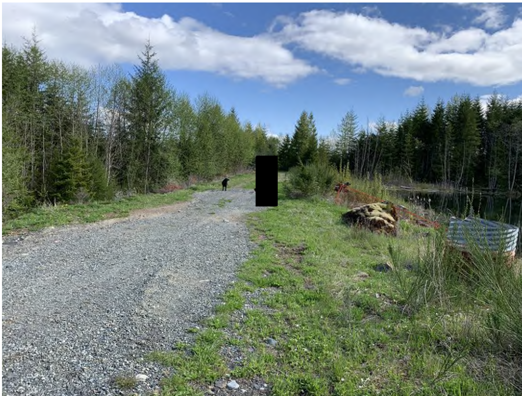
Photo 1: Settling Pond 1 Dam Crest, Small Vegetation Growing on Upstream Slope, Ruts in the Centre of the Dam Have Been Infilled.
