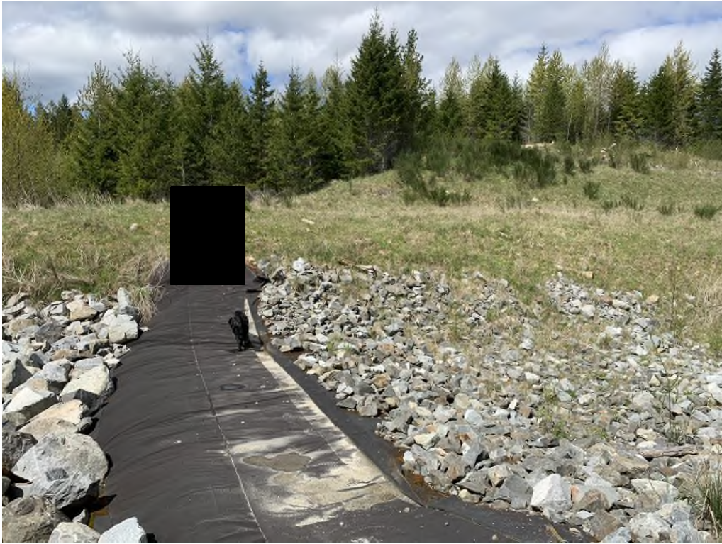
Photo 23: 3 South Pit Pond South Overflow Spillway and Rip Rap Channel, Looking Southwest.
