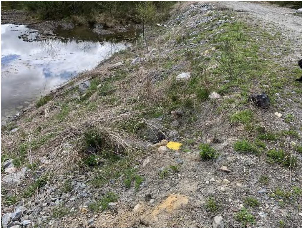
Photo 27: 3 South Pit North Dam, Erosion Runoff Channel on Upstream side of Crest, Looking South.
