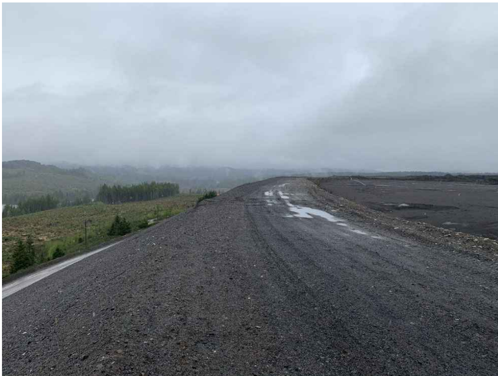
Photo 21: 2-North Pit TDF, Ponding on West Embankment Crest, Looking North.
