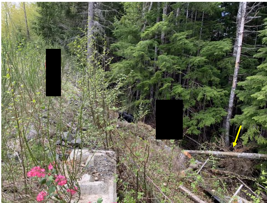
Photo 29: 3 South Pit Pond North Dam Downstream Toe, Lock Blocks Supporting Slope, Trees fallen over and Root Ball Dislodged identified by yellow arrow, Looking West.
