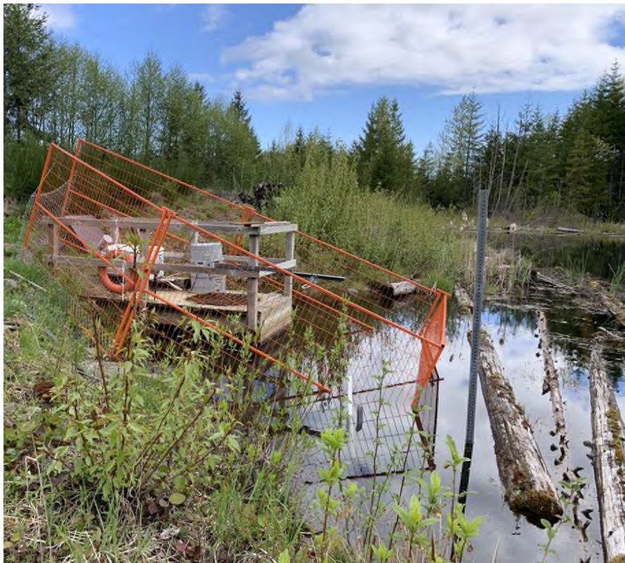
Photo 5: Settling Pond 1 Upstream Decant, Fencing is to Prevent Beavers Blocking Decant, Facing Northeast.
