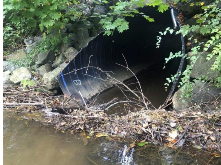
2.) R2 Galerno culvert is easily plugged by Beaver or other debris
