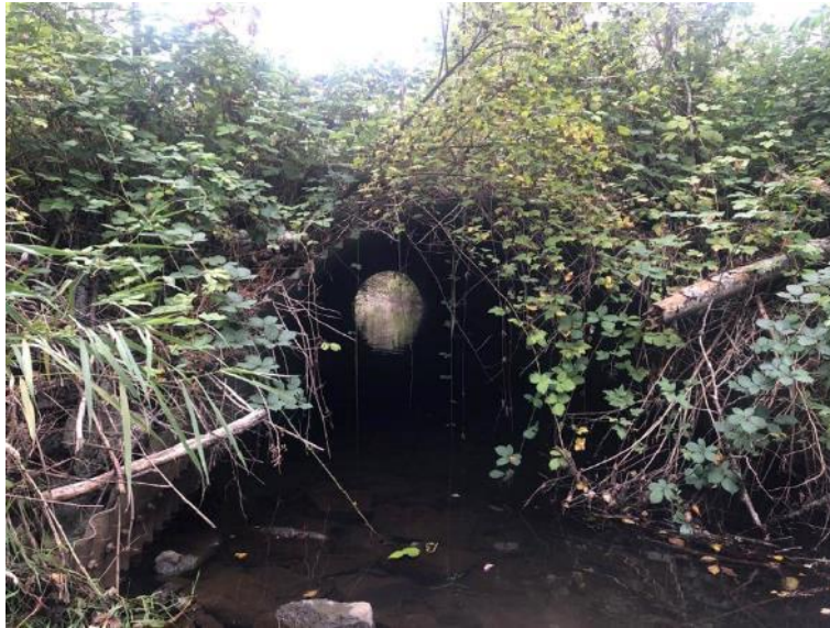
1.) R3 – S. Alder culvert is embedded Arch – passable
