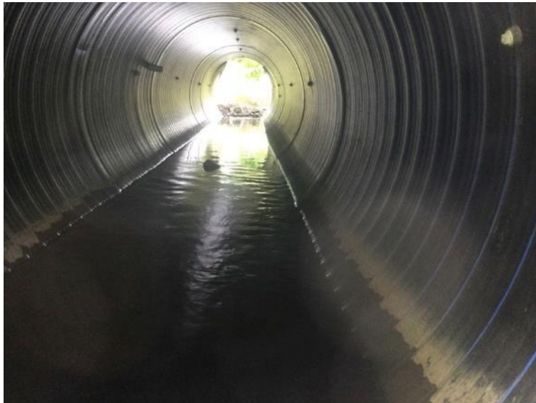
R2 – Culvert lacks embedded depth
