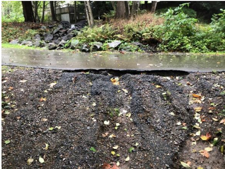
R4 – Stormwater overflow/erosion across trail (Site 82)
