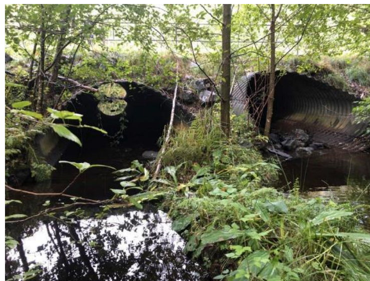
2.) R1 – Twin 3.2m Arch culverts at Rockland Crossing
