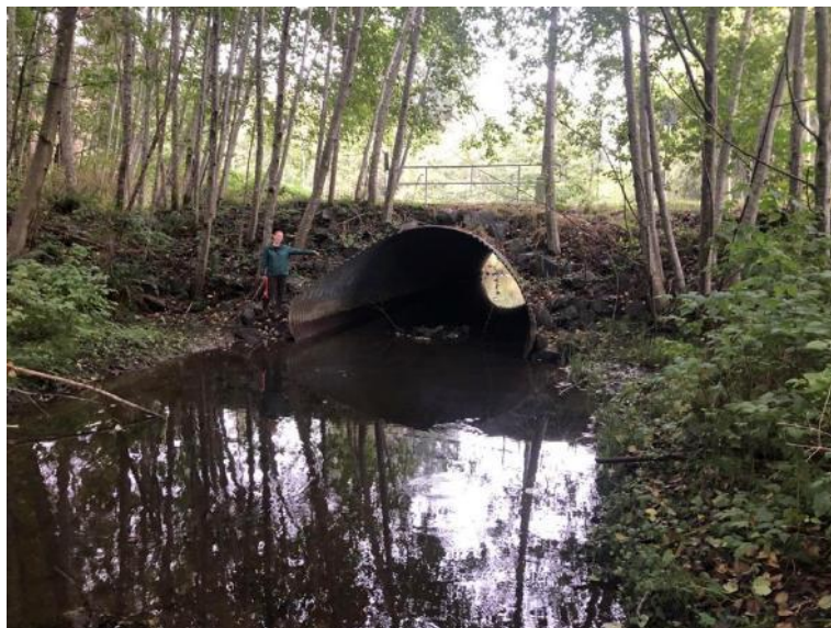
1.) R4 - Rockland 4.2m flat bottom culvert.
