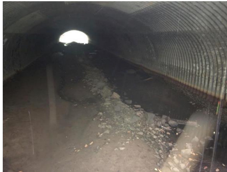
4.) Hwy 8m Arch culvert accommodates wildlife passage
