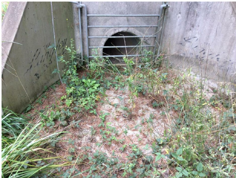
Photo 2. North Argonaut Road Ditch at 0+180m, the ditch passed through a driveway culvert approximately 50m southwest of the western property boundary, no evidence of flow was observed at this location or within 30m of the proposed development.
