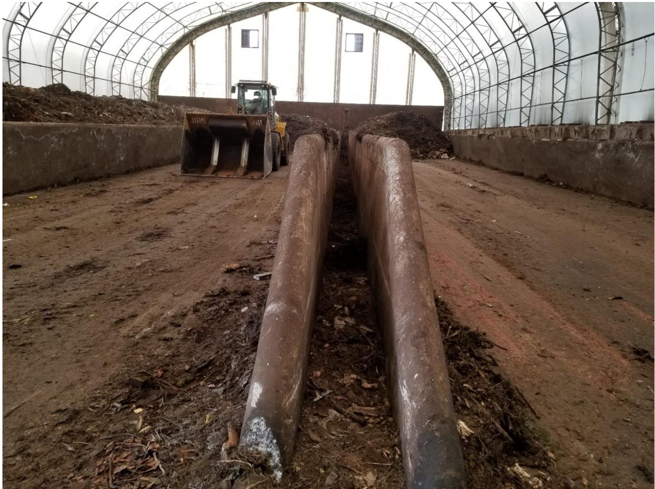
FIGURE 2: TYPICAL PRIMARY AND SECONDARY COMPOSTING FACILITY BUILDING INTERIOR (POURED IN PLACE FOUNDATION) PLEASE REFER TO DRAWING # 209 AND #210 FOR FURTHER DETAILS
