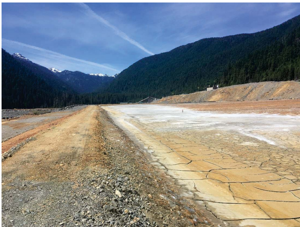
Photo 3: Dessicated surface of the APA, near the East Decant.
