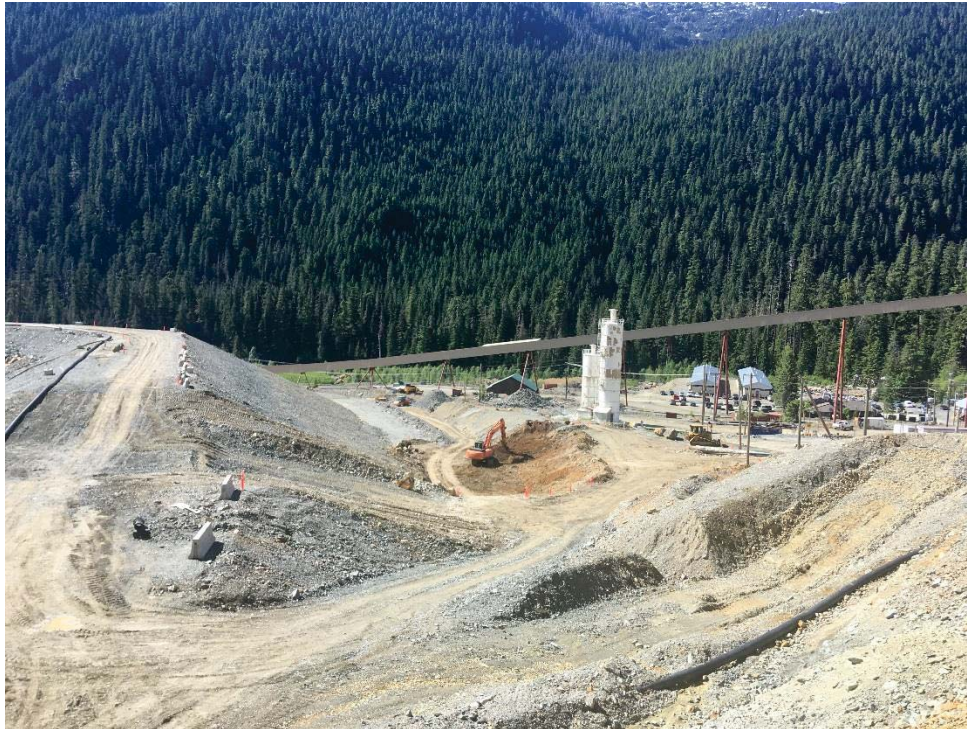
Photo 7: Spillway armouring fully removed. Excavation for raise foundation preparation is underway in Panel 4 area.
