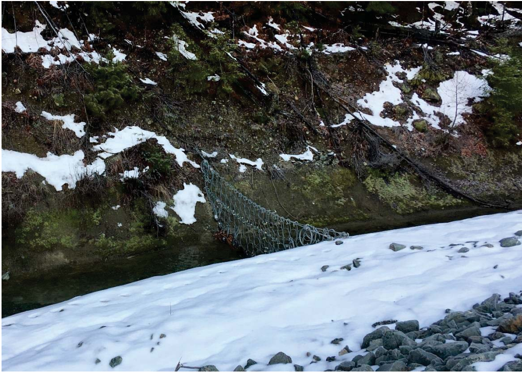
Photo 9: Minor debris in the bottom edge of the debris net.
