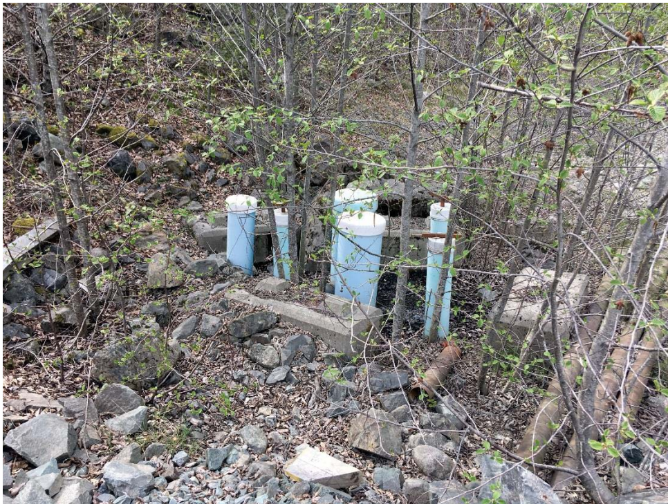
Photo 10: Trees growing around outer drain risers.
