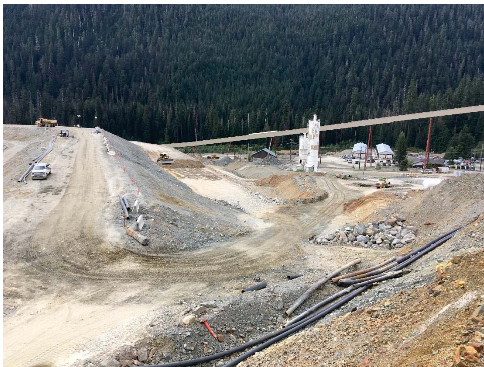
Photo 7: Construction of the downstream shell continues.
