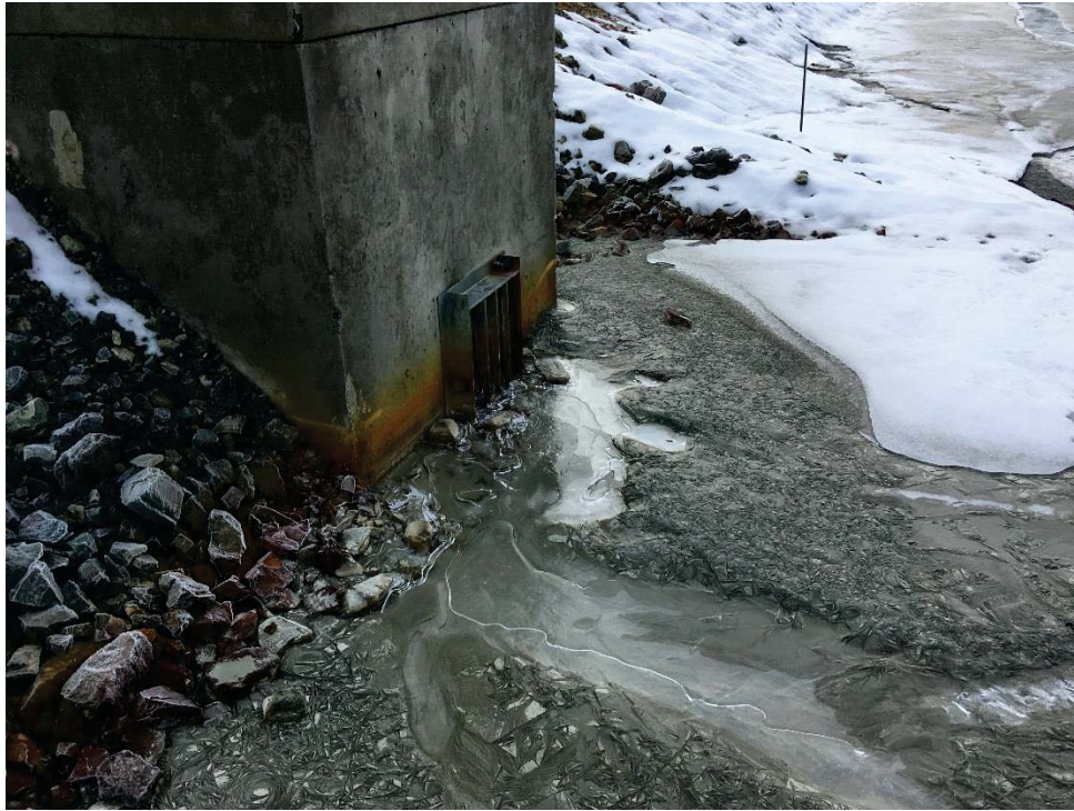
Photo 3: APA East Decant. Clear of debris. Frozen surface, no significant flow.
