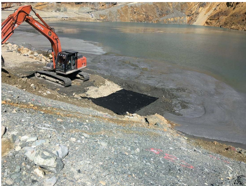
Photo 7: Construction on the upstream toe of the Lynx TDF dam raise (22 July).
