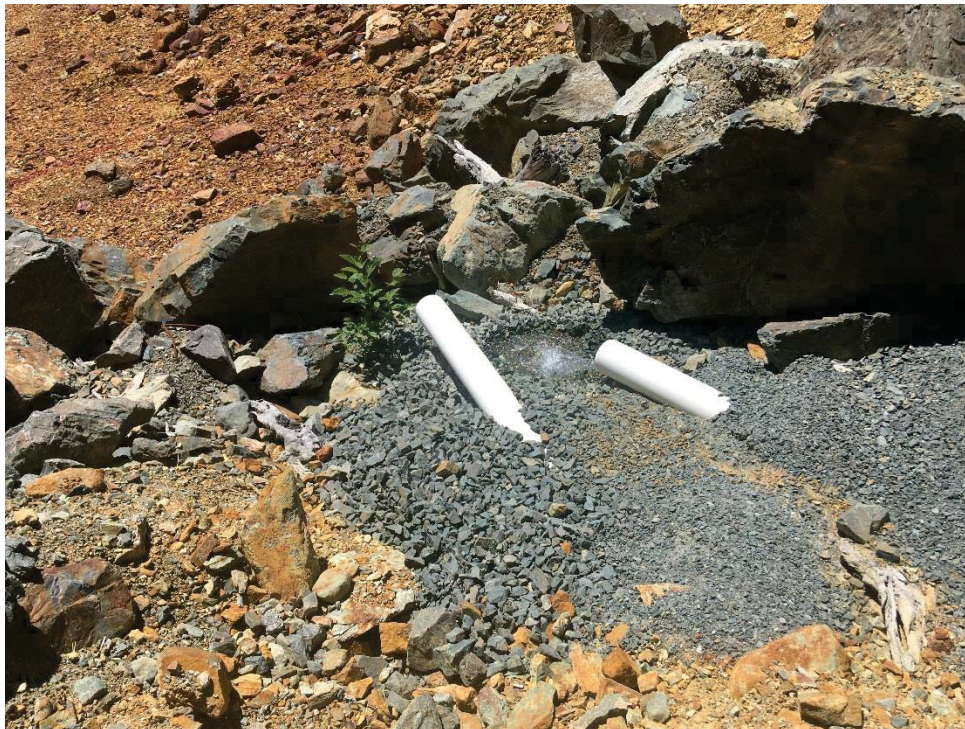
Photo 10: LLDD subdrain at the APA east abutment continues to flow at an estimated 0.5 L/s, similar to spring levels.
