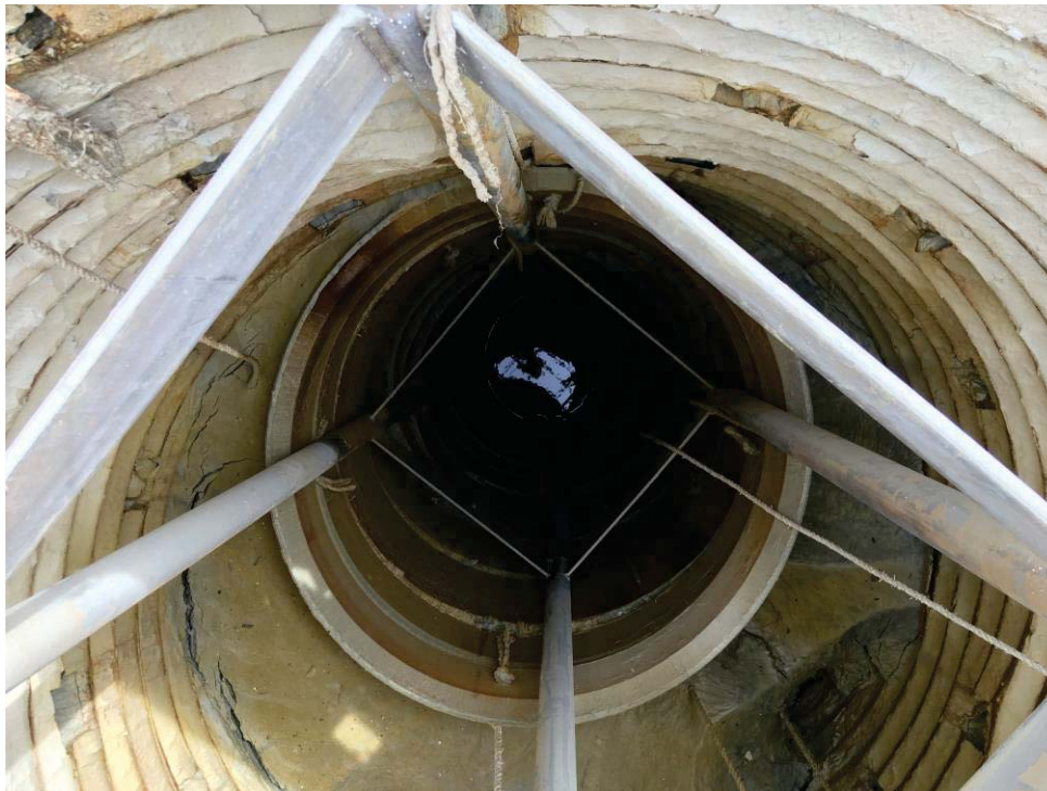
Photo 4: Looking down the old APA Decant. Water level in the tower is related to local groundwater phreatic level.
