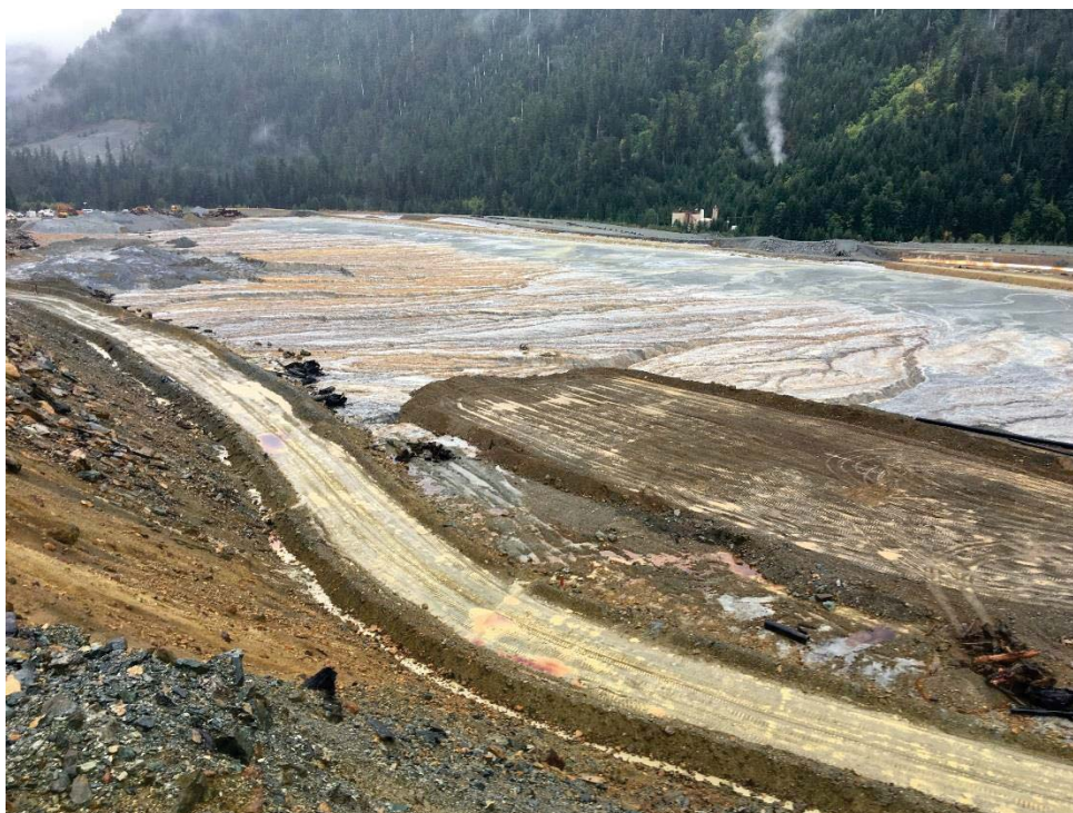
Photo 1: Overview of the Old TDF. Fill has been advanced from the laydown area to the east, covering a significant gully. Gullies should be filled with materials consistent with the tailings in order to reduce formation of preferential seepage pathways at closure.
