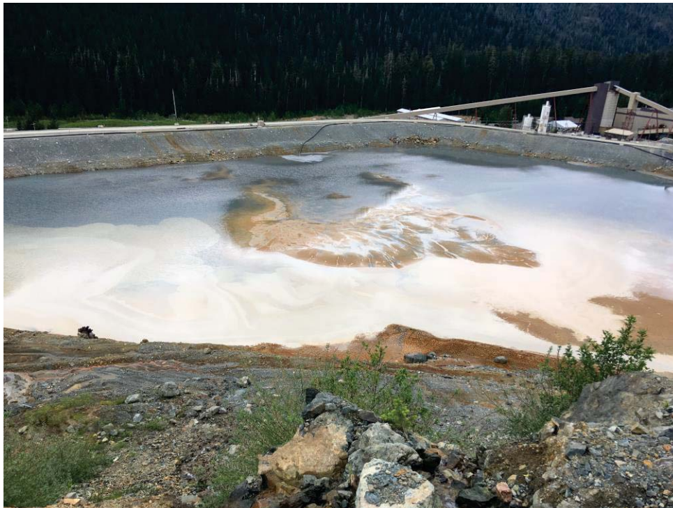
Photo 6: View from above the Lynx Springs Drain capture area showing slurry tailings deposition point on the south arm of the dam near Plane E and mud wave formed in dredgate following slurry deposition.
