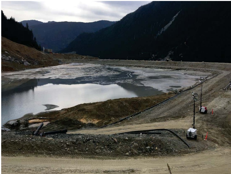
Photo 6: View of Lynx TDF from the 10L portal. The base lift/platform on the upstream side is complete. Construction on the upstream side has stopped pending additional stability modeling of the upstream slope configuration. Mud wave from paste deposition is visible.
