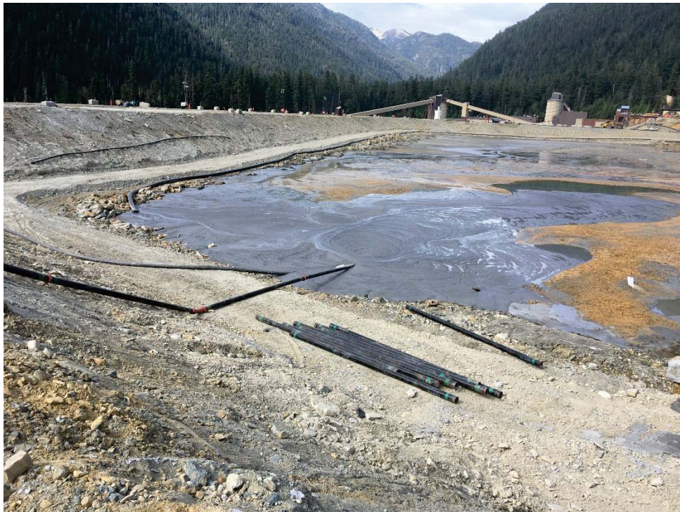
Photo 4: Paste deposition has commenced from the east arm of Lynx TDF Dam. The paste is displacing the dredgate, creating a significant mud wave.
