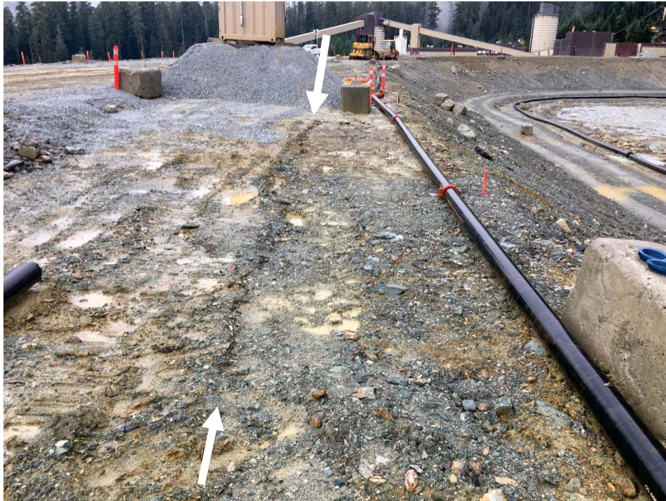
Photo 7: Crack on Lynx TDF Dam upstream crest near Plane E. The crack has apparent opening up to about 5 cm and has an apparent vertical offset of similar magnitude. This crack should be monitored for further development.
