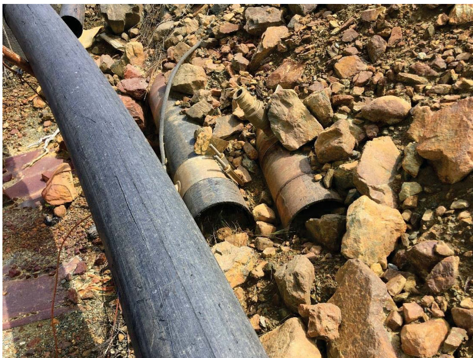
Photo 15: Example of stray disused pipes just above the Superpond liner.
