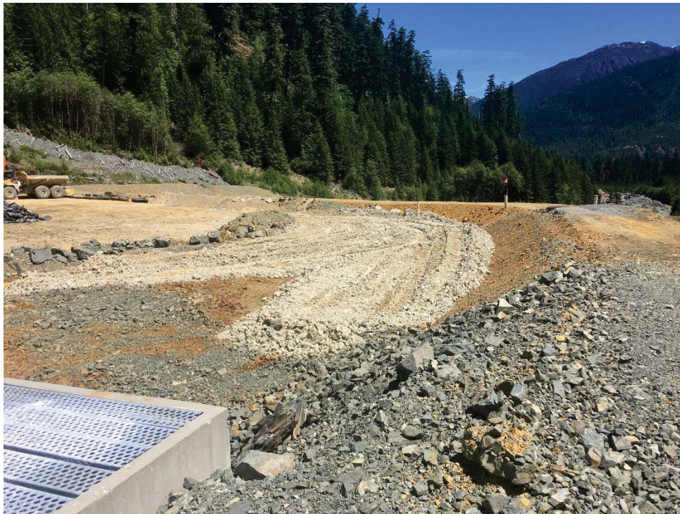
Photo 4: Stockpiles along the APA Berm crest removed. Some material was used to regrade the area and fill the closed depressions near the crest.
