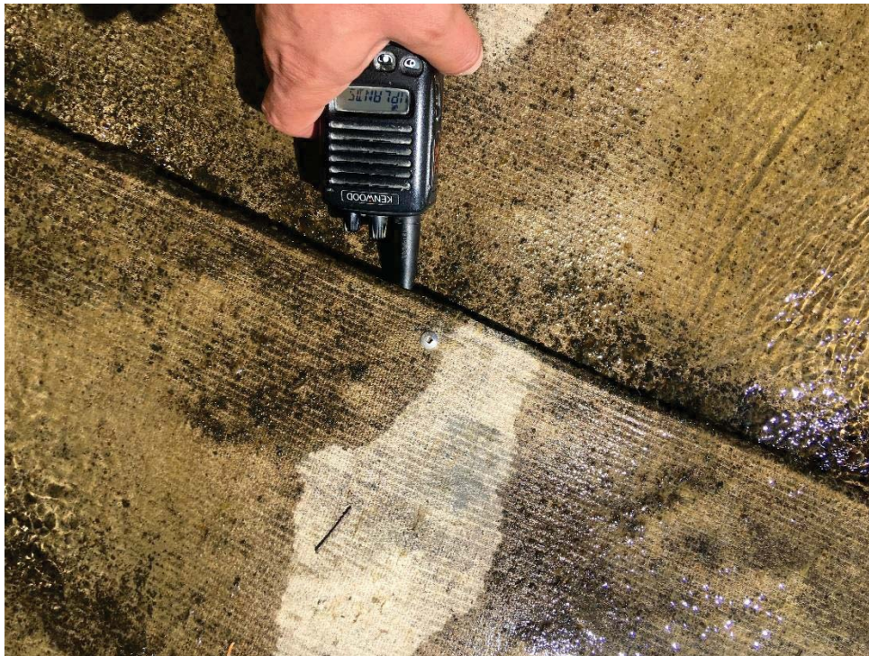
Photo 10: Closeup view of a delamination.
