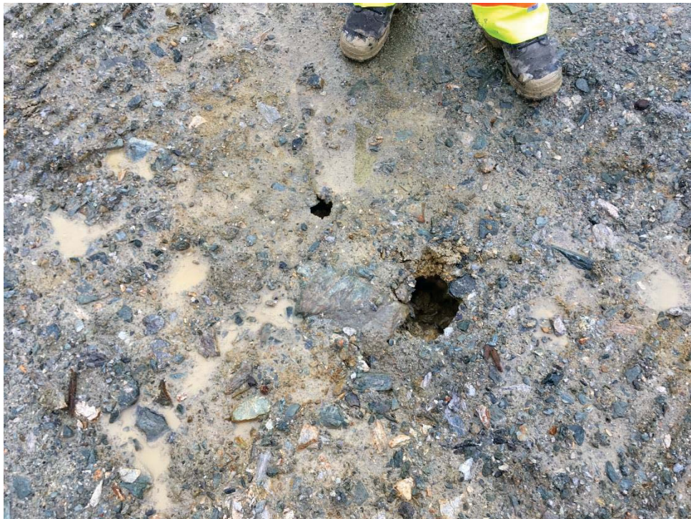
Photo 8: Voids found along the continuation of the alignment of the crack shown in Photo 7.
