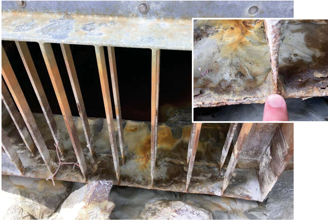
Photo 3: Corroded trash rack bars on the APA West Decant. East Decant is in similar condition.
