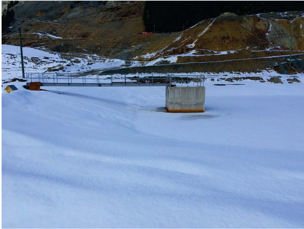
Photo 3: Old TDF Surge Pond decant with ice-covered pond. Water level is at design normal operating level for low flows.
