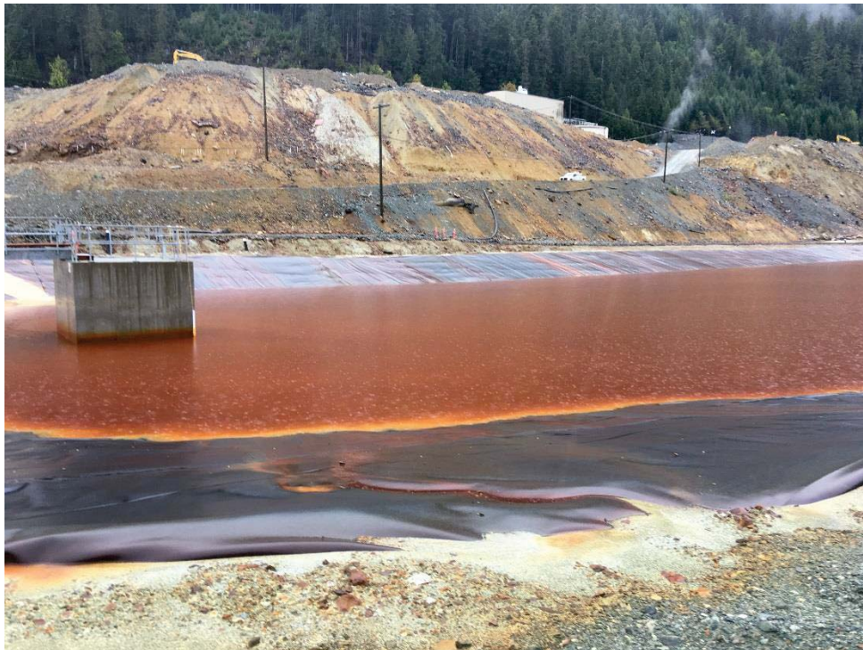
Photo 4: Old TDF Surge Pond water level is at the decant outlet, as intended.
