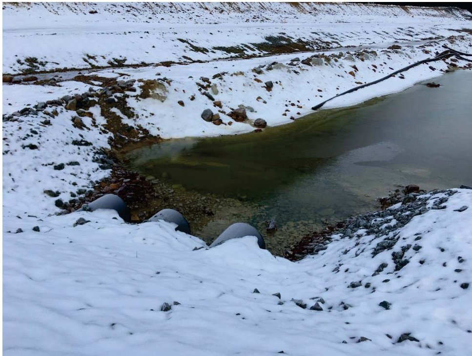
Photo 4: Water ponded upstream of APA Spillway Culverts. Depth is controlled by pipe invert.
