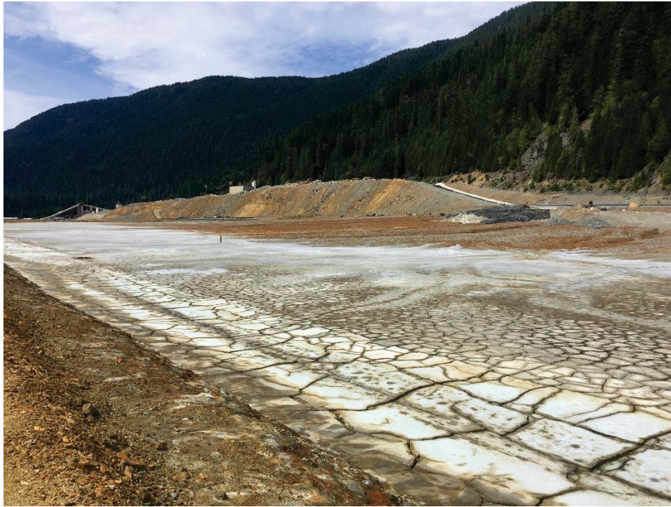
Photo 1: Old TDF viewed from near the East Decant. Surface has desiccated in the summer weather.
