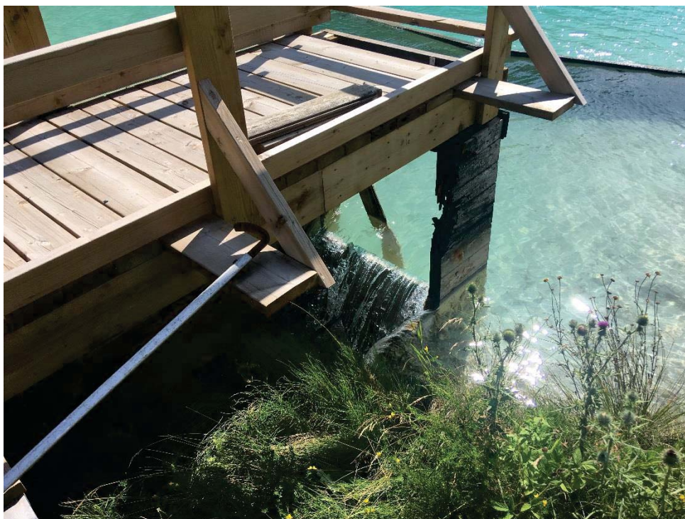
Photo 17: Example of a timber decant in poor condition.
