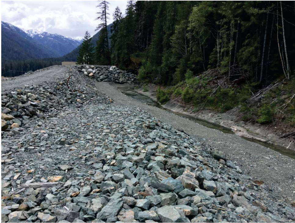
Photo 9: LLDD debris basin is clear of sediment/debris.
