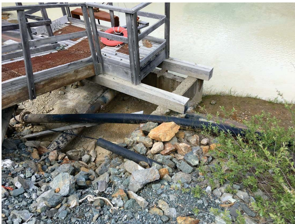
Photo 11: Poor condition of the upstream sump box for the secondary Superpond outlet.
