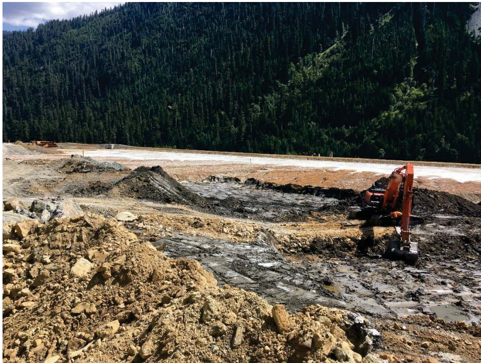
Photo 2: Tailings excavation at the apex of the APA for use in Lynx TDF construction.
