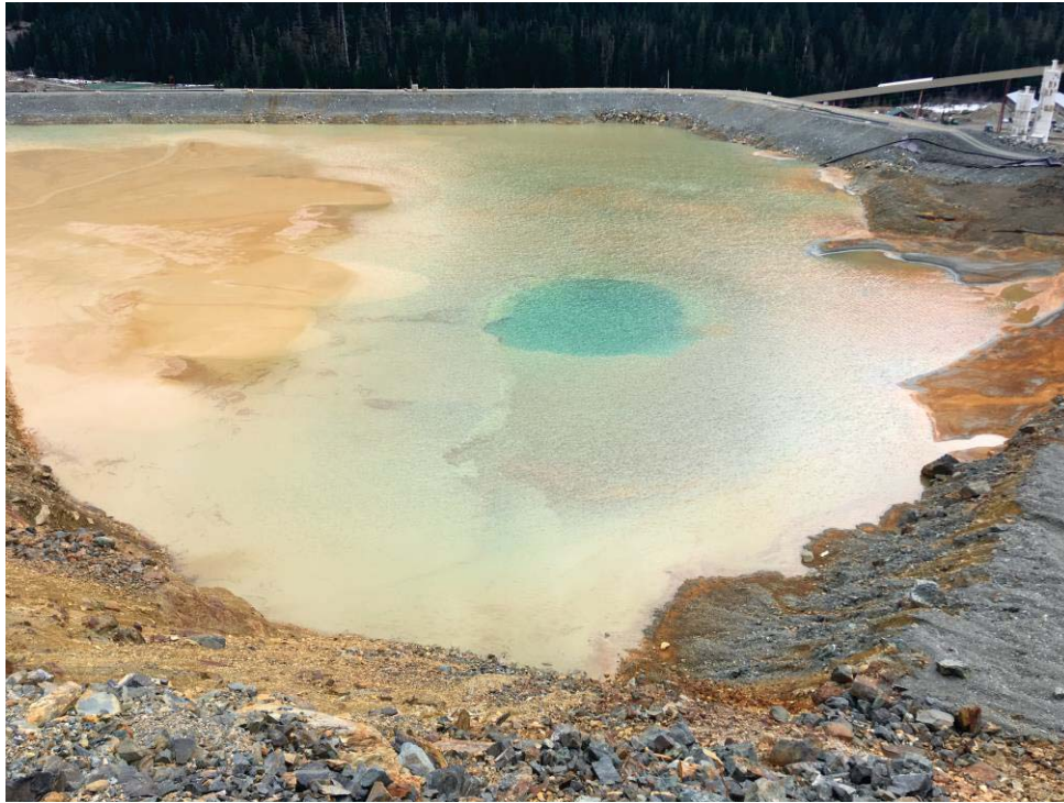
Photo 5: Lynx TDF sinkhole. The diameter is much larger than prior observations.
