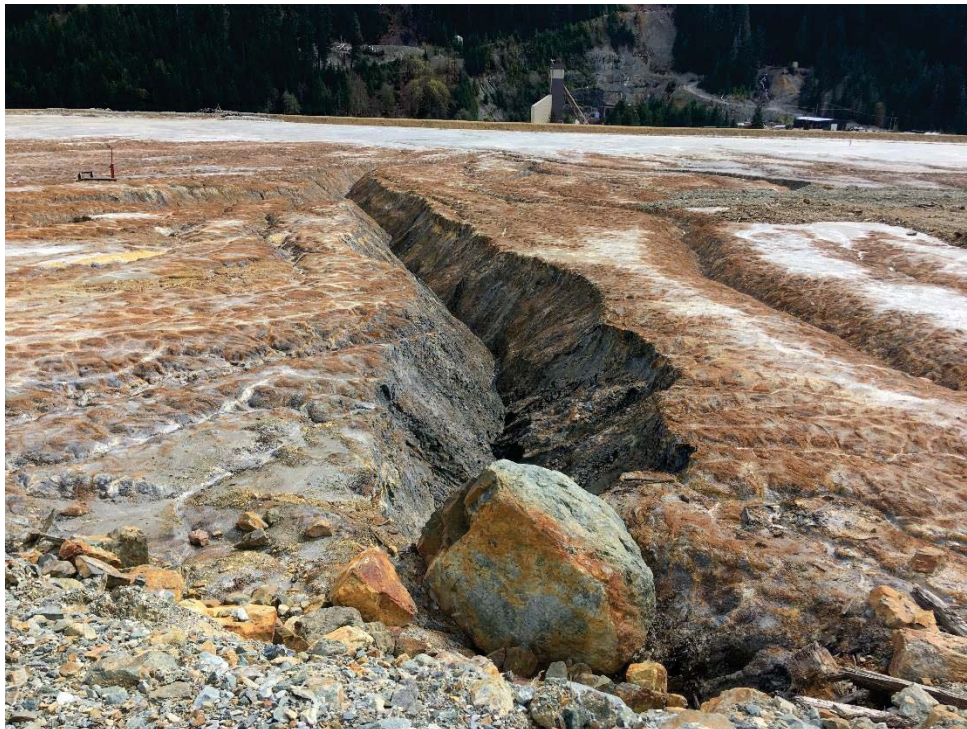
Photo 2: Active gully erosion on the APA below WRD 6
