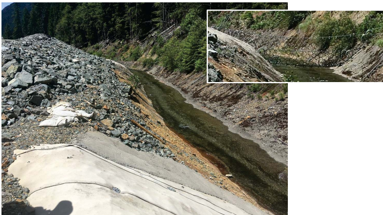
Photo 9: LLDD at the crest of the concrete cloth section. Debris net is clear (inset).
