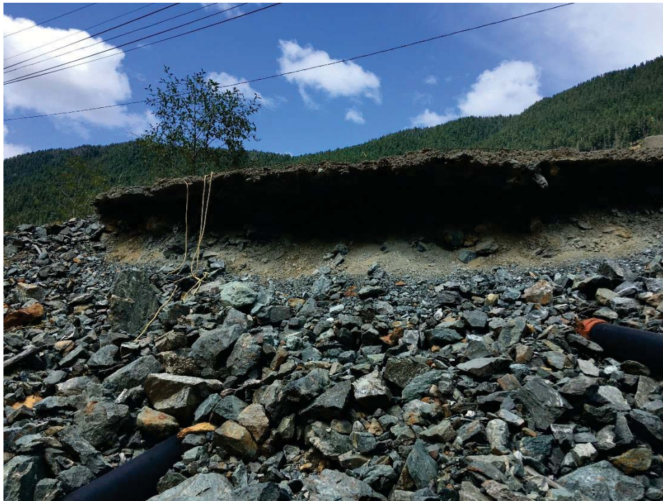
Photo 12: Undermined condition of the secondary outlet sump on the downstream side of the Superpond embankment.
