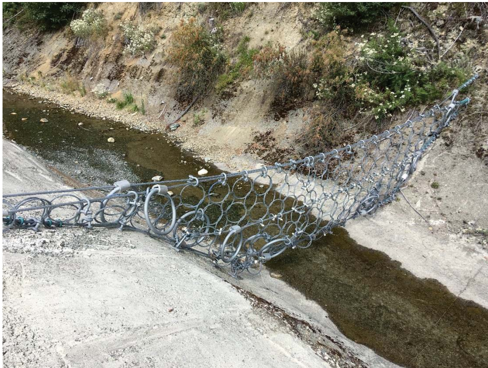
Photo 10: LLDD debris net is clear and in good condition.
