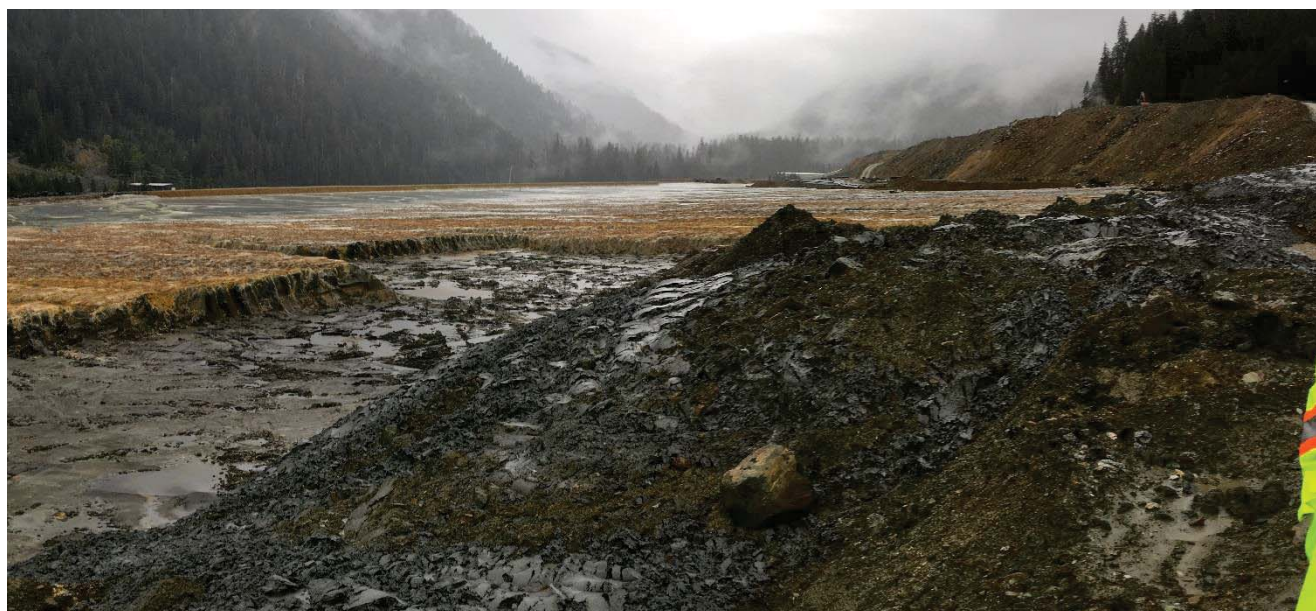
Photo 2: Cake material dumped above the excavations created during the summer. This material should be spread into the excavation if practical.
