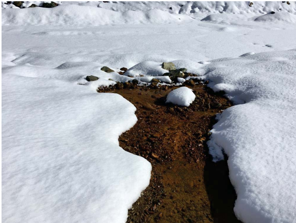
Photo 4: Seepage from the APA buttress drain outlet.
