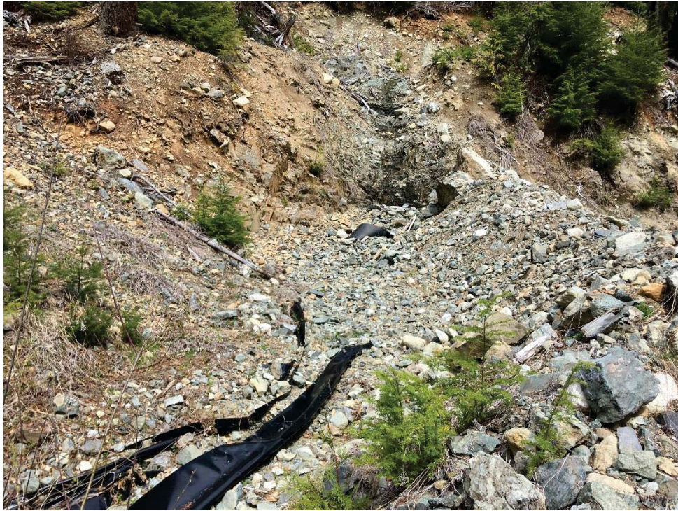
Photo 7: Damaged geomembrane liner at the Upper Arnica/Lower Arnica Diversion transition.
