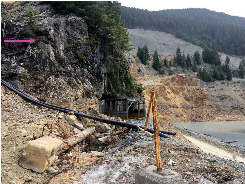
Photo 8: The ultimate final downstream crest of Lynx TDF Dam has been marked on the cliff above 10L East portal. Dam centreline is several metres on the other side of the portal.
