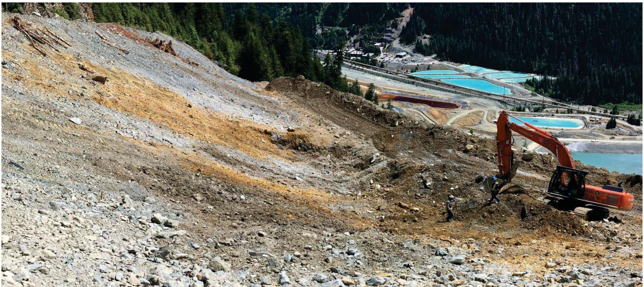
Photo 8: Removal of Waste Rock Dump 2 Phase 2, Area 1 is underway. The slope below the diversion is being trimmed at 1.5H:1V. Natural ground has not been encountered.
