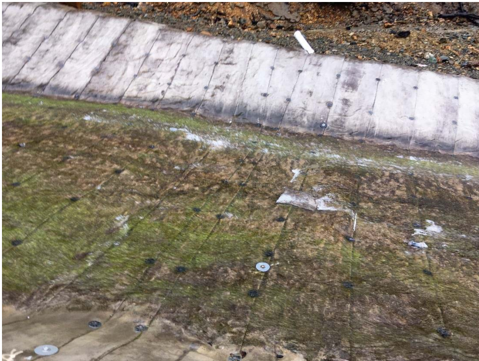
Photo 10: Repairs in the LLDD near the crest of the DD Hill, at the site of a puncture and delamination. The puncture has been patched and the delamination has been sealed with a caulking-type compound. This area should be monitored for performance in high-flows.
