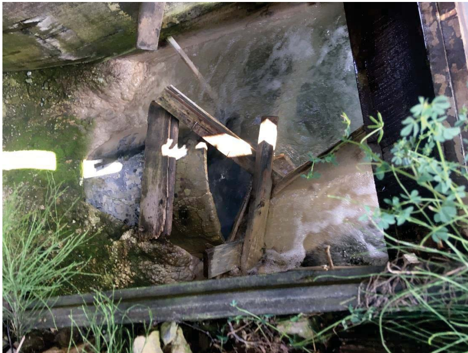
Photo 18: Wood debris partially blocking the decant shown above. This debris would be difficult to remove safely.
