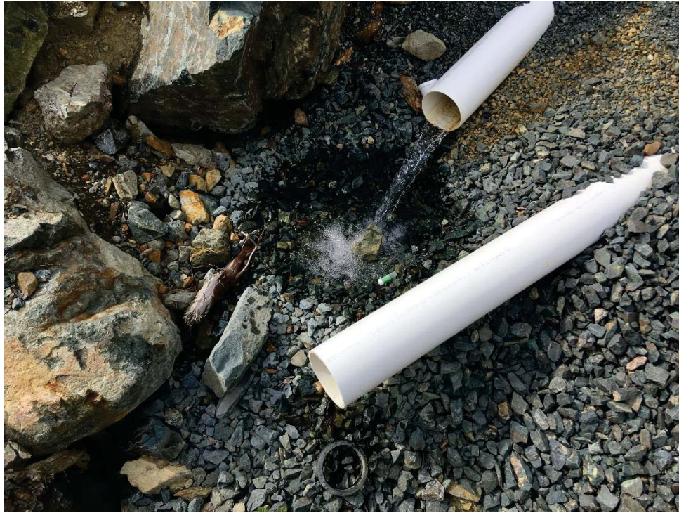
Photo 1: Subdrain flow at the APA East Abutment
