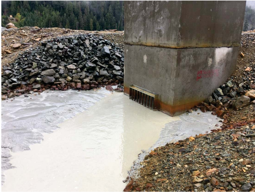
Photo 3: Moderate flow through the APA west decant. Note the turbidity of the water.
