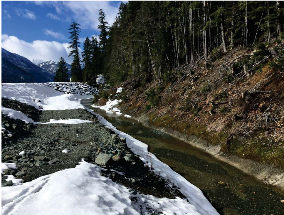
Photo 9: LLDD debris basin clear of accumulation.
