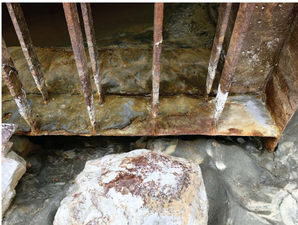
Photo 3: Corrosion damage to the trash rack at the APA West Decant
