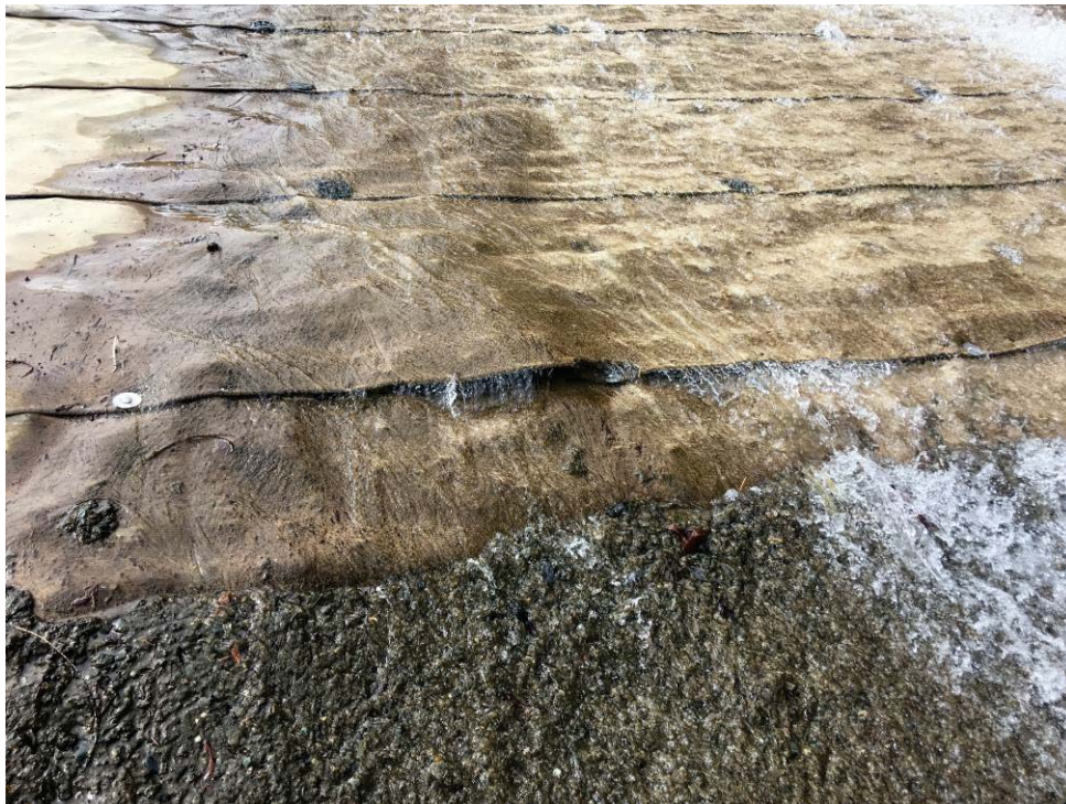
Photo 10: Example delamination near the terminal section of the LLDD.
