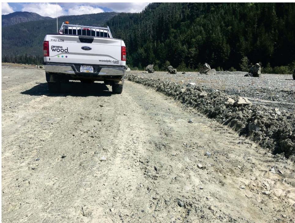
Photo 3: Windrow on the Seismic Upgrade Berm (22 July). This was regraded prior to 29 July.
