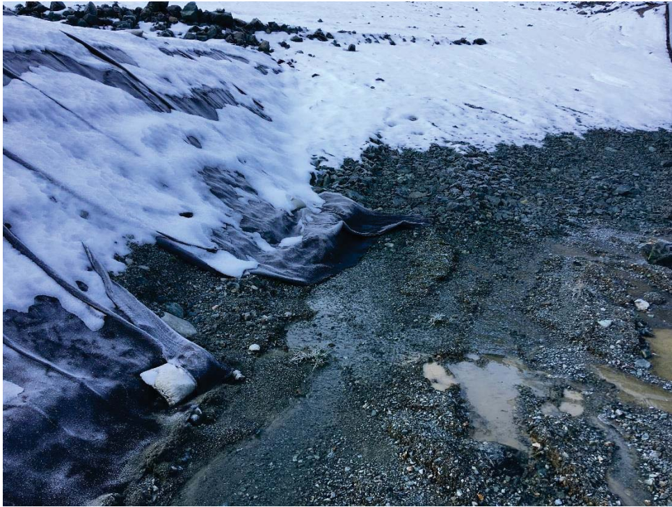
Photo 7: Seepage adjacent to the Lynx Spring Drain
