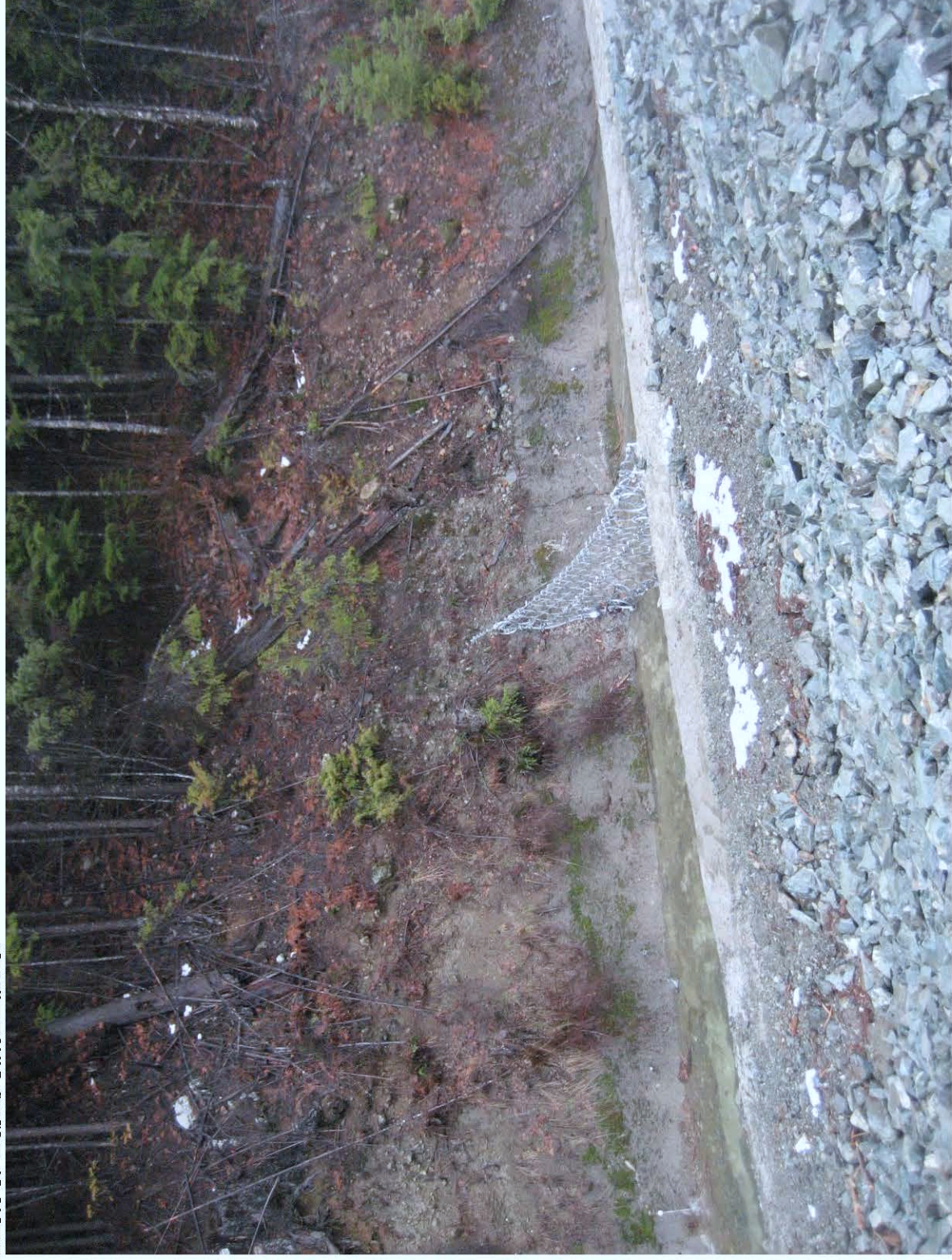
Photo 8: Debris Catch Barrier
