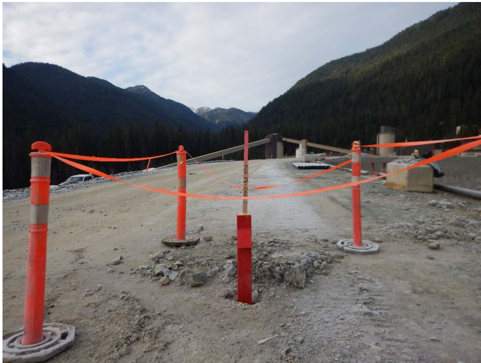
PHOTO 53: BH19_04 Protective cover installation using bentonite chips (December 30, 2019)
