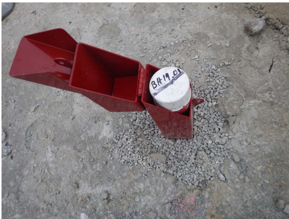
PHOTO 55: BH19_01 Protective cover installation using bentonite chips (December 30, 2019)
