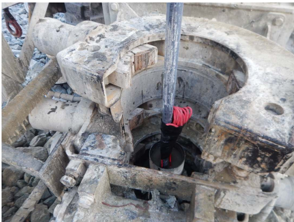
PHOTO 37: BH19_02 VWP Installation (November 29, 2019)
