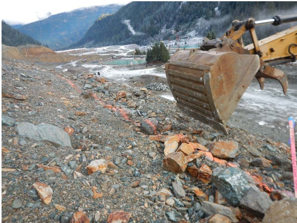
PHOTO 12: Excavator removing large rocks along Path for MASW19-02 Seismic Investigation (November 26, 2019)
