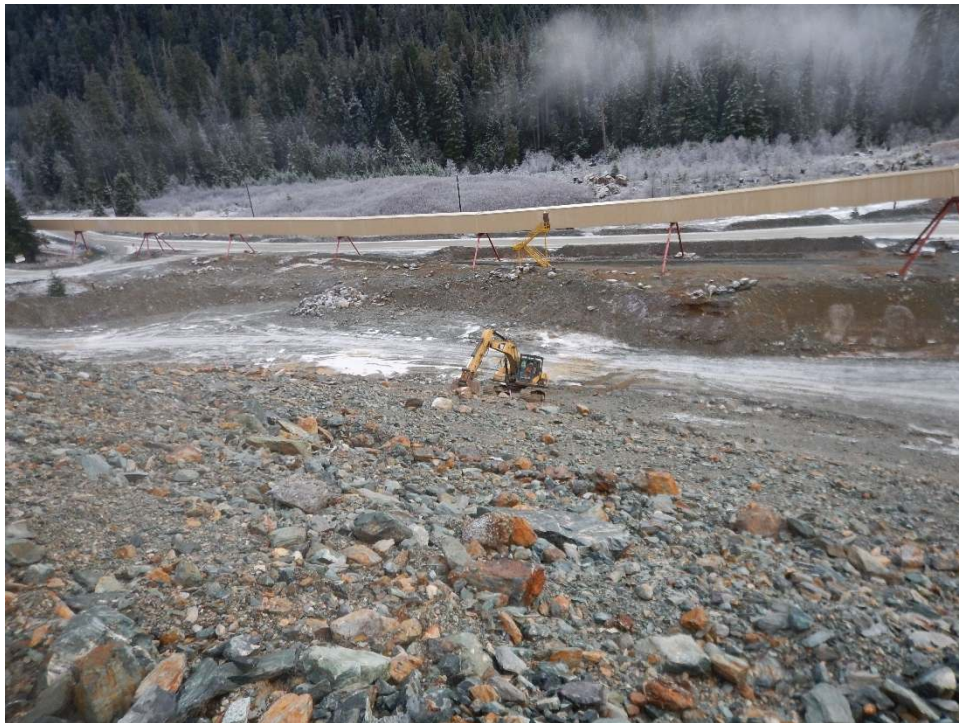
PHOTO 11: Excavator Creating Path for MASW19-02 Seismic Investigation (November 26, 2019)
