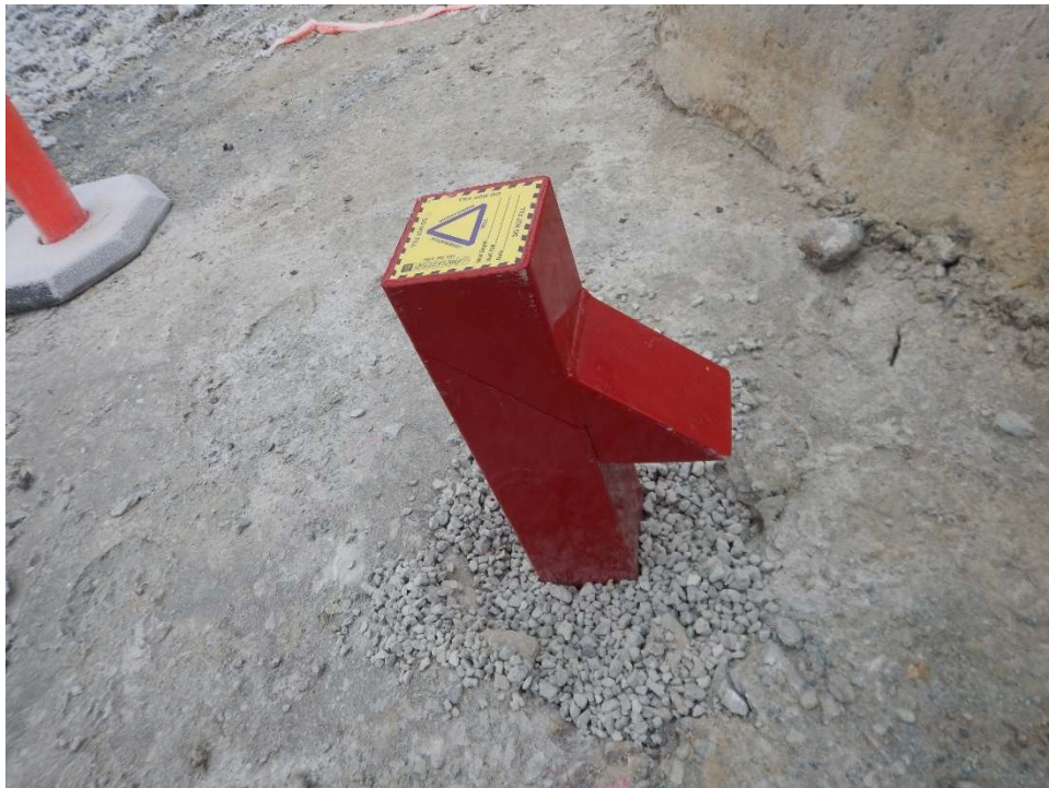
PHOTO 52: BH19_04 Protective cover installation using bentonite chips (December 1, 2019)
