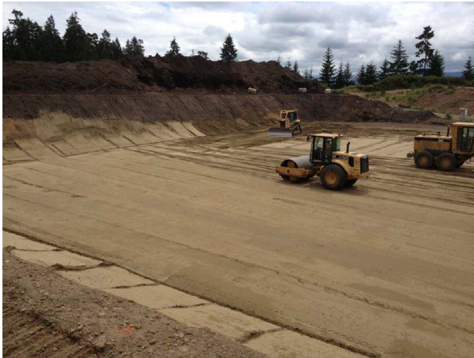
Photo 3 - Compaction of Sand Protection Layer – Looking Southeast - 2015
