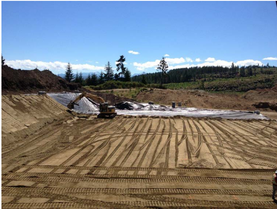
Photo 5 - Bottom Liner and Leak Detection Layer Installation – Looking South - 2015
