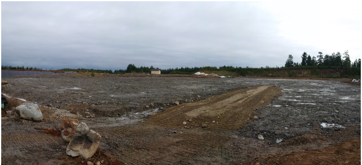
Photo 15 - Graded Intermediate Cover over Lined Cell – Looking East - December 2017
