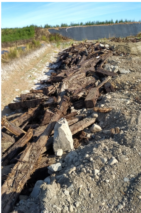
Photo 13 - Cover Soil Application over Waste Timber – Looking North - 2017
