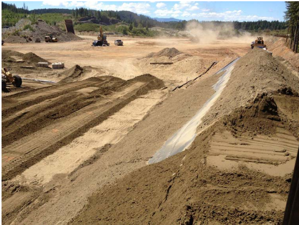
Photo 6 - Leak detection layer installation – Looking West - 2015
