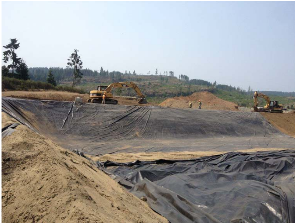
Photo 9 - Liner Installation – Looking Southwest - 2015
