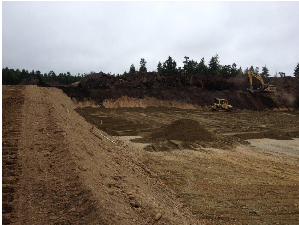
Photo 2 - Sand Protection Layer – Looking East - 2015
