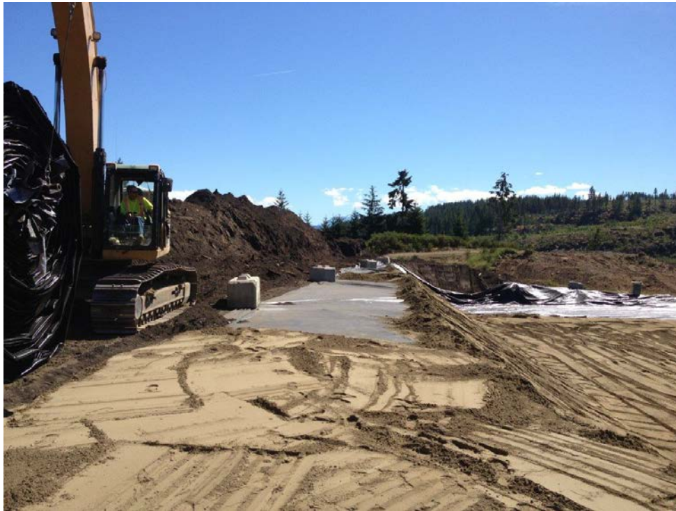
Photo 7 - Leak Detection Layer Installation – Looking South - 2015
