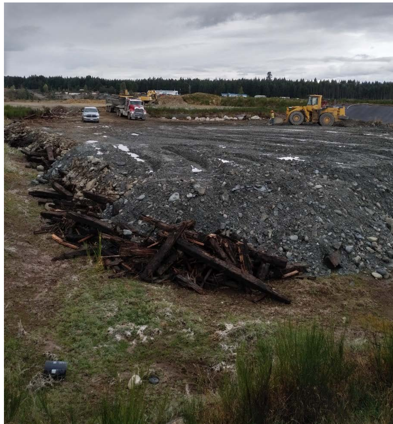
Photo 12 - Cover Soil Application over Waste Timber – Looking Northwest - 2017
