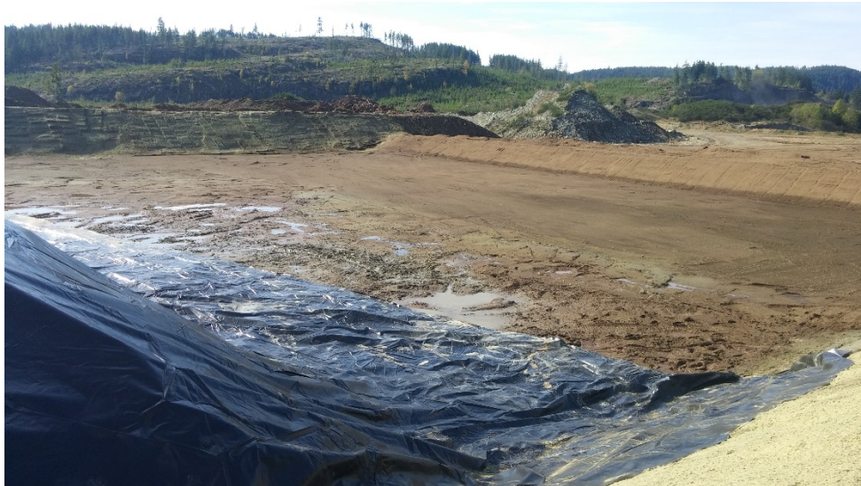
Photo 10 - Completed Lined Cell with Covered Waste – Looking Southwest - 2015
