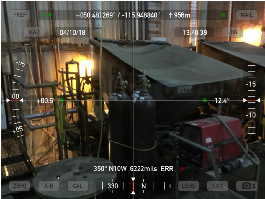
No valve protection cap
