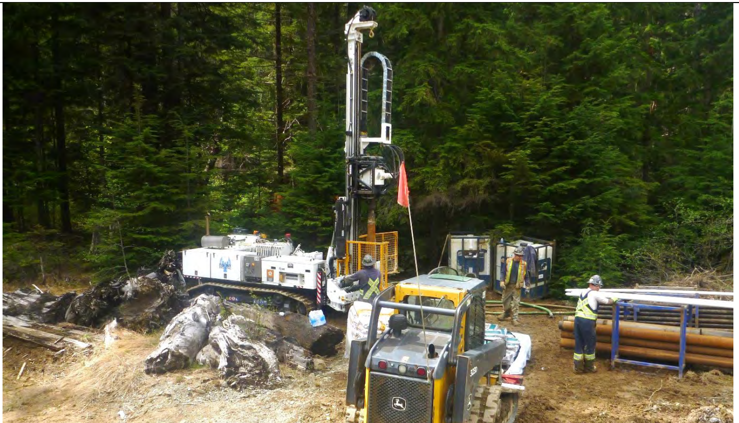
Photo 2: Site set-up at MW18-07S/D during drilling. Drill rods and casing were carried from the rack to the drill rig. The John Deere 323d Terrain Loaded was used to transport drill equipment and materials between drilling locations.
