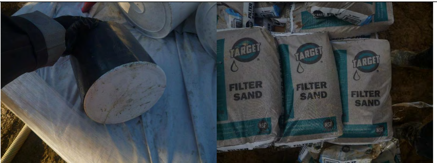
Photo 4: End cap used for pumping wells (left). 10/20 filter sand used for all installations (right).
