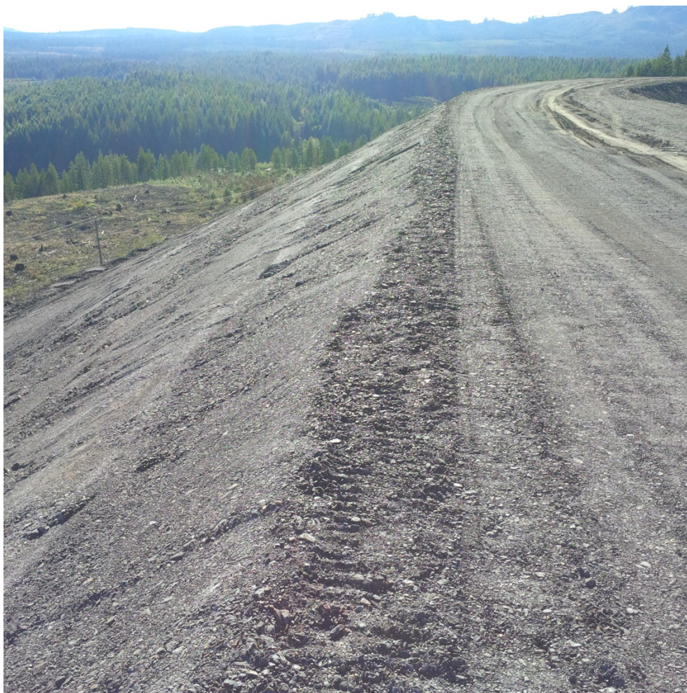
Photograph 7: Downstream Face After Re-sloping, Looking Northwest, September 11, 2015.
