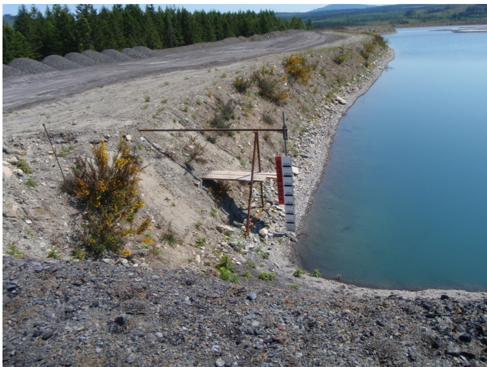
Photograph 11: East Embankment Upstream Slope with Freeboard Gage, Looking South, May 26, 2015.
