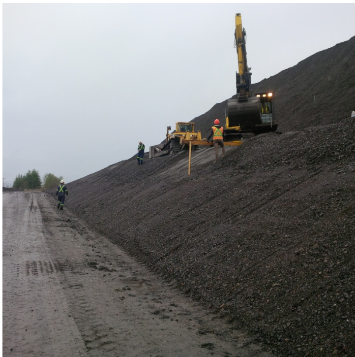
Photograph 5: Placing Coarse Coal Rejects, Looking North, September 2, 2015.
