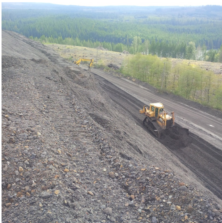
Photograph 6: Widening The Downstream Slope, Looking South September 8, 2015.
