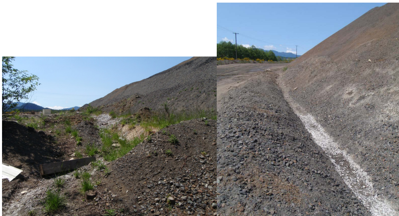
Photograph 19a (left): South Embankment Drainage Ditch Along Downstream Toe, Looking West, and 19b (right): Looking Northwest, May 26, 2015.
