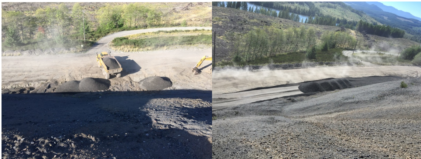
Photograph 4: Placement Coarse Coal Rejects To Widen The Downstream Toe, Looking West, August 18, 2015.
