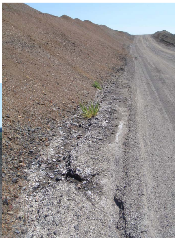
Photograph 26a (left): West Embankment Access Ramp, Looking South, and 26b (left) Seep and Soft Ground, Looking South, May 26, 2015.
