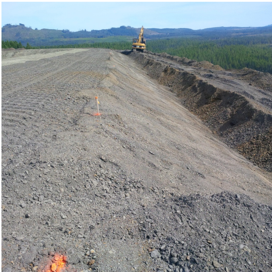
Photograph 3: Re-sloping At Downstream Crest, Looking South, August 17 2015.
