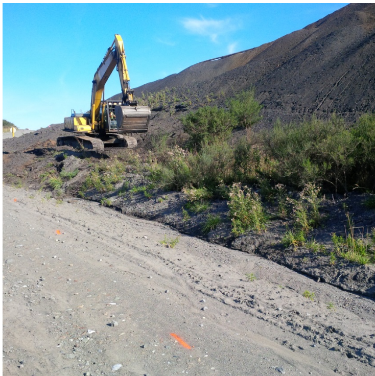
Photograph 1: Removing Vegetation From The Downstream Slope Of The West Embankment, Looking North August 17, 2015.
