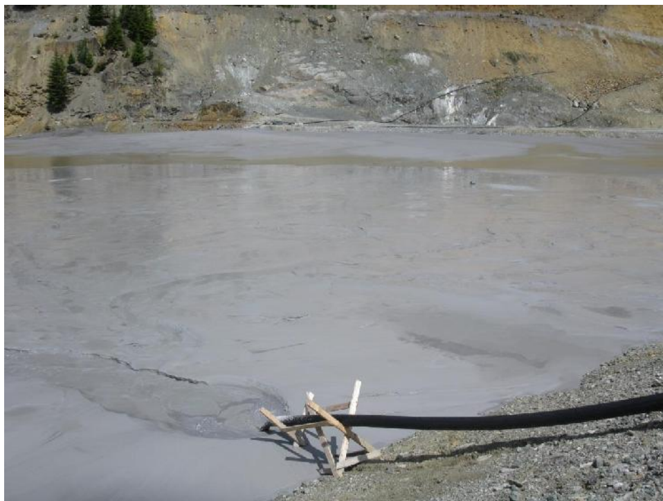
Photo 22 – Sand tailings deposition from center of Lynx Dam south arm, looking north/northeast.
