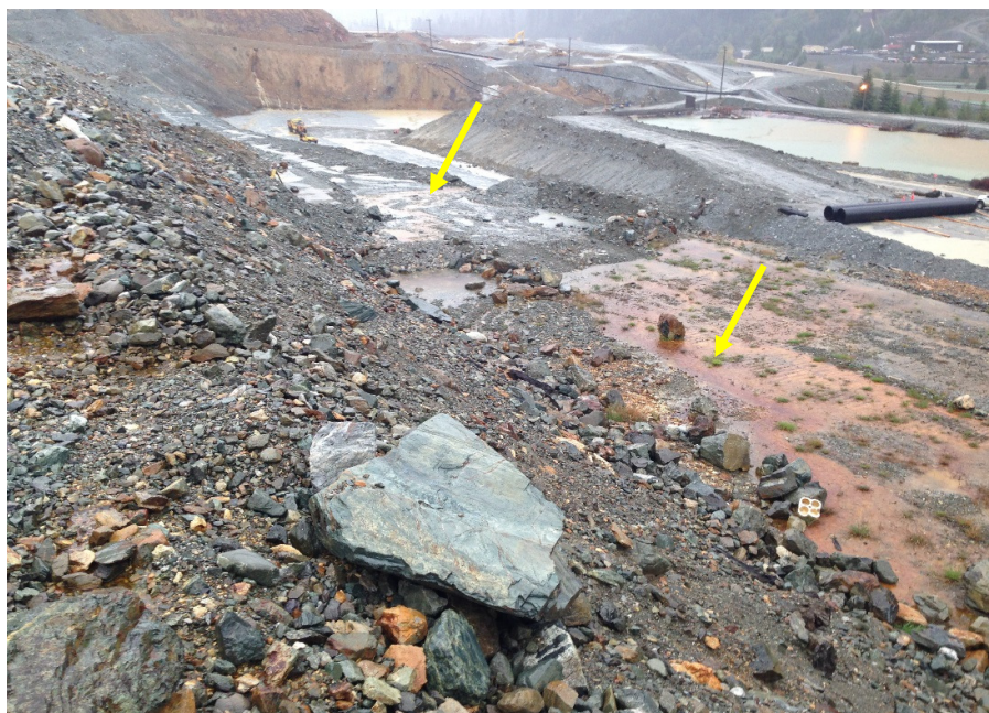
Photo 26: Seepage and surface runoff on Lynx Dam mid-level "2011" bench, looking southeast (September 24, 2015).
