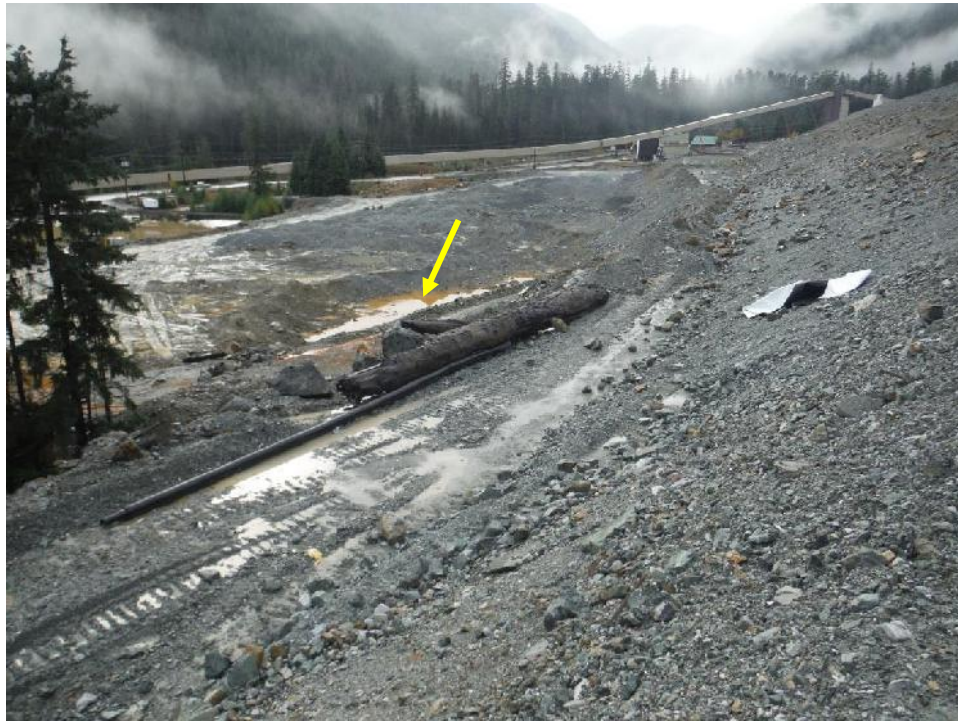
Photo 31 – Easternmost lower bench and toe of Lynx Dam south arm, looking west. ARD ponding between the remains of “Zone J material” Superpile and the dam toe.
