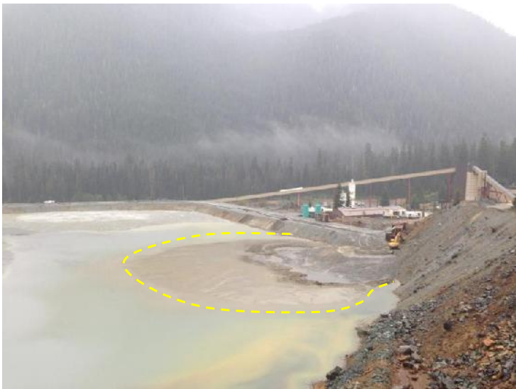
Photo 22 – Eastern half of Lynx TDF, looking southwest. Dumped material at the west abutment has created a mud wave (dashed line). Ponded water at the back of pit exhibiting ARD staining.
