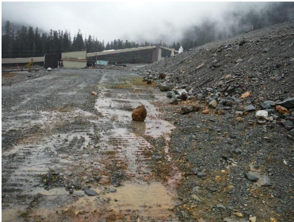
Photo 28 – Seepage on the “2011 Bench” of Lynx Dam, looking west.
