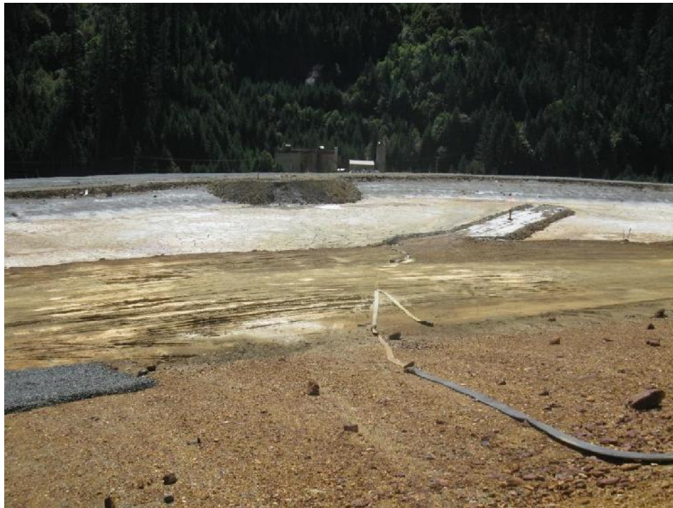
Photo 3 – 4:1 Slope and base of the Paste Berm and East Strip near Instrument Plane C, looking southeast (no water accumulation or trace of seepage).
