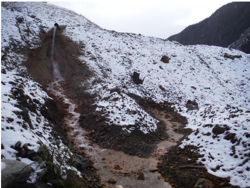
Photo 22 – Phillips Reach discharge below Waste Dump #1. Note seepage at the right side of photo.
