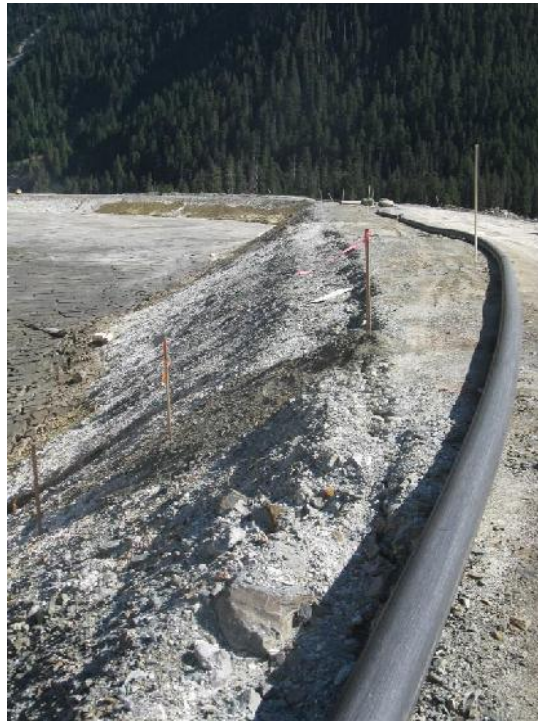
Photo 19 – Close-up view at the sloughing zone in the upstream shell of Lynx Dam west arm, looking south.
