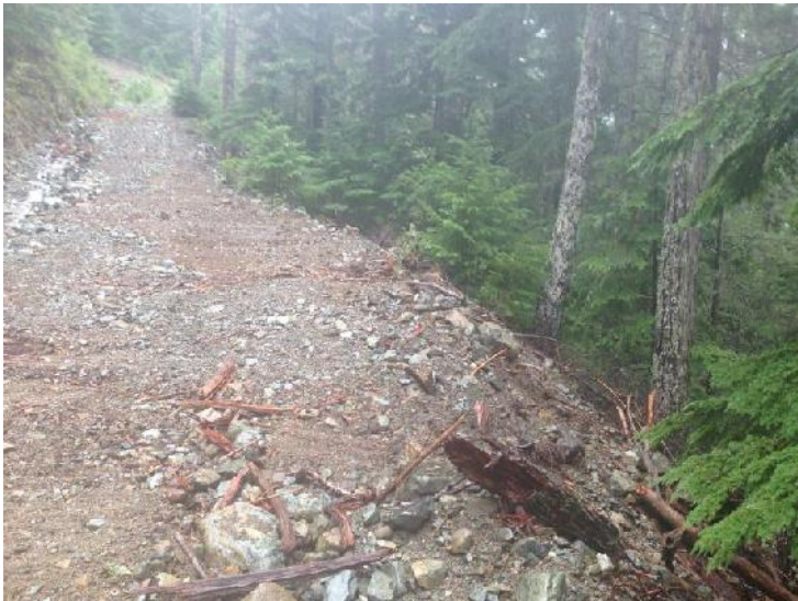
Photo 40 – Fill side-cast over wood and against trees during lower Arnica Reach repairs – side-cast material should be pulled back and used to increase freeboard by raising the road.
