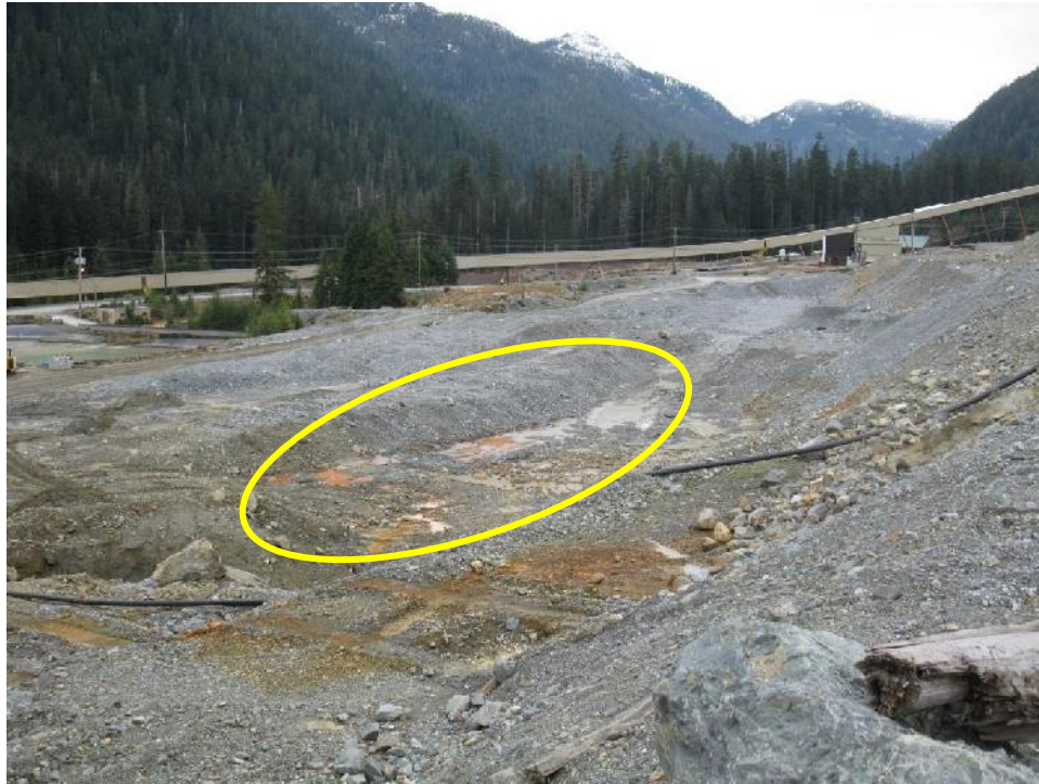
Photo 19 – Lynx Dam south arm east lower benches and toe area, looking west, showing ponding at the toe of the 'Zone J material' stockpile.
