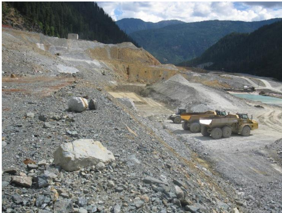
Photo 16 – Lynx Dam south arm toe looking east from the mid-level bench (note the foundation preparation work in the 3410 m elevation toe area).
