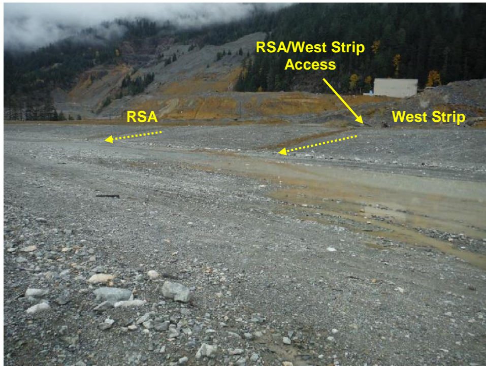
Photo 19 – ARD runoff on the 6:1 Slope coming in from the RSA/West Strip access and ponding on the surface of the Seismic Berm, looking northwest.
