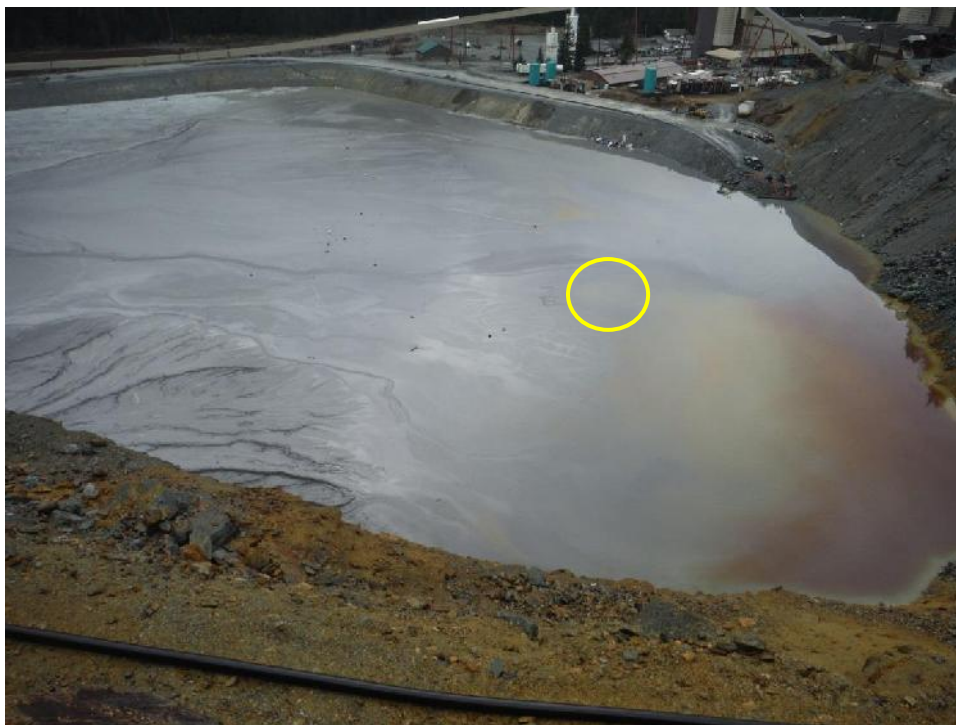
Photo 22 – Southwest view of Lynx TDF with sinkhole barely visible (circled area).
