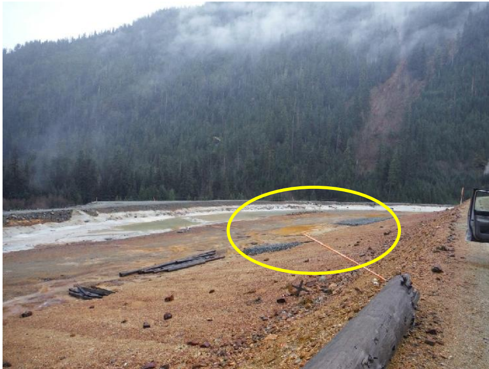
Photo 11 – View of the East Strip showing ARD seepage areas at the downstream toe of the Paste Berm and “anti-piping” pads (circled), looking south from the east abutment.
