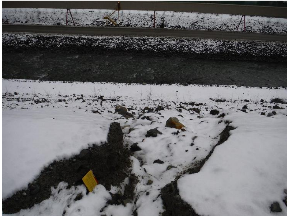
Photo 11 – New erosion gully into the Seismic Berm downstream face, just east of the Old TDF spillway.
