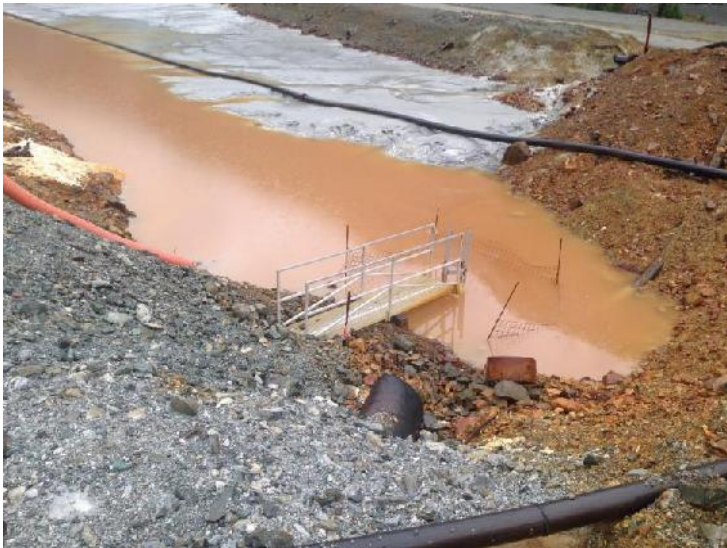
Photo 12 – Gangway leading to the Strip decant (under water).
