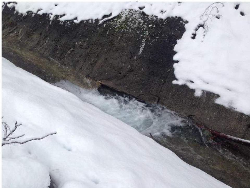
Photo 20 – Close-up view of a hole in the shotcrete lining of the Lower Lynx Diversion Ditch (see the circled area on the previous photo).
