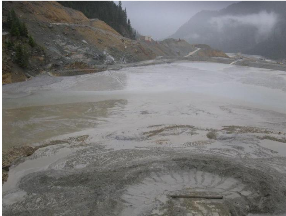
Photo 17 – Overview of Lynx TDF, looking east, with excavated materials from the RSA disposed near the west abutment in foreground.
