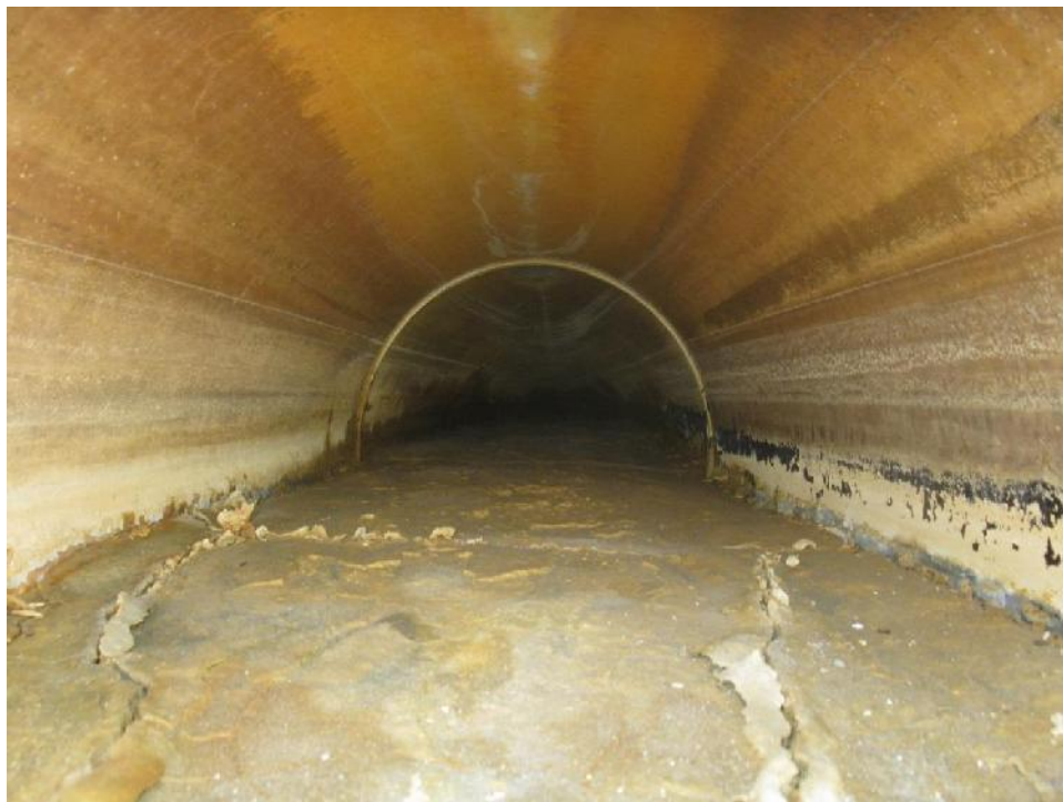
Photo 6 – Interior of one of the culverts under the Old TDF spillway. Culvert is completely plugged with tailings solids.
