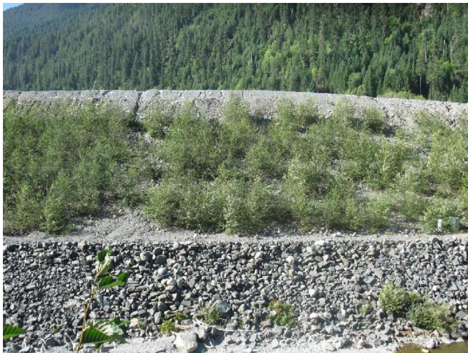
Photo 10 – Slope and rockfill toe of the Seismic Upgrade Berm, ~ Sta. 1+100.
