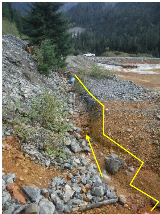
Photo 8 – Main spring at the toe of the Paste Berm east abutment, looking towards the north end of the East Strip.
