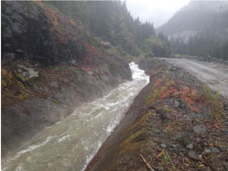
Photo 19 – Moderate flow in the shotcrete-lined section of the Lower Lynx Diversion Ditch, looking east (downstream).
