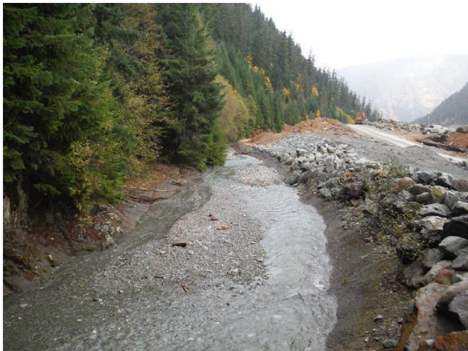
Photo 22 – Lower Lynx Diversion Ditch near Cascade Reach, looking east. Note the presence of gravel bars along the channel.
