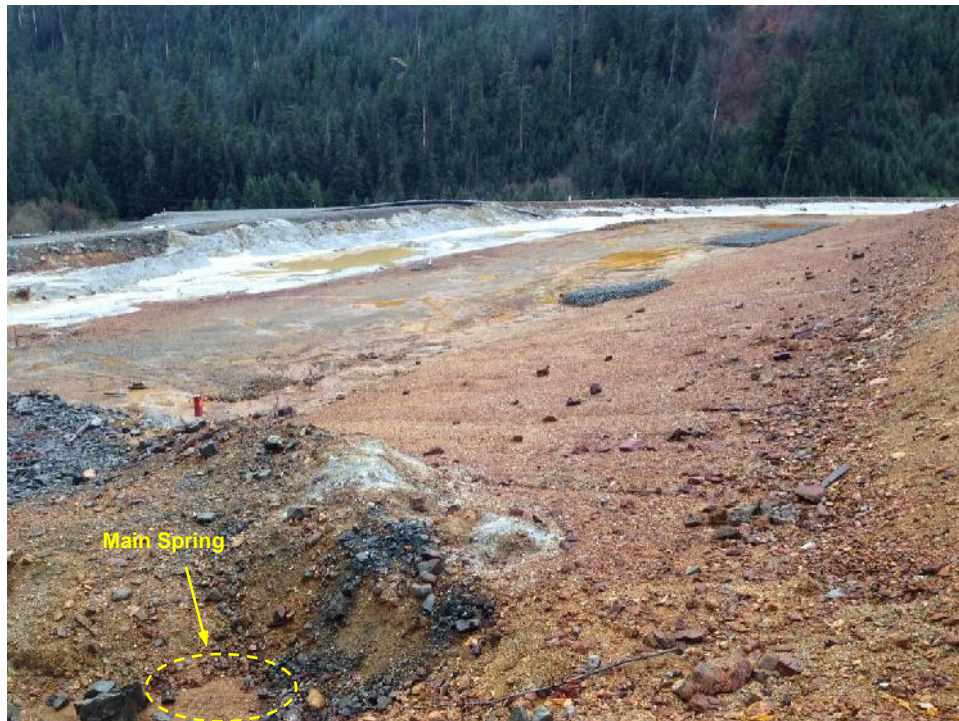
Photo 5 – East abutment of the Old TDF and seepage areas along the toe of the APA Paste Berm, looking south.
