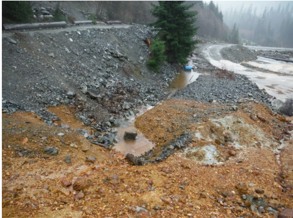
Photo 7: High water flow out of the main spring at the Paste Berm east abutment, looking east (November 27, 2014).
