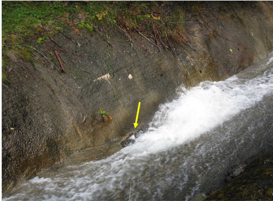
Photo 45: Hole in shotcrete lining of the Lower Lynx Diversion Ditch (October 31, 2015).
