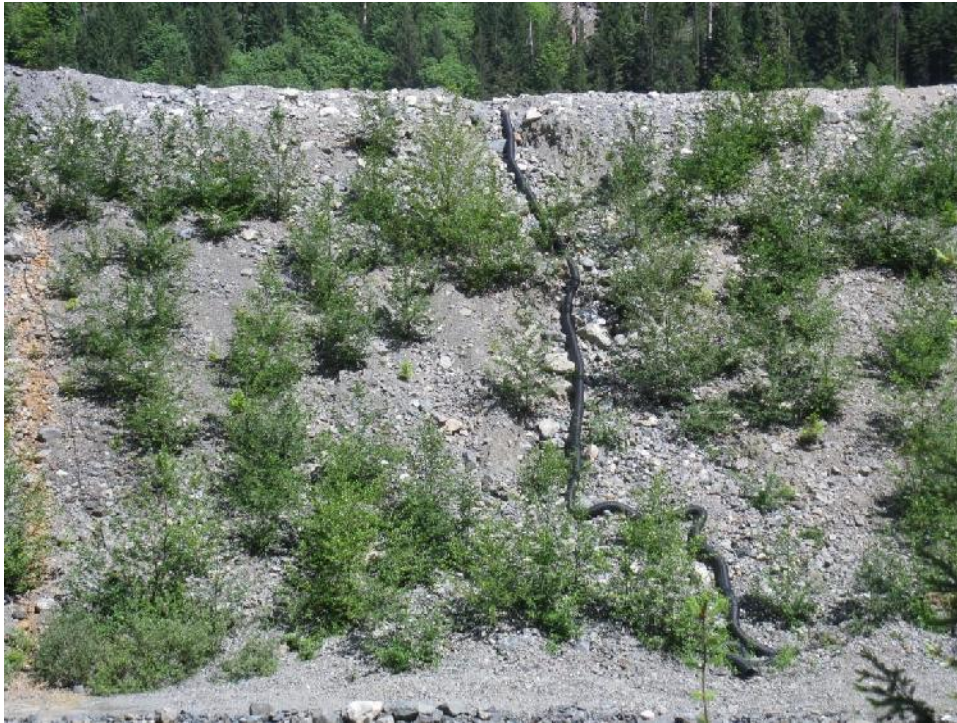
Photo 17 – New drainage pipe on the Seismic Berm downstream face.
