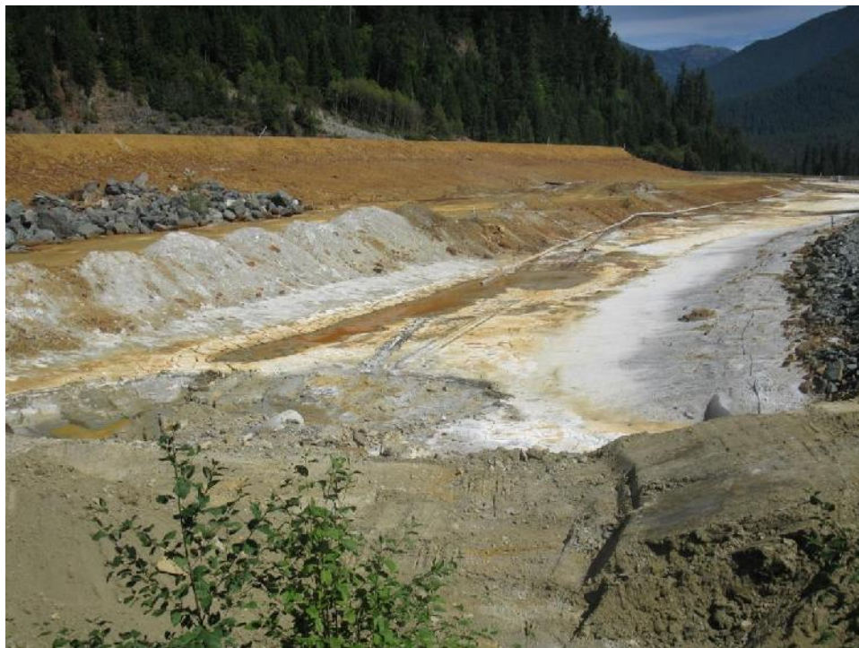
Photo 4 – Paste Berm and East Strip looking east from the Old TDF spillway. Excavation is in preparation for culvert cleaning.
