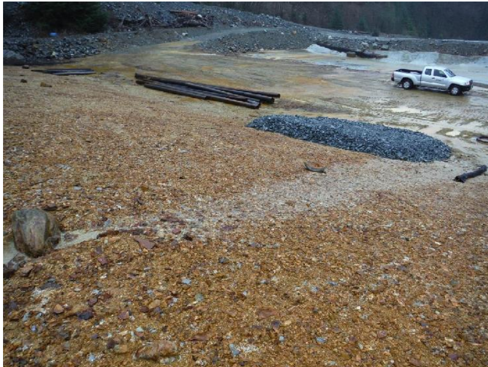
Photo 3 – Seepage from discrete source along the east arm of the Paste Berm (photo taken on 2014-11-27).
