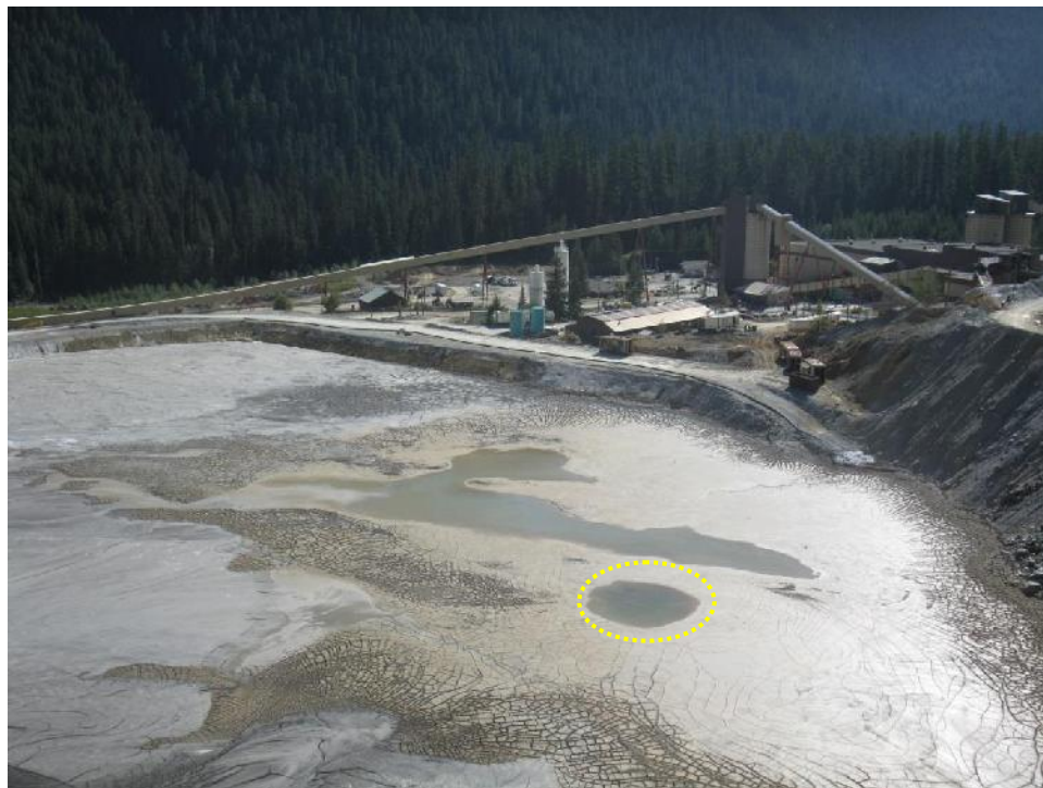
Photo 16 – Overview of Lynx TDF, looking southwest (recurrent depression in paste surface clearly visible, marked by dotted circle).
