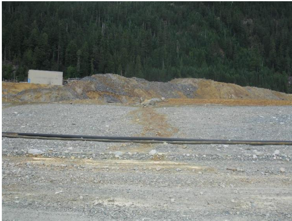
Photo 7 – ARD staining on the Seismic Upgrade 6:1 Slope and main bench below the access road at the west end of the Strip, looking north.
