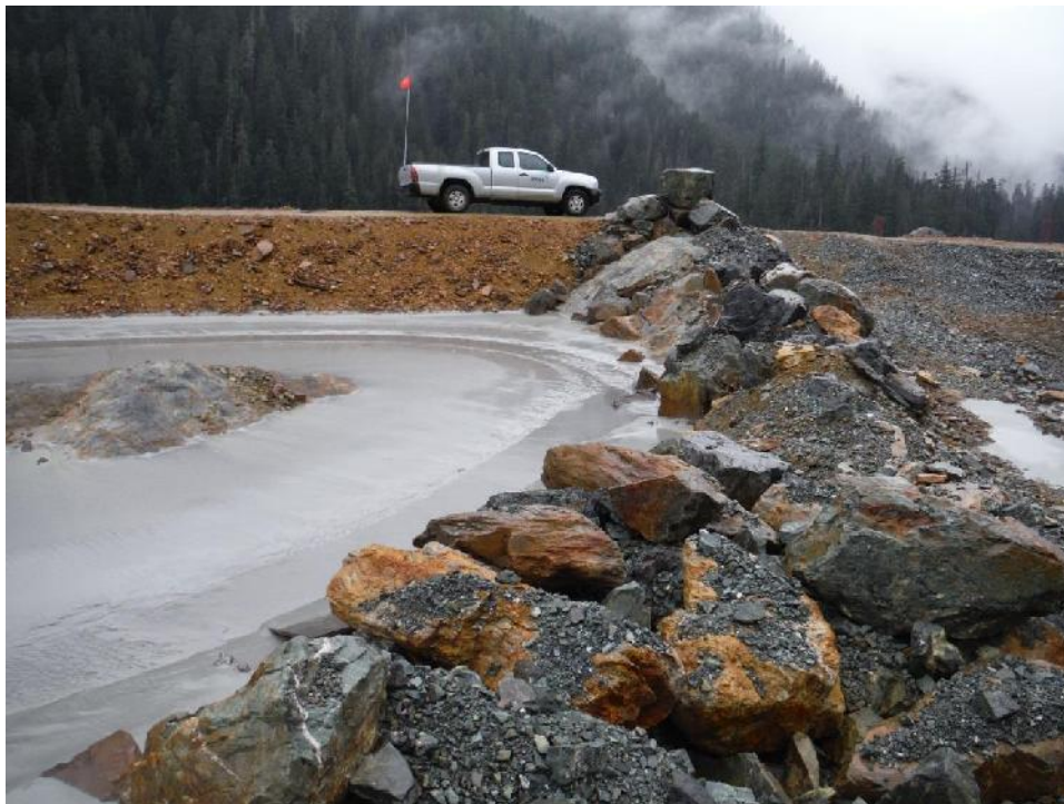
Photo 6 – Tailings slurry flowing through rocks at the APA decant, looking southwest (ramp leading to the decant structure immediately to the right of the photo)
