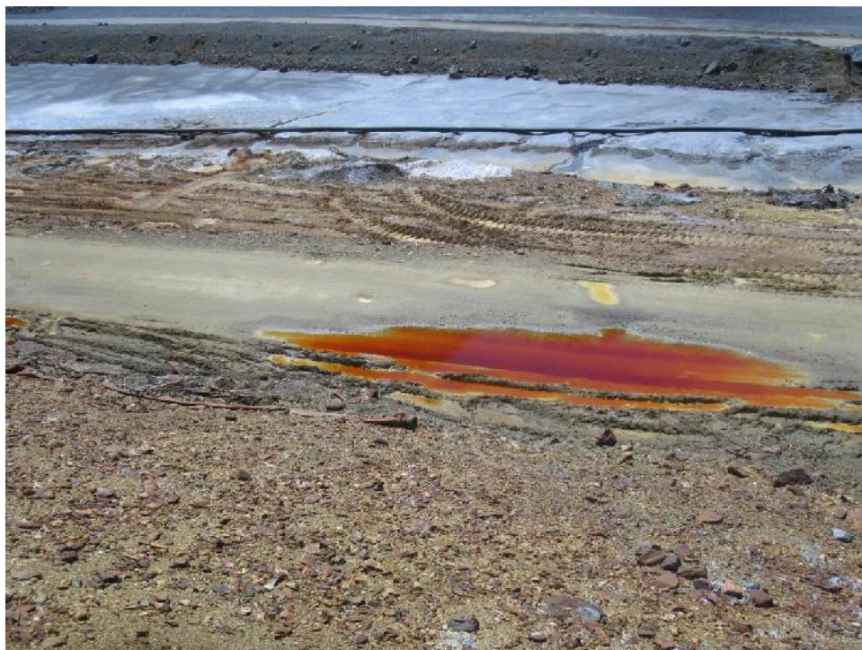
Photo 10 – ARD seepage at the toe of the Paste Berm near the Strip decant location (Strip decant is to the right).
