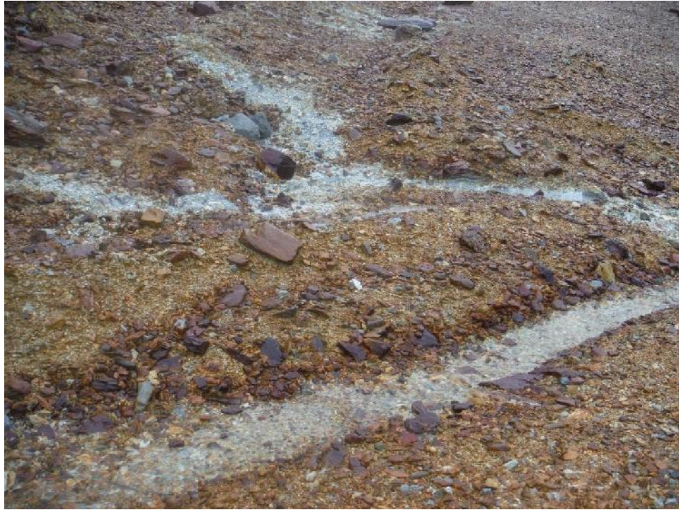
Photo 13 – Seepage areas at the base of the Paste Berm, Old TDF East Strip.
