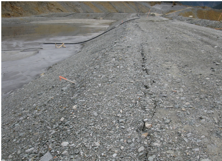
Photo 18: Crack along the upstream side of Lynx Dam south arm, looking east (March 5, 2015).
