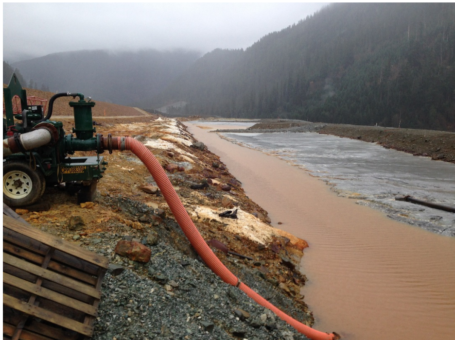
Photo 40: View of West Strip from the decant area, looking east. Note presence of pump to manage water levels (October 30, 2015).
