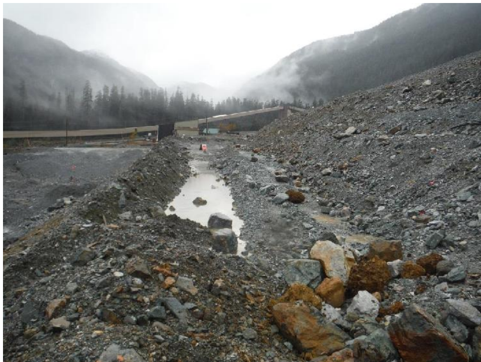
Photo 32 – Seepage and ponding on Lynx Dam “2011 Bench”, near Instrument Plane F, looking west.
