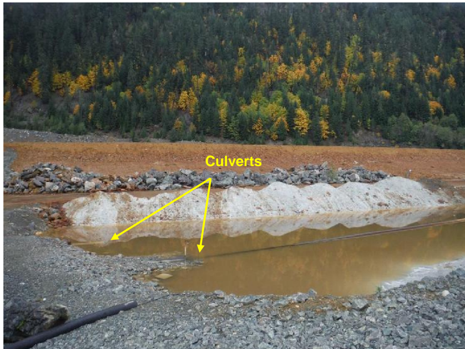
Photo 13 – Lime piles along the west end of the East Strip, looking north. Water level is above the intake of the two culverts passing under the Old TDF spillway.
