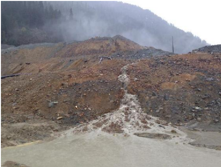
Photo 32 – Uncontrolled surface runoff coming from haul roads into Superpond outlet area.
