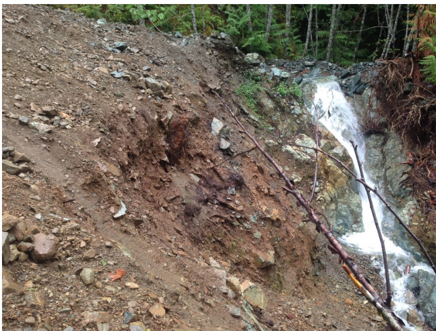
Photo 51: Erosion of slope at the east end of Upper Lynx Diversion Ditch near Cascade Reach (Taken September 24, 2015).
