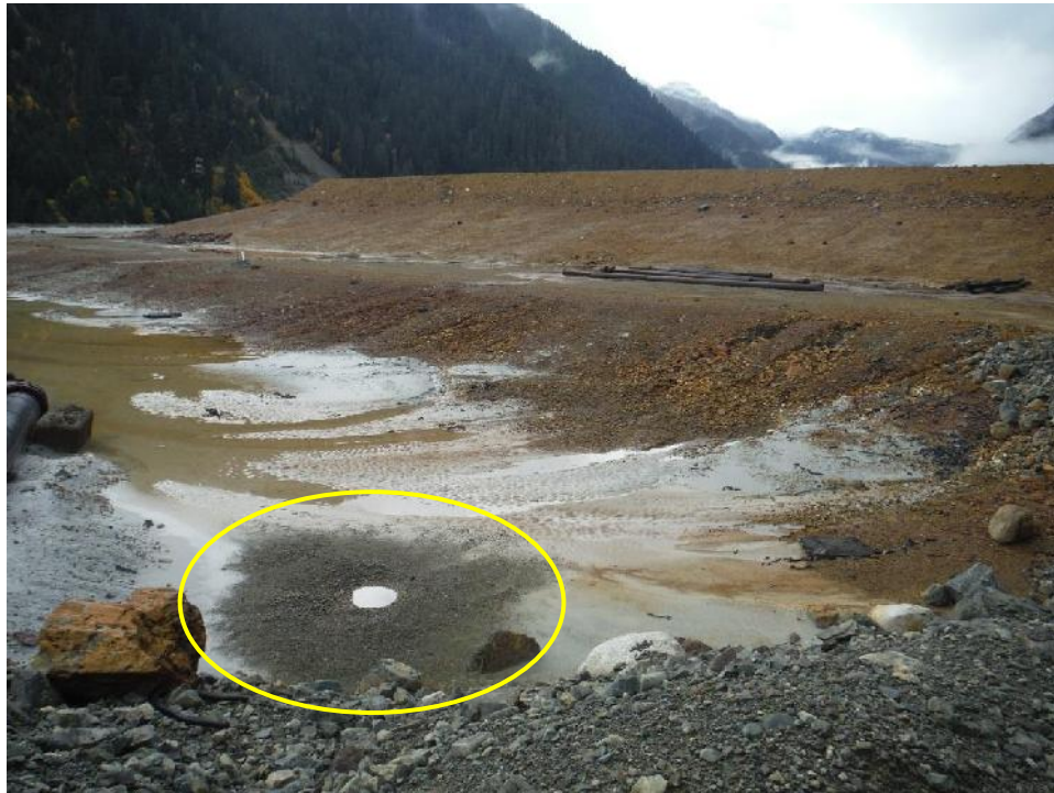
Photo 9 – North end of the East Strip, looking south/southwest. A water boil area formed a cone of coarse sand around the “vent”.
