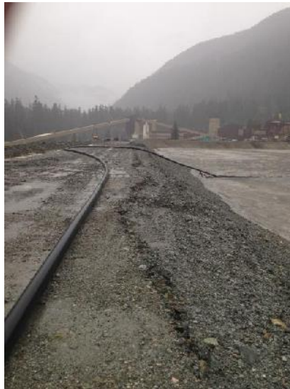
Photo 27 (left) – Trench in upstream half of Lynx Dam crest to route piezometer wires. Photo 28 (right) – Cracking at the contact of the Zone J core and the upstream dam shell.
