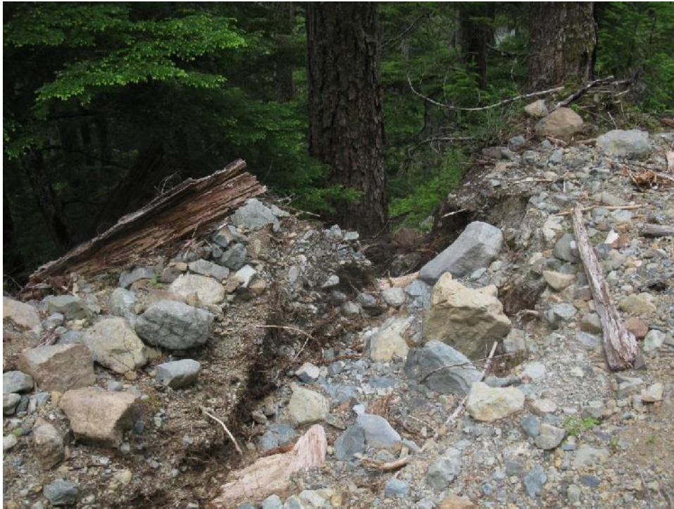
Photo 27 – Breach of lower Arnica diversion ditch near the lower end.
