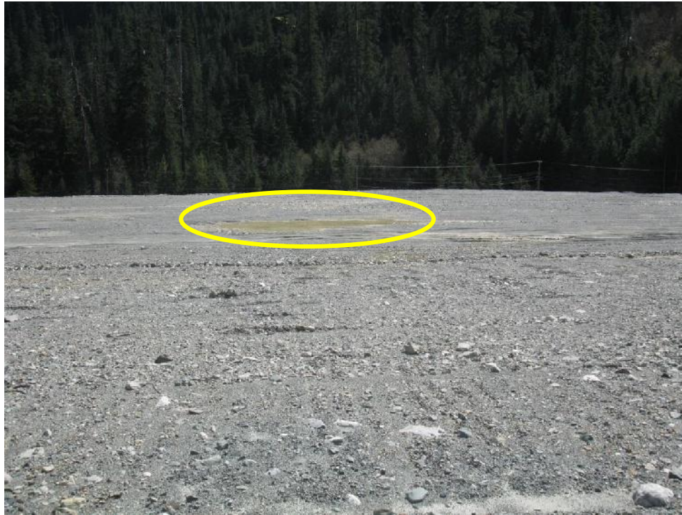
Photo 11 – ARD puddle at toe of 6:1 Slope near Instrument Plane C, looking south.
