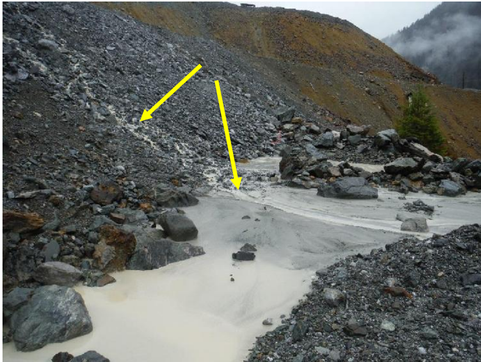
Photo 29 – Runoff on the side of A-Ramp embankment carrying sediments down to dam toe in Phillips Sump area.
