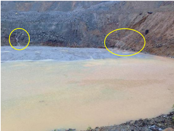
Photo 34 – Eastern area of Lynx Dam foundation panels flooded, looking north (seeps circled).
