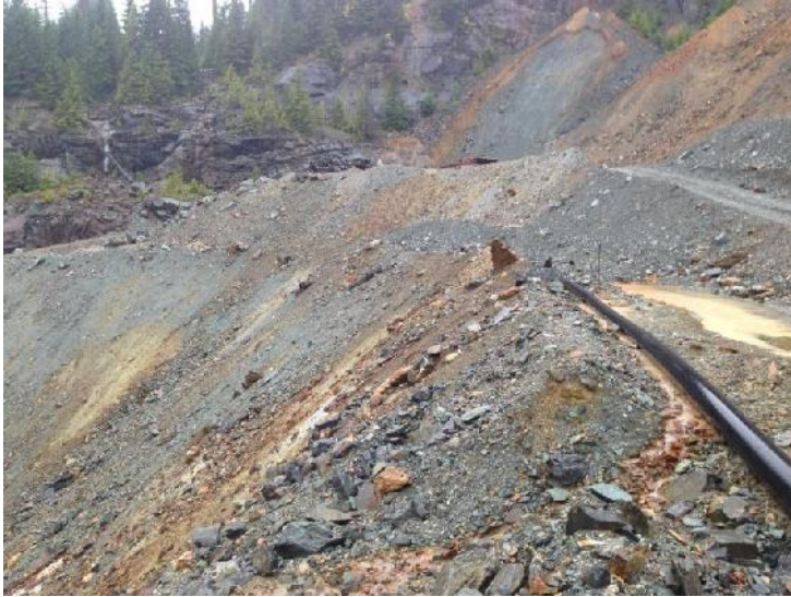
Photo 25 – Seepage at the toe of Lynx Pit slide area, looking west.
