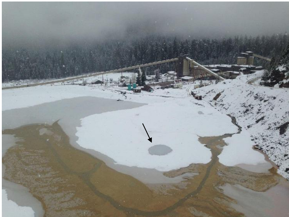
Photo 2 – Lynx TDF, looking southwest. The recurrent depression is visible in the edge of the mud wave, at the arrow.
