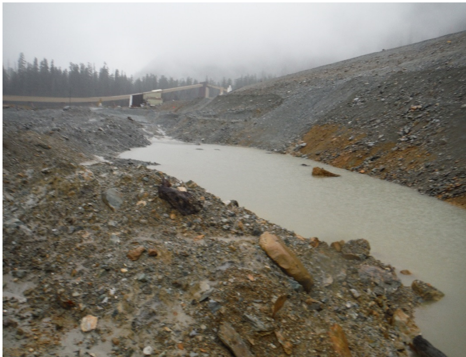
Photo 10: Flooding at toe of Lynx Dam, looking west (December 10, 2014).
