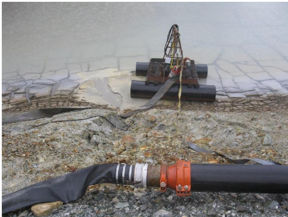
Photo 20 – Electric pump and pump line at the Lynx TDF west arm.
