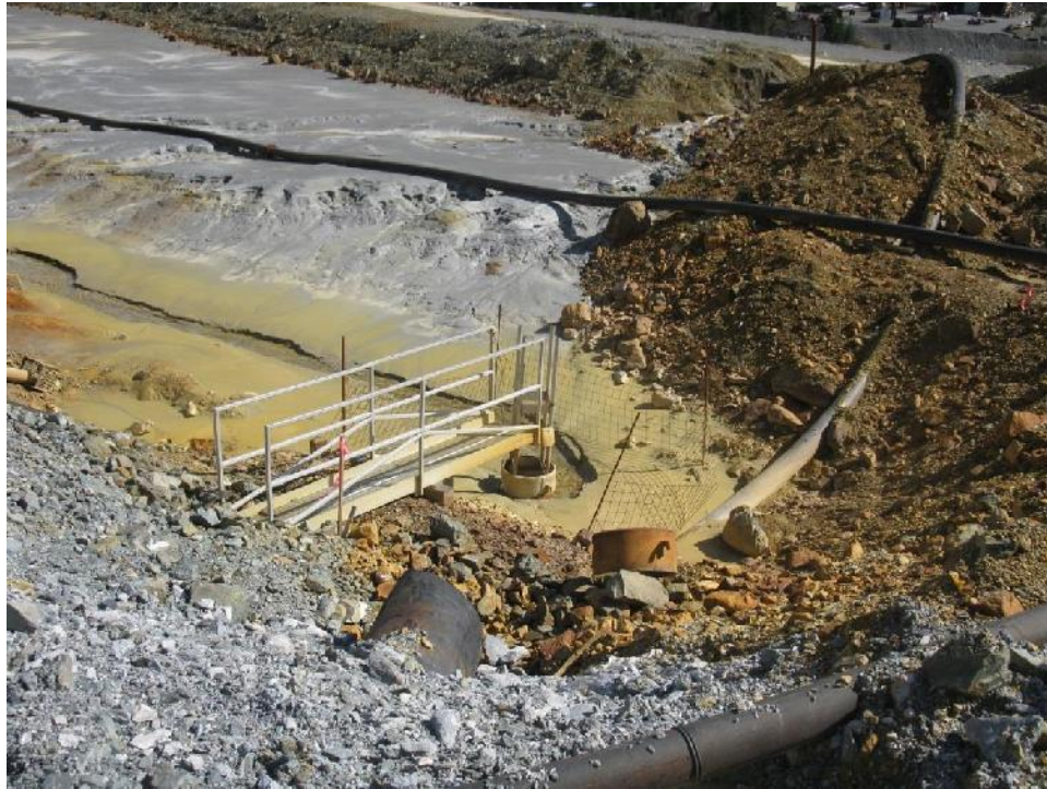
Photo 9 – Strip decant and overflow spillway pipe.
