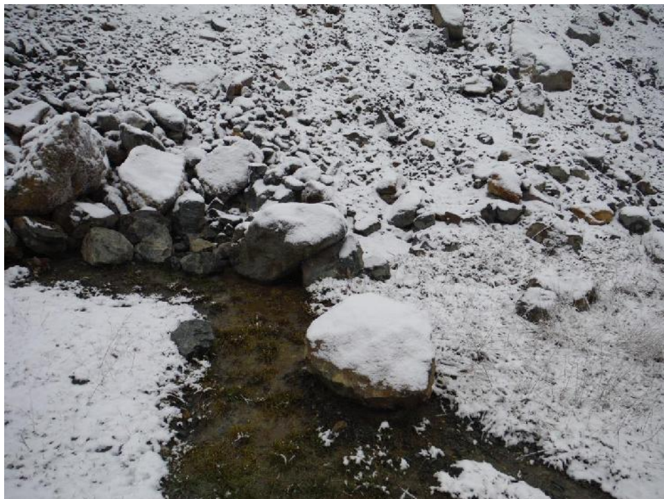
Photo 20 – Some seepage on the mid-level “2011 Bench” of Lynx Dam south arm.
