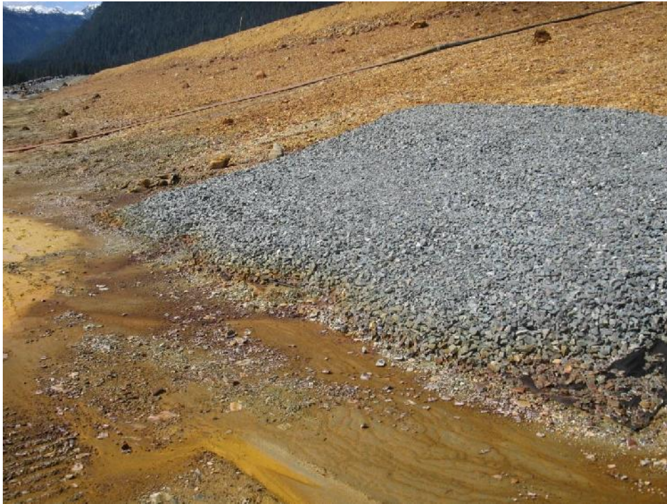
Photo 5 – ARD seepage at the base of the Paste Berm near Instrument Plane C, showing one of the clean rock pads built to prevent piping erosion.
