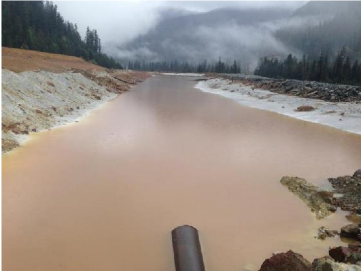
Photo 11 – Ponded water in the East Strip, looking east from the Old TDF spillway (the inlet of one of the culverts passing under the spillway located in the foreground).
