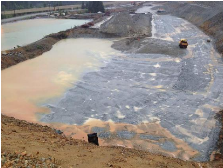
Photo 33 – South/east area of Lynx Dam foundation panels flooded.
