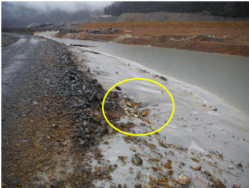
Photo 12 – East Strip, looking west from central area (yellow circle showing sinkhole into the OEB sand beach).
