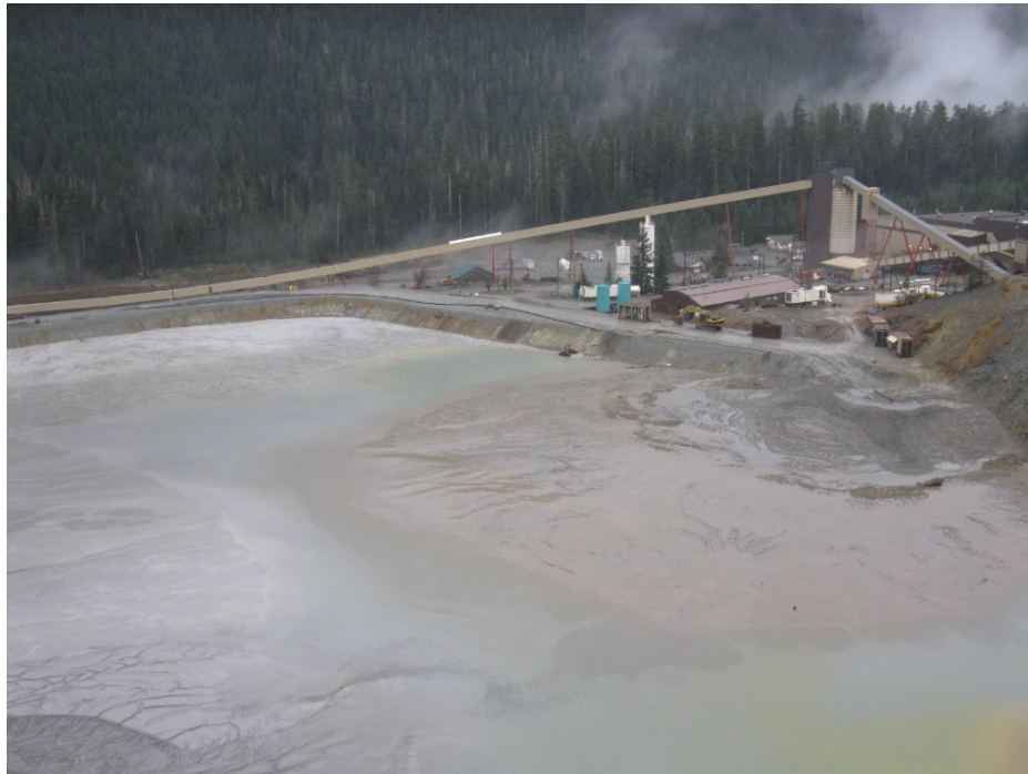
Photo 23: View of Lynx TDF, looking southwest. Note mud wave in tailings created by construction waste deposition in the northwest corner (October 31, 2015).
