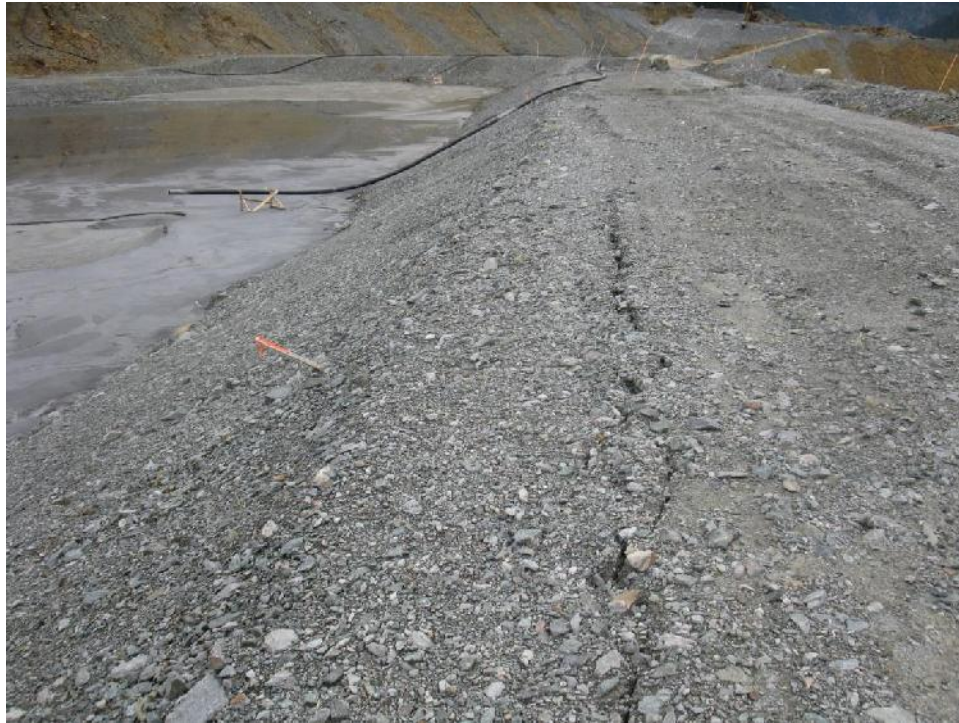
Photo 17 – Crack along the upstream crest of Lynx Dam south arm, looking east.
