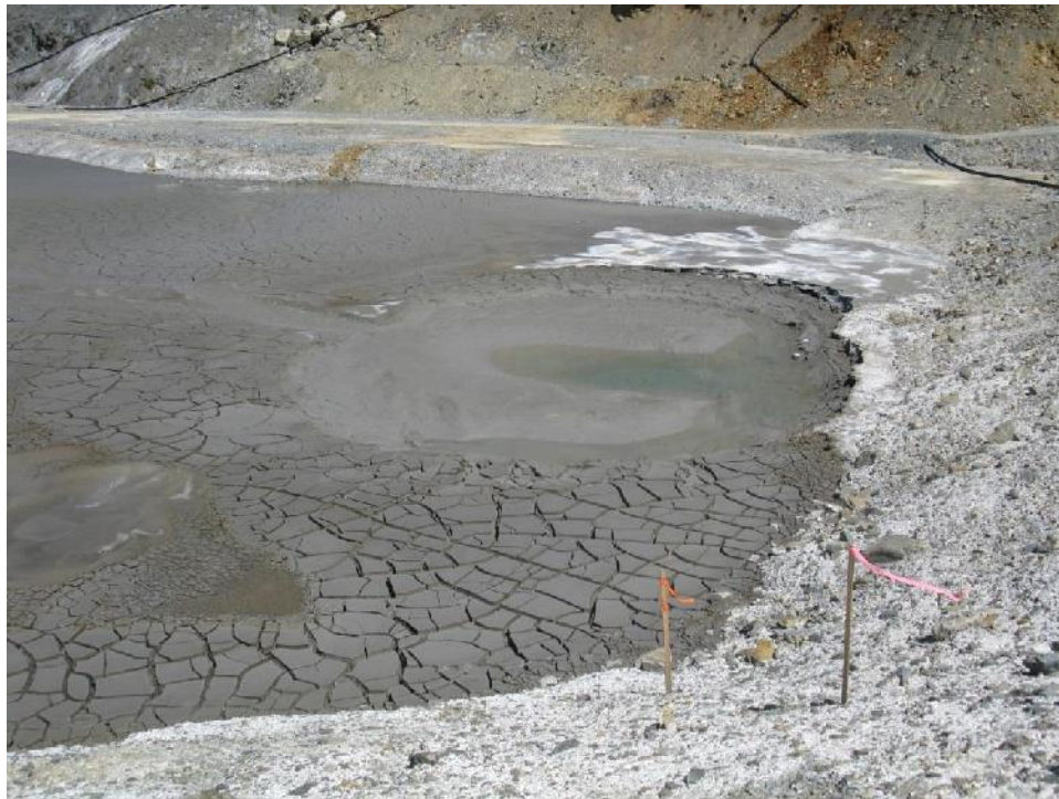
Photo 19 – Desiccation cracking on the paste surface at the east end of Lynx TDF, looking north.
