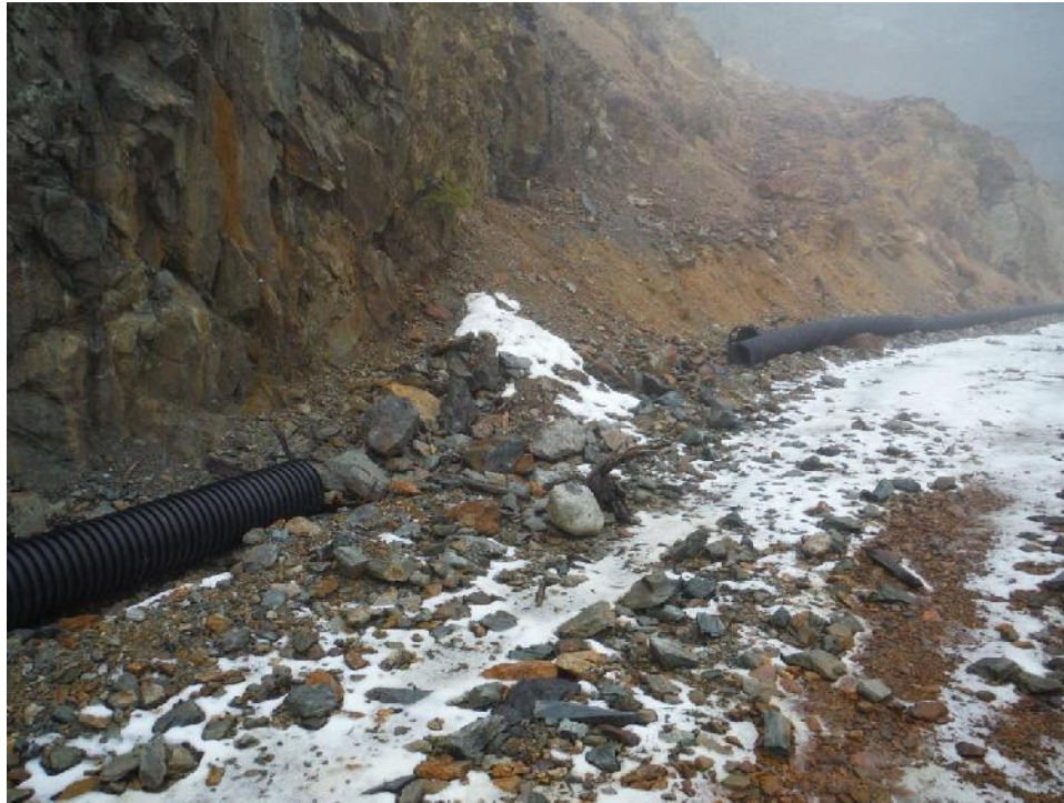
Photo 23 – Torn drainage pipe along water diversion just above Lynx Pit Slide area.
