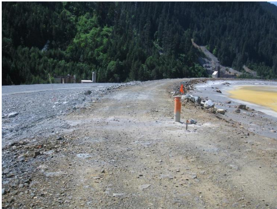
Photo 6 – Piezometer datalogger enclosure on the OEB road, looking south/southwest. This enclosure needs to be moved to the left of the road, down the 6:1 slope.
