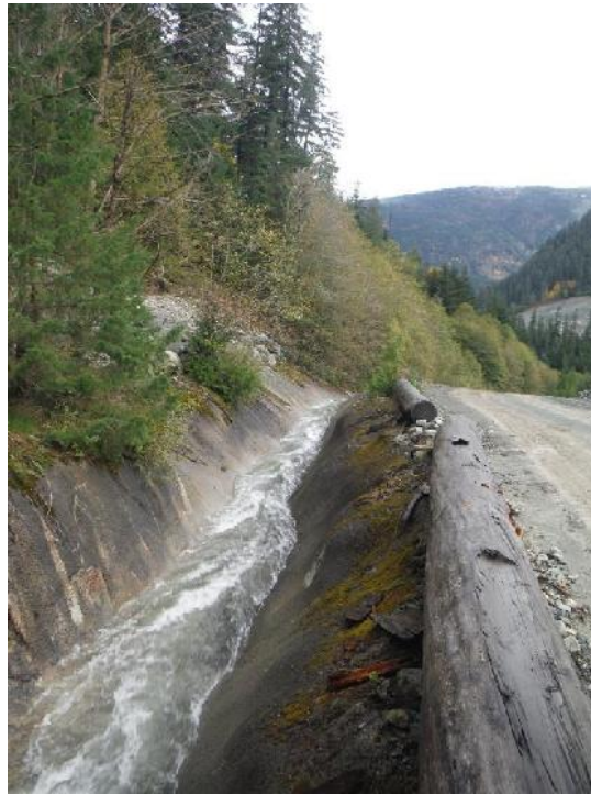
Photo 23 – Lined section of Lower Lynx Diversion Ditch near the Paste Berm east abutment.
