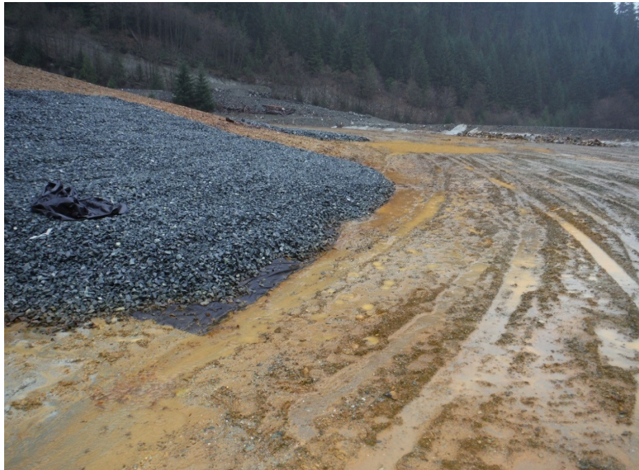
Photo 6: Patching work completed for the piping erosion at the Paste Berm toe, constructed using geotextile filter fabric and free draining material, looking northeast (November 27, 2014).
