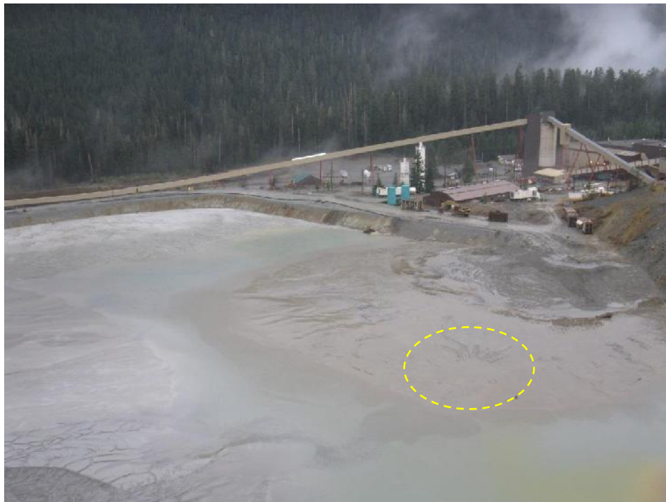
Photo 18 – Overview of the west part of Lynx TDF, looking southwest. The circled area corresponds to the location of the recurrent depression on the tailings surface.
