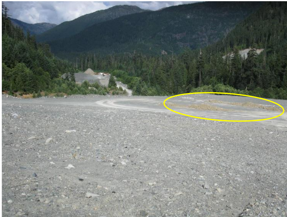
Photo 9 – East abutment of the Seismic Upgrade Berm, looking east towards the on-site Quarry. Piles of PAG mine waste are circled.
