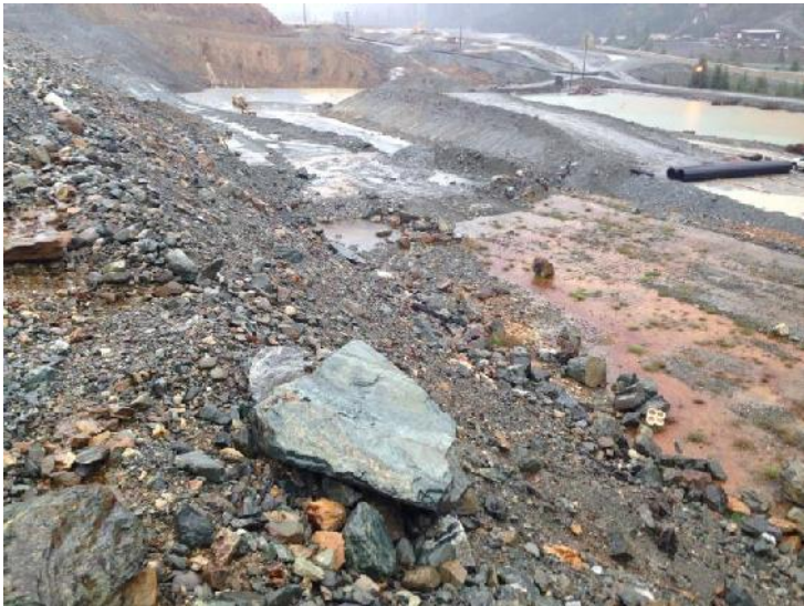
Photo 36 – Seepage and surface runoff on Lynx Dam mid-level bench (in foreground) and Lynx Dam foundation panels area, Zone J stockpile and Super Pond (in background), looking southeast.
