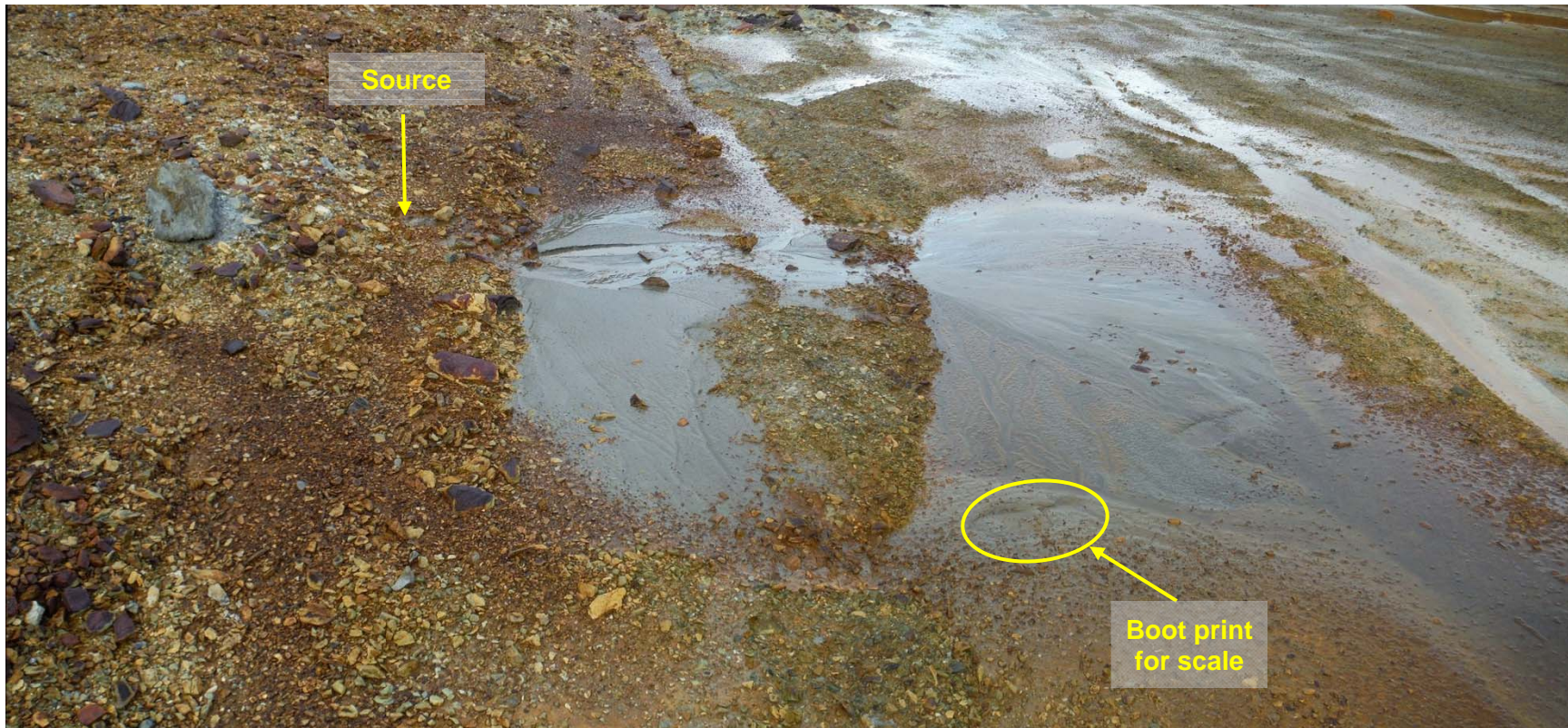
Photo 3 – Side view of piping area looking northwest along the toe of the Paste Berm.
