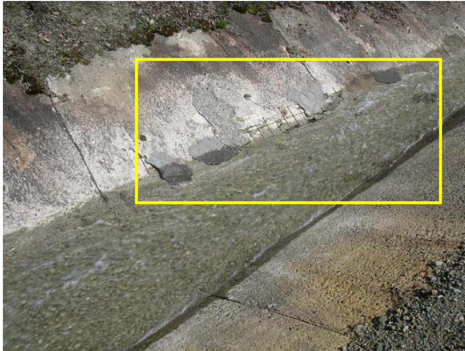
Photo 17 – Patches, exposed rebar and holes in Lower Lynx Diversion Ditch shotcrete liner.
