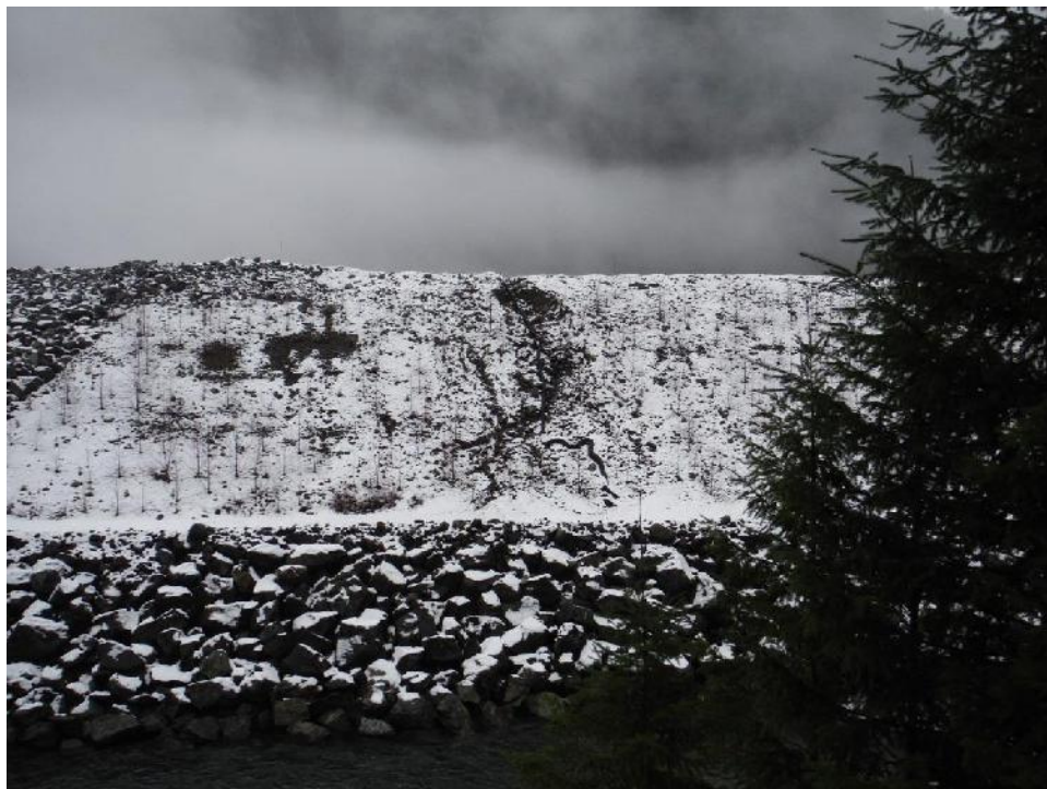
Photo 12 – New erosion gully into the Seismic Berm downstream face, just east of the Old TDF spillway.
