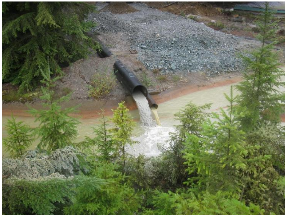
Photo 14 – Turbid water coming out of the APA (large diameter) and the RSA (small diameter) decant lines.
