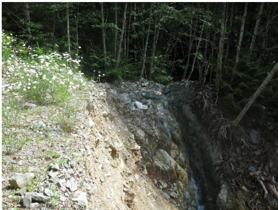
Photo 30 – Headscarp of failure at switchback at lower end of Upper Lynx Diversion. Diversion formerly flowed left to right to the edge of the photo, now captured by the headscarp.
