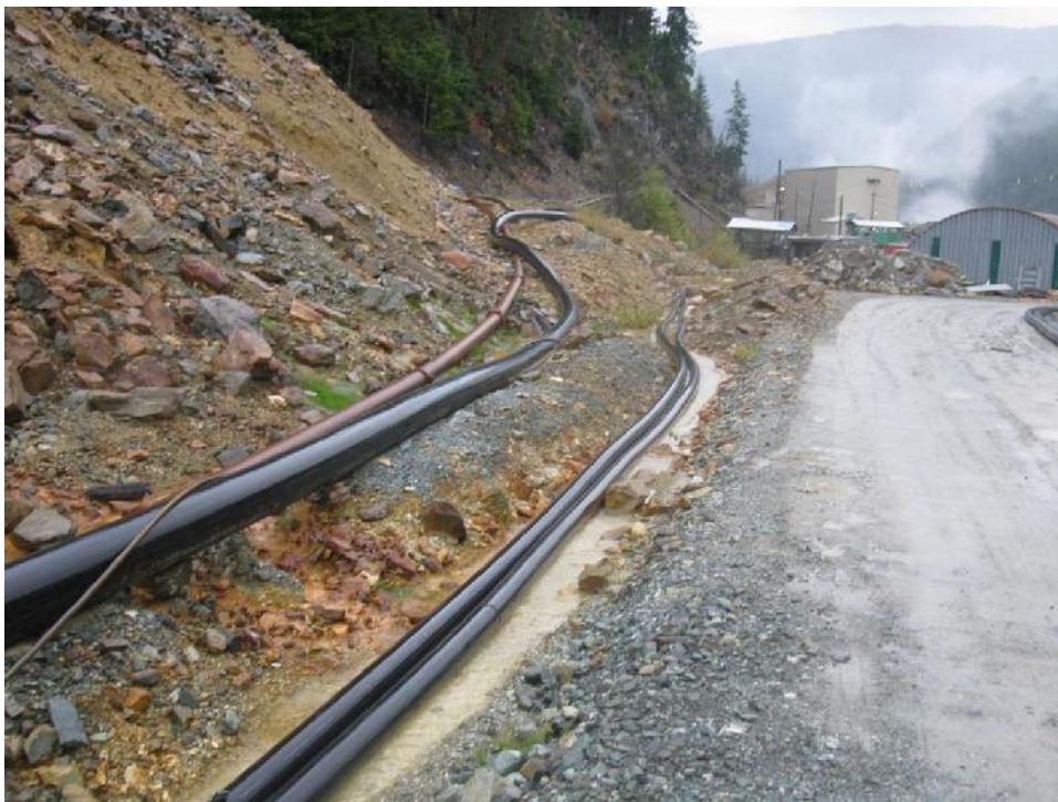
Photo 26 – Seepage and surface runoff collection along the access road at the back of Lynx TDF, looking east. Flow is collected near the Paste Plant (in the background).
