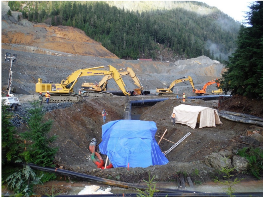
Photo 55: Decant pipeline leading to energy dissipater (December 15, 2015).
