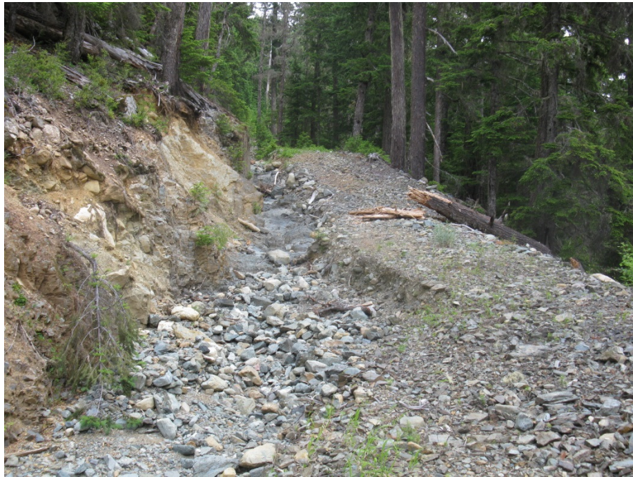
Photo 46: Lower Arnica Reach Ditch, looking upstream. Note side erosion to the right due to high water levels (June 17, 2015).
