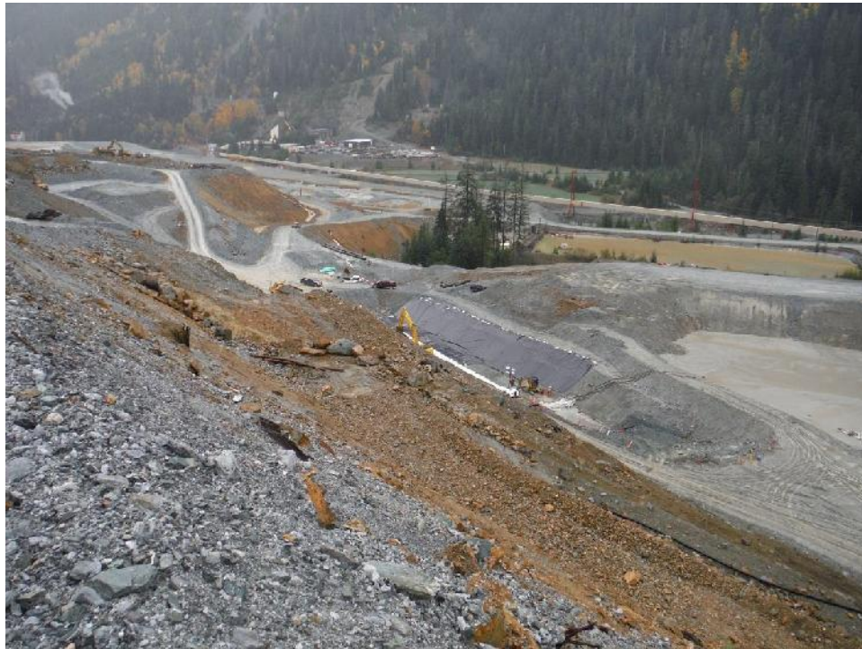
Photo 27 – Section of Lynx Springs Drain going through Lynx Dam east arm under construction, looking east/southeast.
