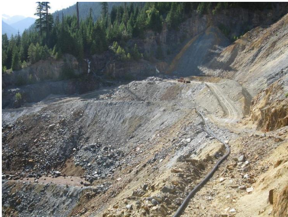
Photo 20 – Lynx Pit slide area, looking west. Berm has been constructed and road access has been restored through the top of the waste dump area.
