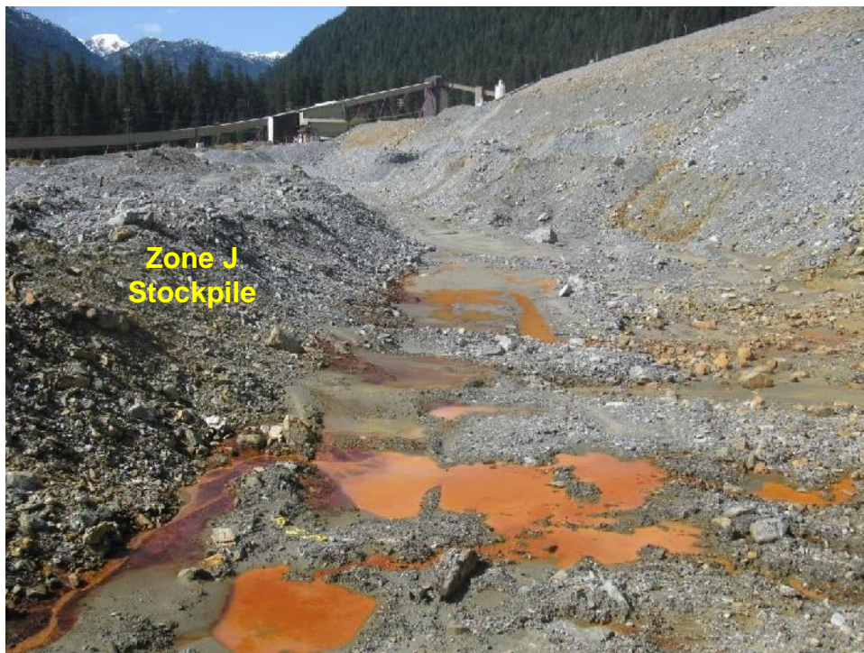
Photo 24 – East portion of Lynx dam south arm toe area with ARD water accumulation (most seepage coming from the “Zone J” material stockpile), looking west.
