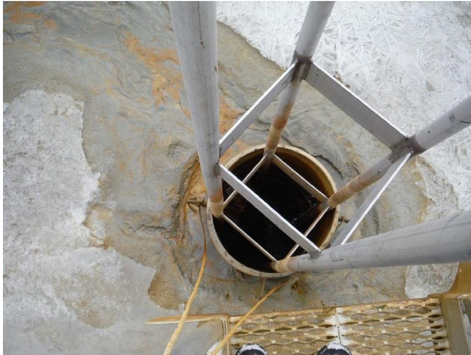
Photo 7 – Top view of Strip decant structure with ice around it.
