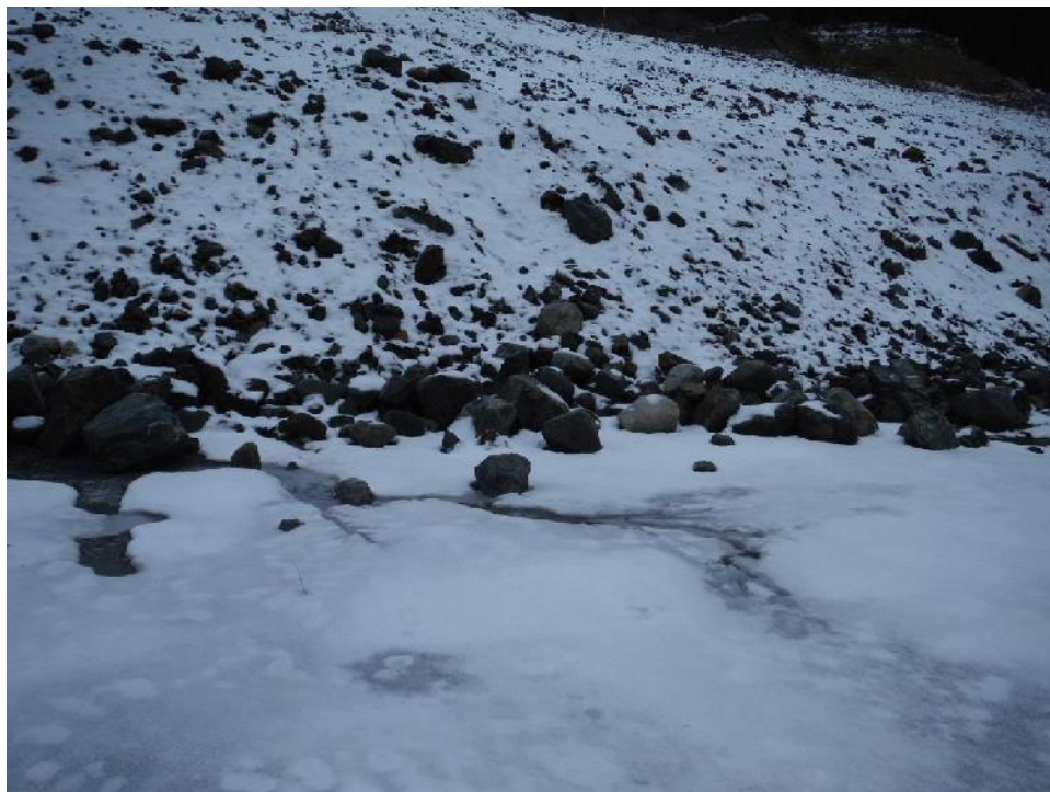
Photo 20 – Seepage flow on Lynx Dam lower bench near east end.
