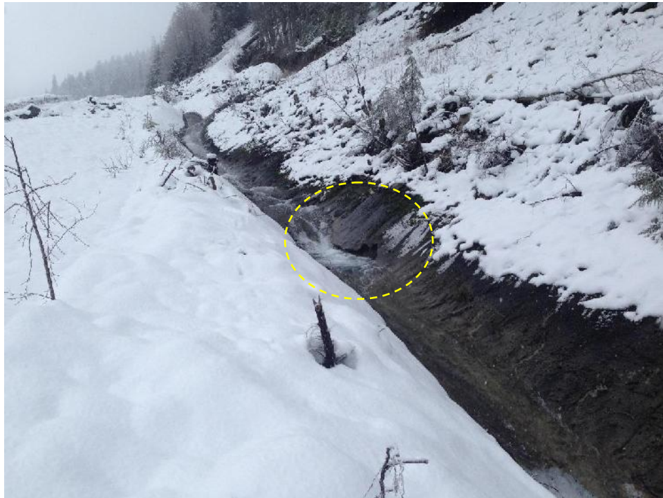
Photo 19 – Damaged section of the Lower Lynx Diversion Ditch shotcrete lining.
