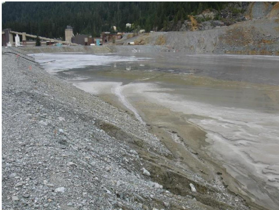
Photo 18 – Minor sloughing of Lynx Dam upstream face of south arm, looking west.
