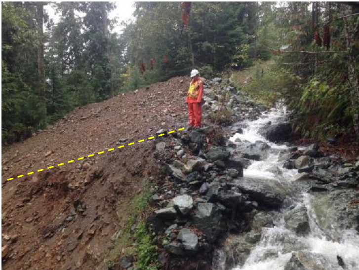
Photo 41 – Re-graded slope and remaining steep slope (above/below dashed line) at the slide area at the east end of the Upper Lynx Diversion Ditch. Additional pullback is recommended.
