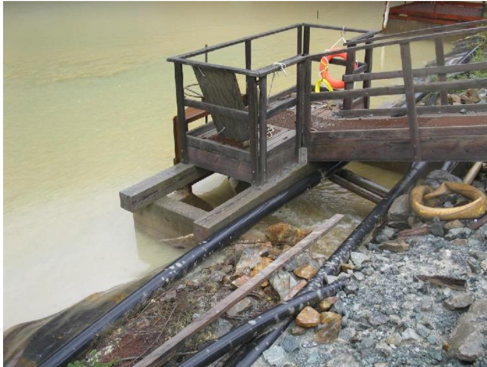
Photo 15 – Turbid water entering the Super Pond outlet.
