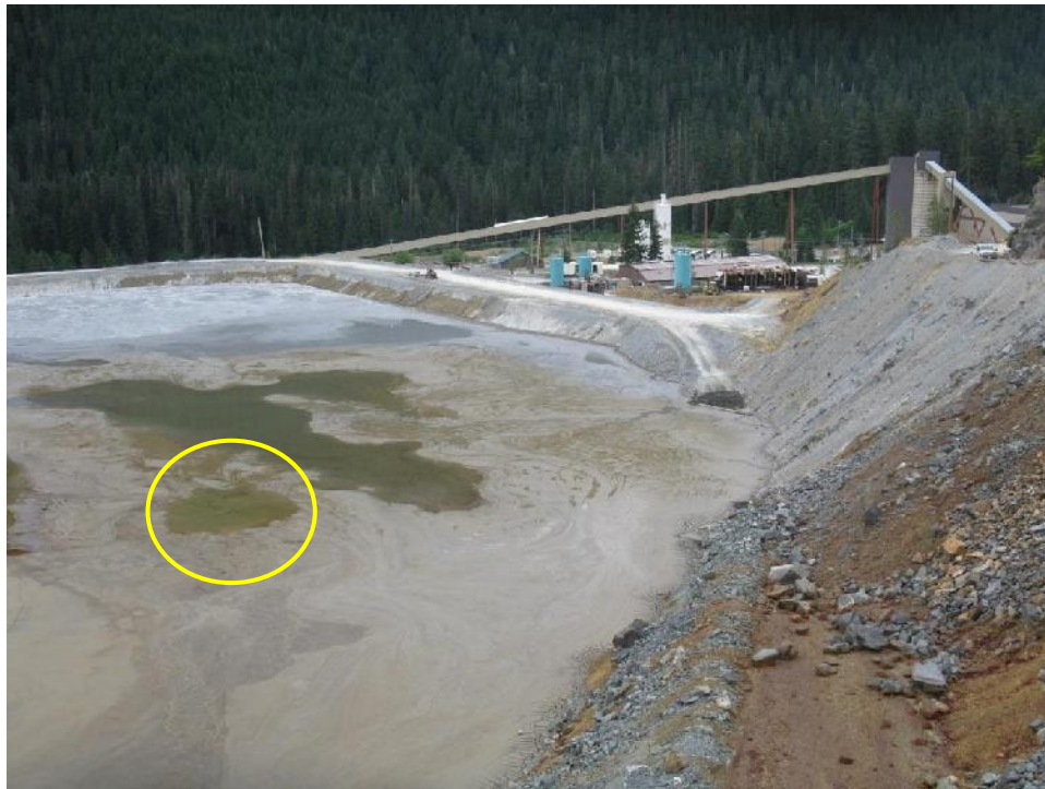
Photo 13 – Lynx TDF, looking southwest. No pumps at the bottom of the ramp (circle shows the location of the recurrent depression).
