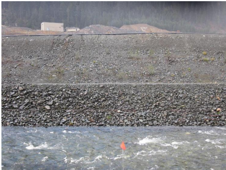
Photo 16 – Minor erosion rills on the 2:1 slope of the Seismic Upgrade Berm at approximately Station 0+200, looking north..
