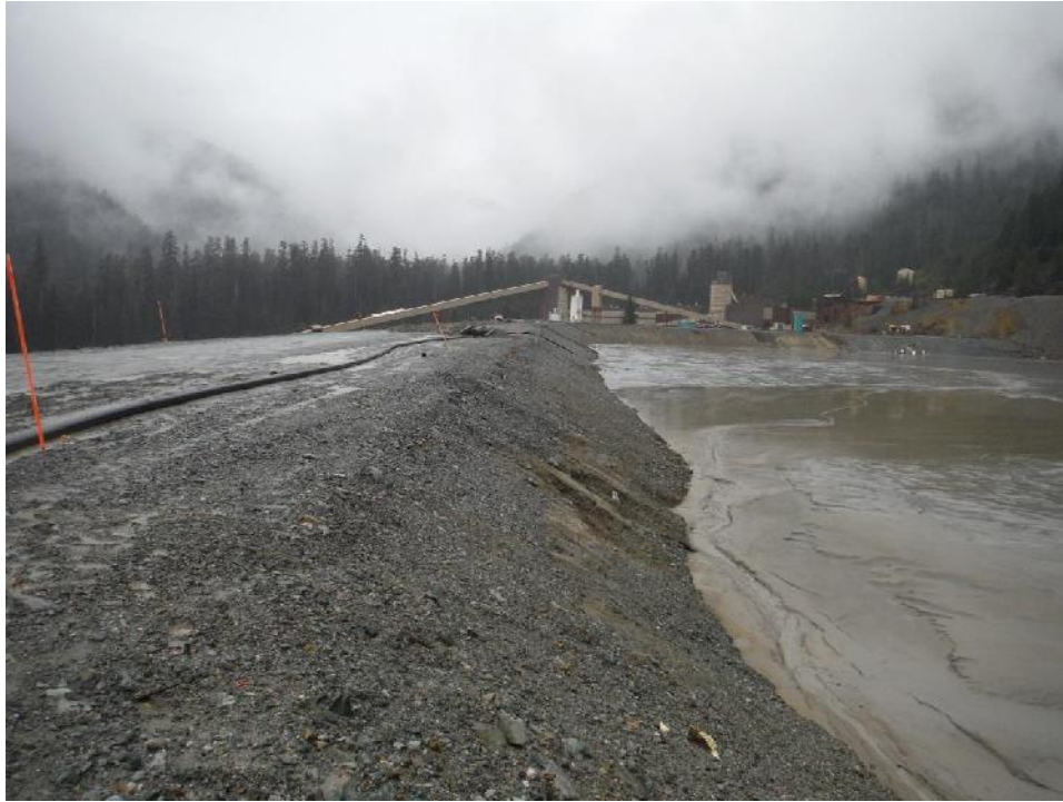
Photo 25 – South arm of Lynx Dam near the east end of the facility showing minor sloughing on upstream face, looking west.
