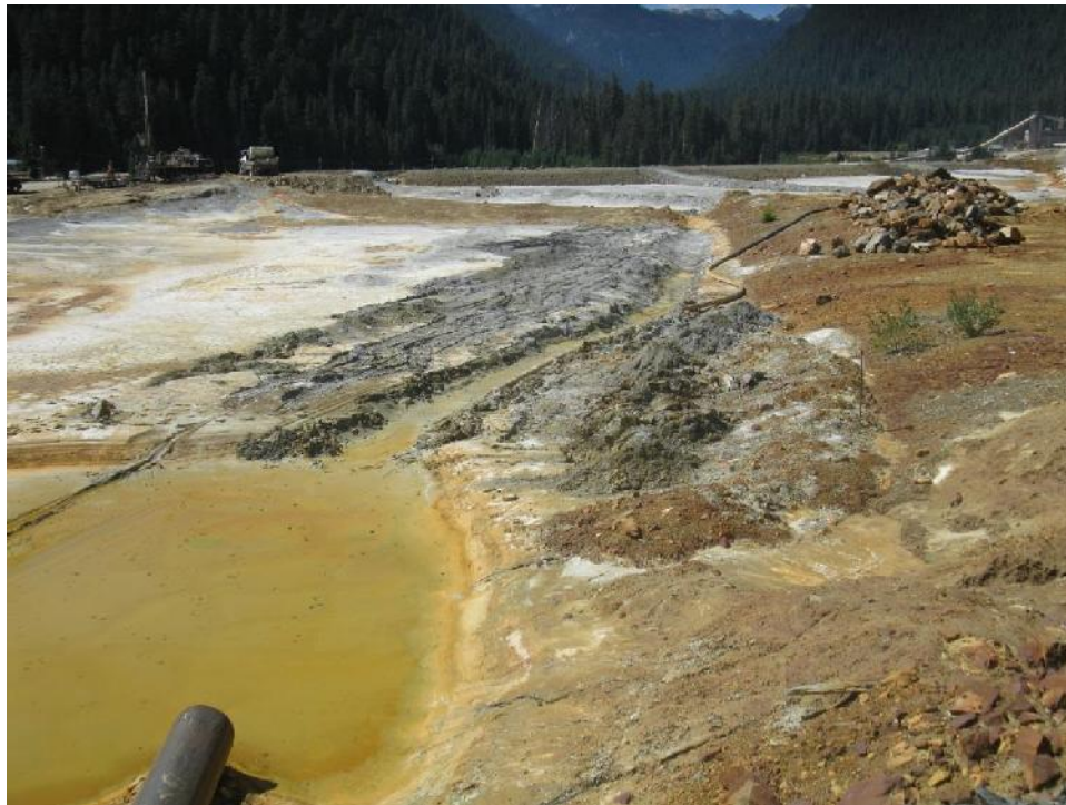
Photo 5 – West Strip looking west from the Old TDF spillway. Ditching to relieve water from excavation is in preparation for culvert clearing.
