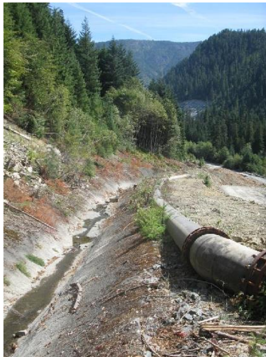
Photo 14 – Shotcrete-lined portion of Lower Lynx Diversion Ditch near Alder Reach Ditch, looking east.
