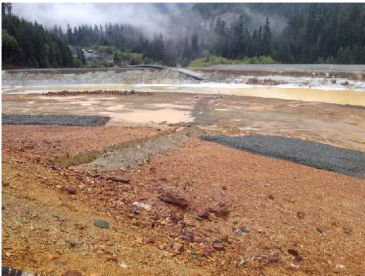
Photo 8 – Pounded water at the base of the Paste Berm between two rock pads (in foreground), ponded water in the East Strip (in background), looking near Instrument Plane C.
