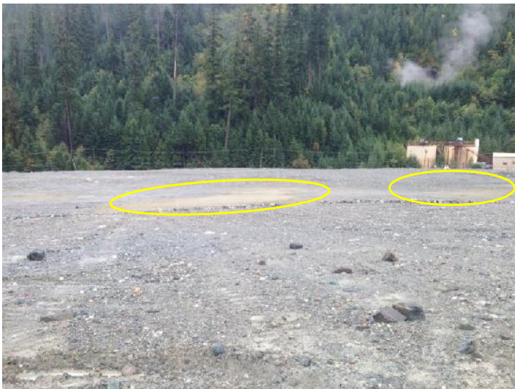
Photo 16 – Puddles at the toe of the 6:1 Slope along the Seismic Upgrade Berm main bench, east of the Old TDF spillway, looking towards the Backfill Plant.
