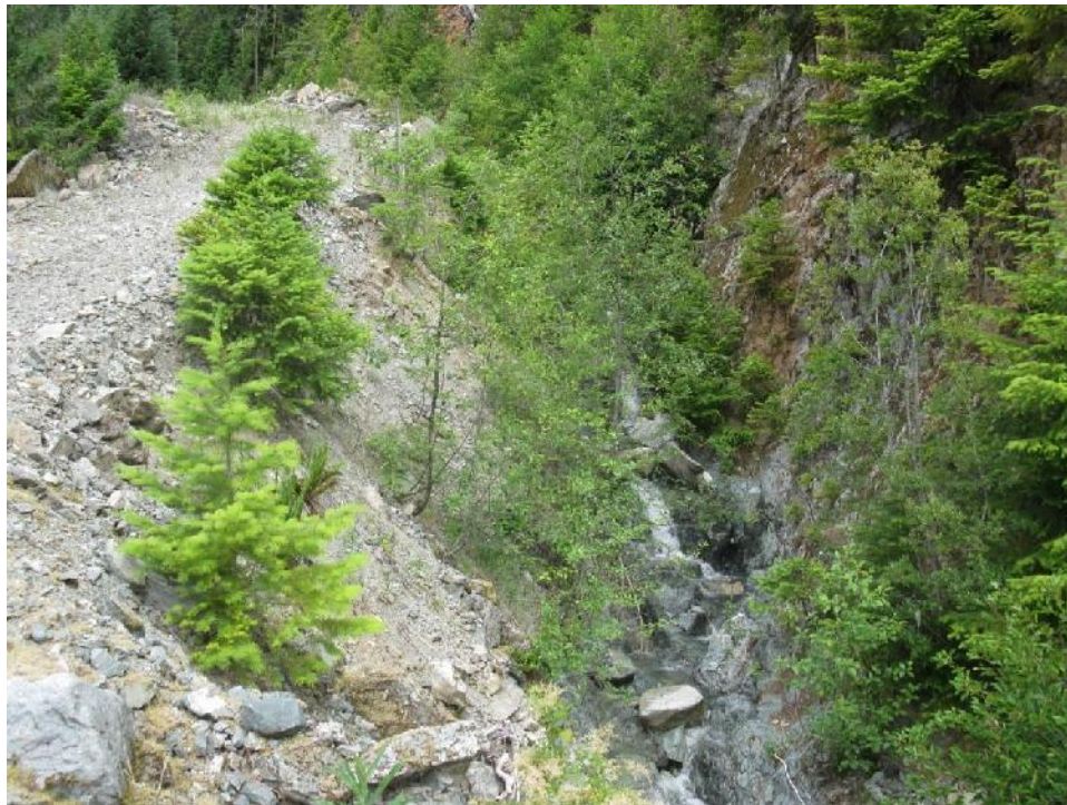
Photo 29 – Brush in Lynx Upper Diversion Ditch, looking upstream.
