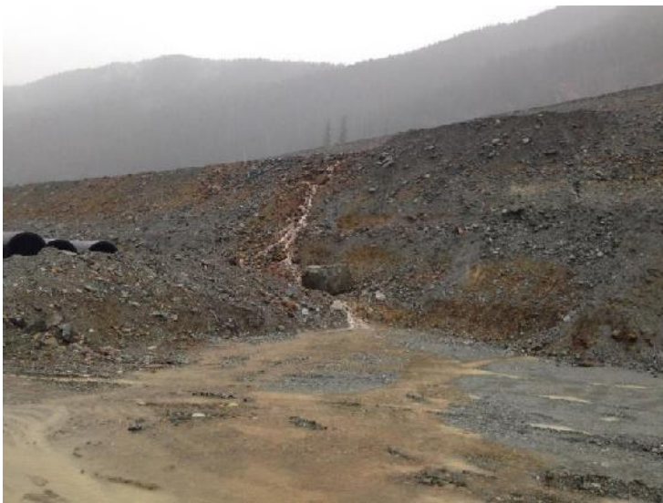
Photo 35 – Surface runoff flowing down the slope of the mid-level bench of Lynx Dam, looking north/northwest.
