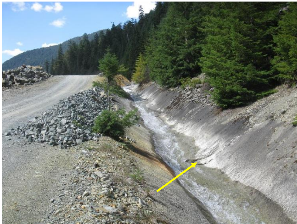
Photo 16 – Hole in Lower Lynx Diversion Ditch shotcrete liner.
