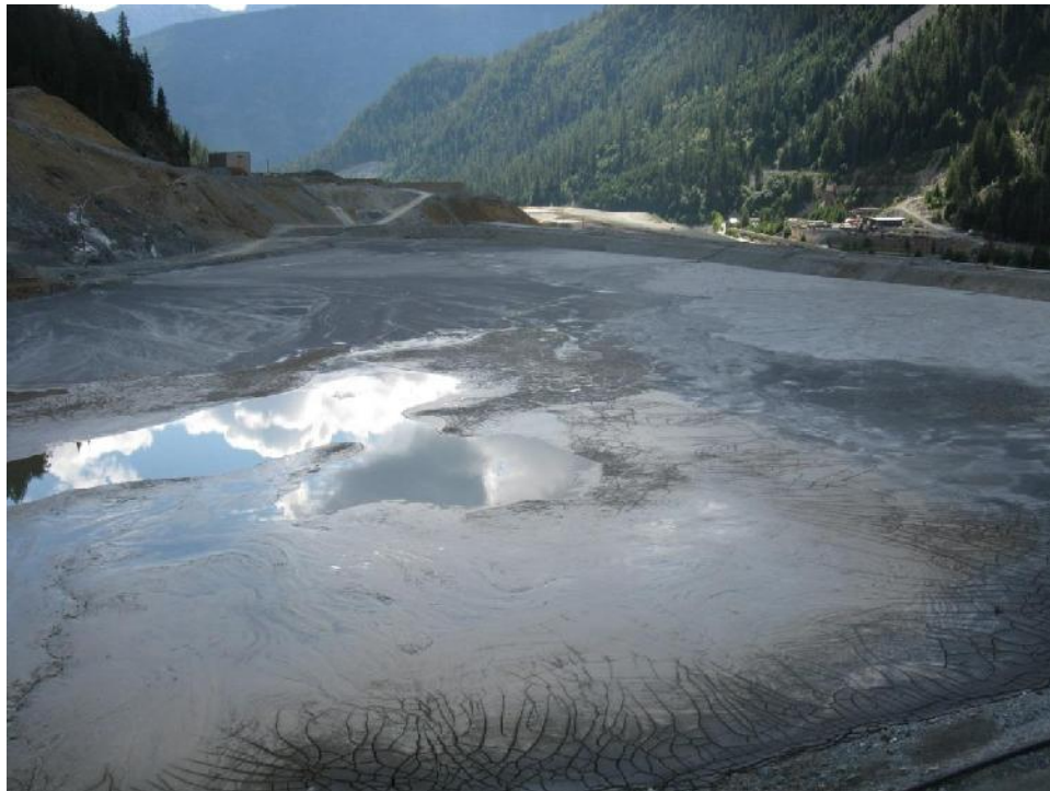
Photo 10 – Lynx TDF with desiccation cracking in fine tailings on exposed beach, looking east.
