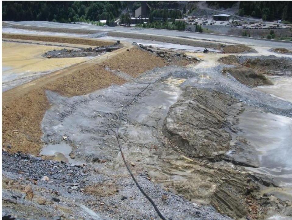
Photo 13 – West arm of the Paste Berm and east end of the RSA, looking south (note the variety of backfill materials onto the Paste Berm surface).
