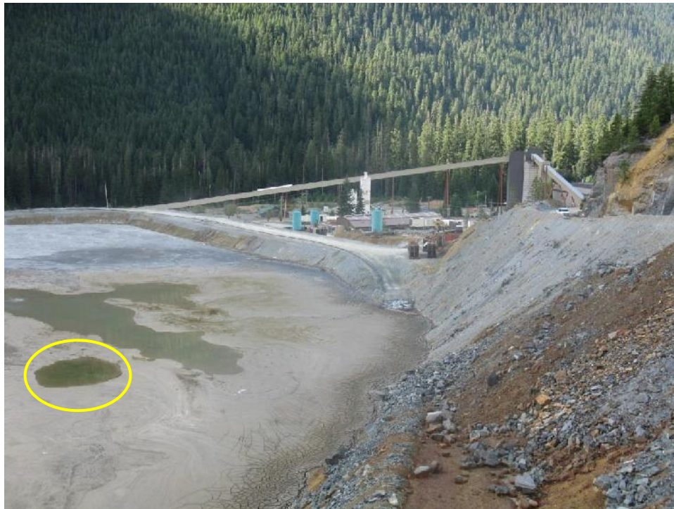
Photo 11 – Lynx TDF, looking southwest at the pump ramp area (no pumps, circled area showing the recurrent depression).
