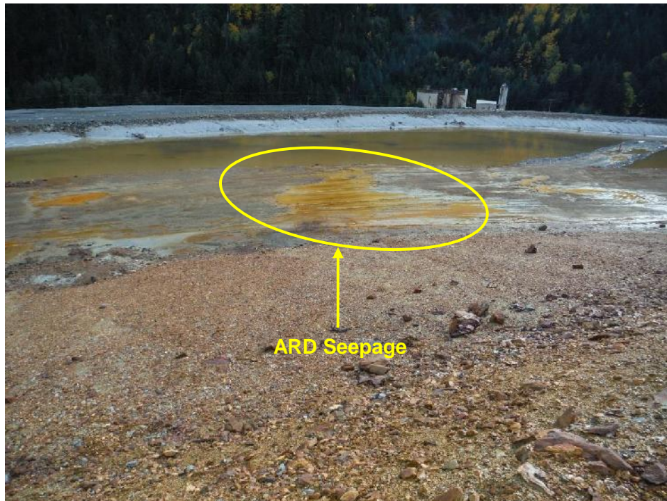
Photo 11 – Looking south down from the Paste Berm towards the Paste Backfill Plant. ARD seepage at the base of berm reporting to the East Strip.
