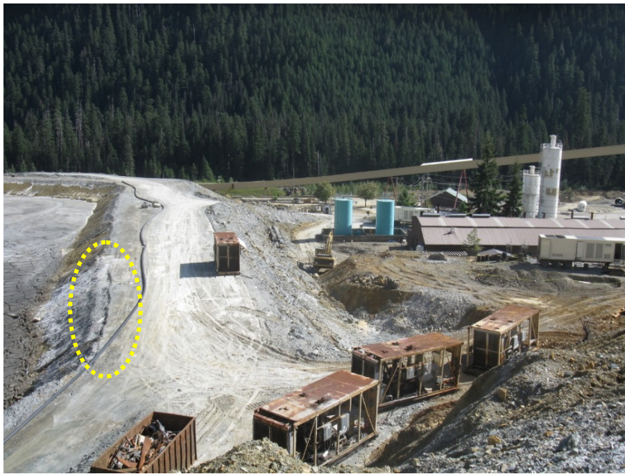
Photo 19: Lynx Dam west arm, looking south, showing minor sloughing of the upstream shell (August 24, 2015).
