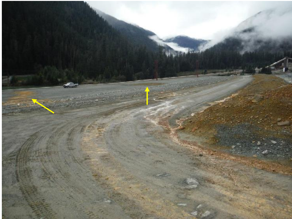
Photo 17 – Areas of ARD seepage on the Seismic Berm fed by runoff from the access road between the West Strip and the RSA, looking southwest.
