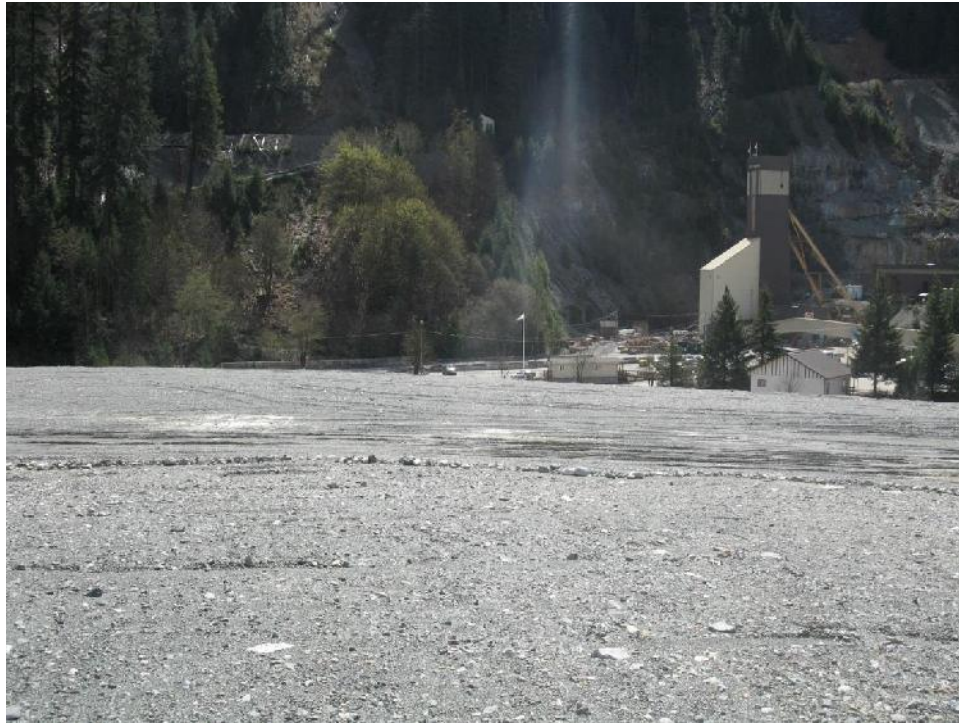
Photo 13 – Puddles and rutting on Seismic Berm ~ Sta. 0+700, looking south.
