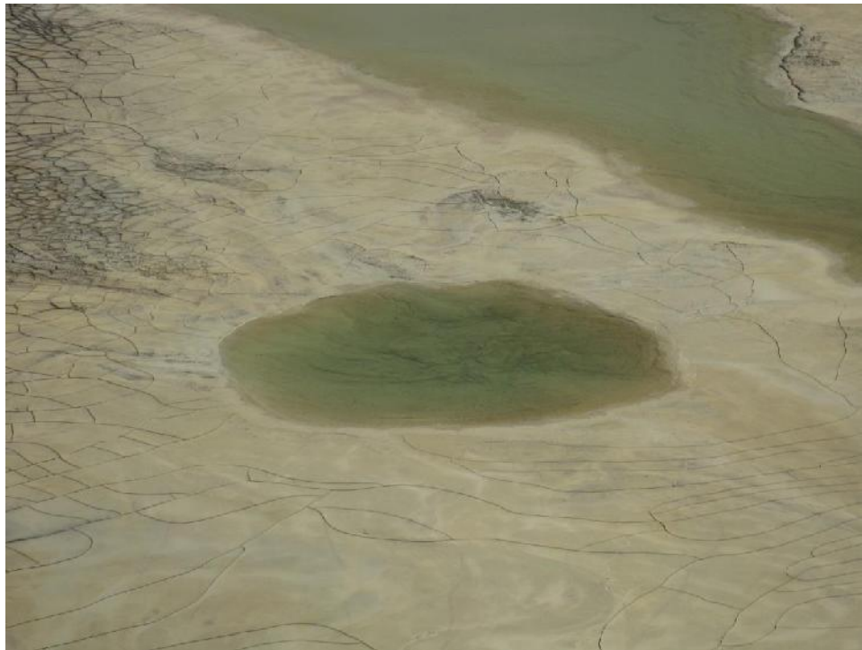
Photo 17 – Close-up view of the recurrent depression in Lynx TDF paste surface (see previous photo for location).
