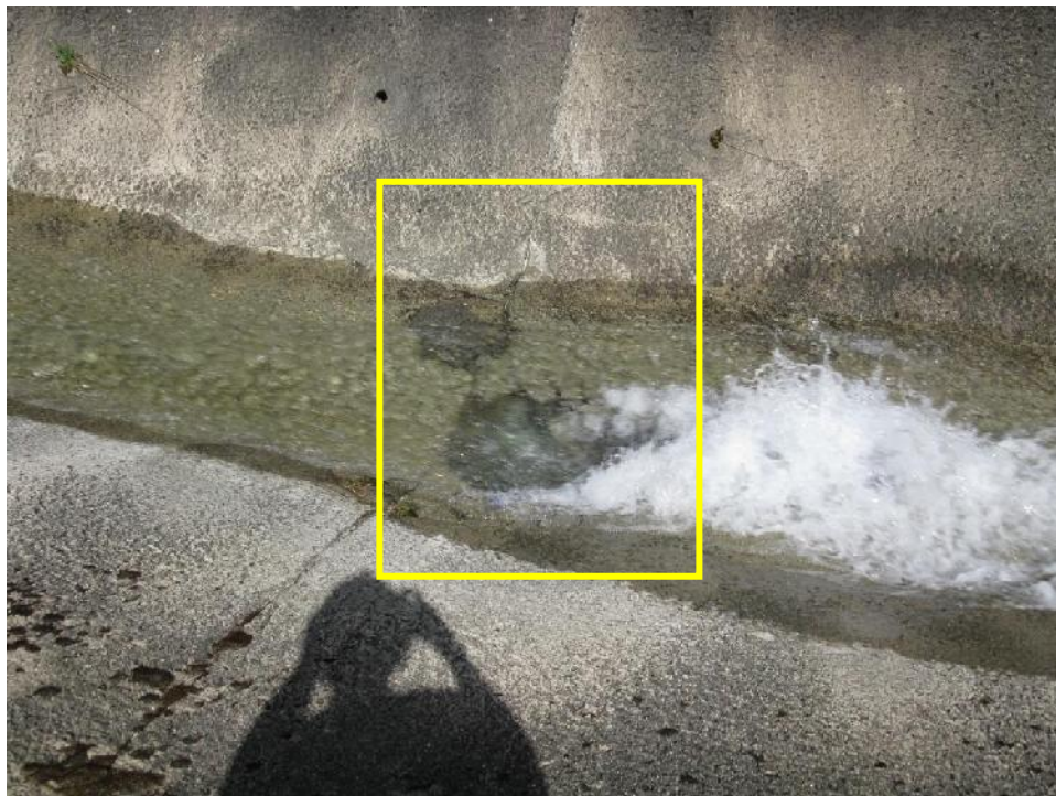
Photo 18 – Hole in Lower Lynx Diversion Ditch shotcrete liner.
