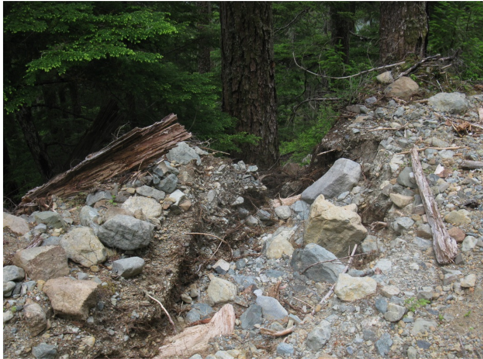
Photo 47: Lower Arnica Reach Ditch breach of the side of the slope caused by lack of freeboard (Taken June 17, 2015).
