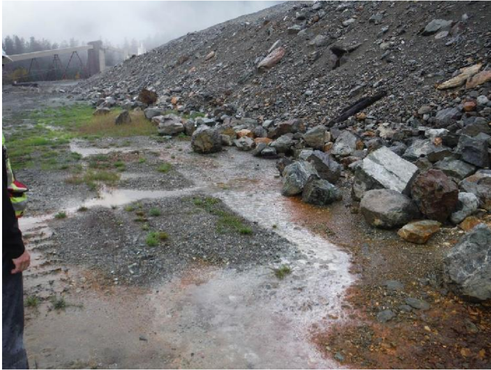
Photo 33 – Seepage on Lynx Dam “2011 Bench”, near Instrument Plane E.
