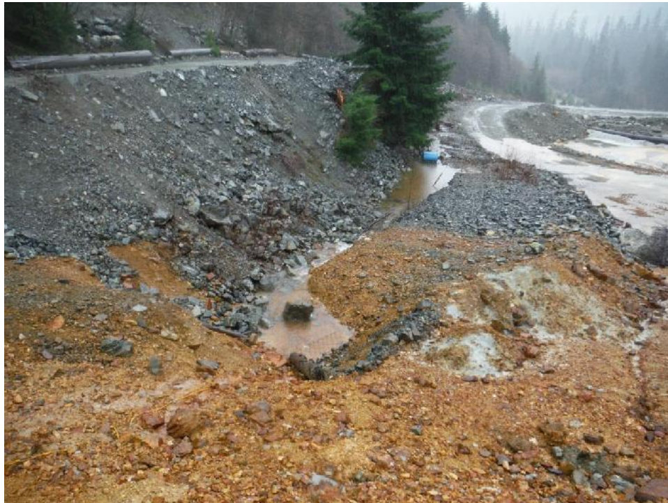
Photo 5 – High flow at the main spring on 2014-11-27 (toe of Paste Berm east abutment).
