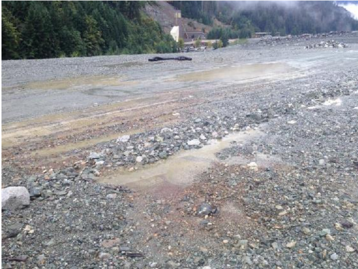
Photo 17 – Wet areas and puddles on the Seismic Upgrade Berm main bench near the access road between the RSA and the Strip, looking southwest.
