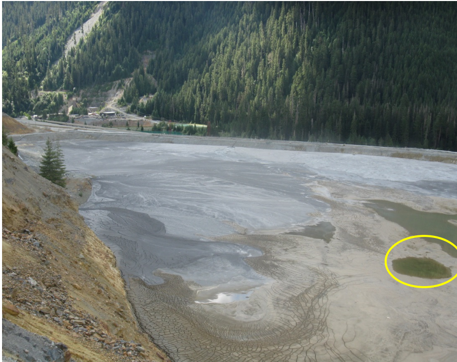
Photo 21: Overview of Lynx TDF in dry season, looking southeast, showing recurrent depression in yellow. Note tailings beach against south arm (July 23, 2015).
