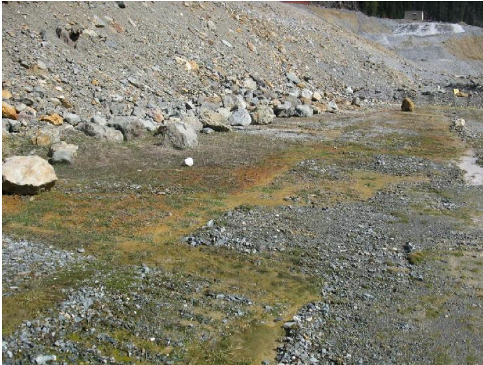
Photo 25 – Seepage and mossy area on the surface of Lynx Dam lower “2011 Bench” ~ Sta. 4+00, looking east/northeast.
