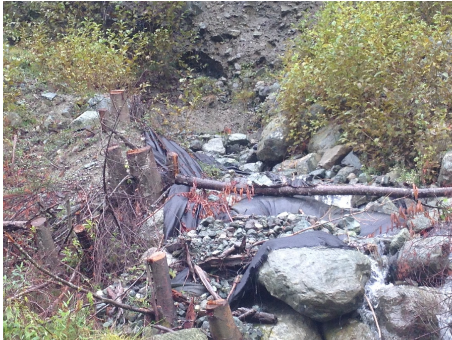
Photo 53: Debris at Alder Reach Ditch outfall into Lynx Lower Diversion Ditch (September 24, 2015).
