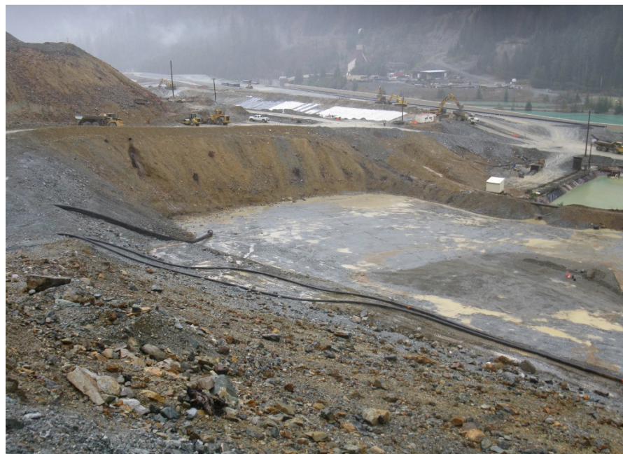
Photo 28: View of Lynx TDF panels area, looking southeast, showing improved drainage out of the south end due to a culvert leading to Super Pond (October 31, 2015).
