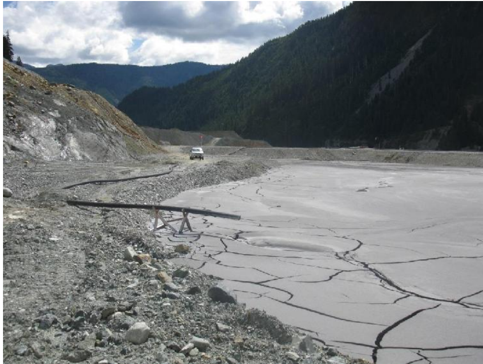
Photo 13 – Tailings surface and deposition point along the Springs Drain road, looking east.
