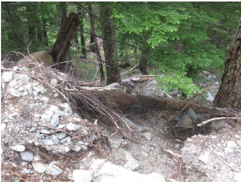
Photo 26 – Debris and fallen tree in breach along the lower reach of Arnica Ditch.
