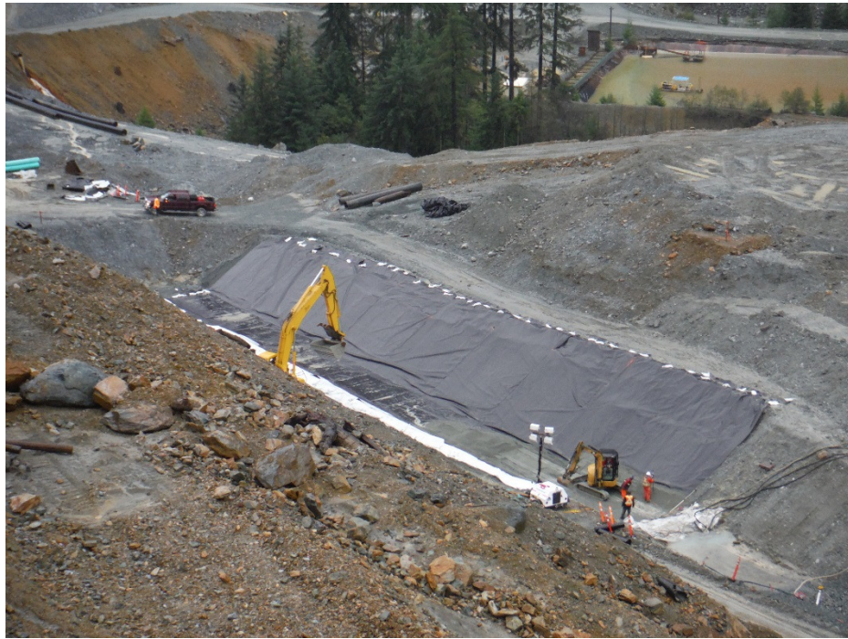
Photo 1: Construction of Lynx Springs Drain, going through the east arm of Lynx Dam, looking southeast (October 23, 2014).
