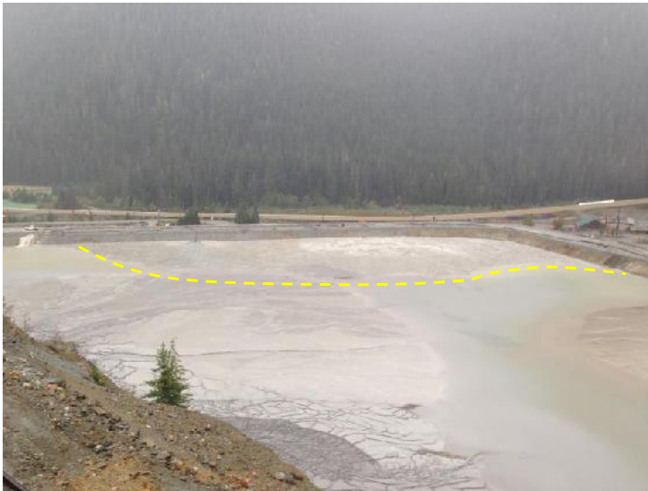
Photo 23 – Lynx TDF, looking south. Cracked area in the foreground is a paste tailings fan. The dashed line is delineating the sand beach above water. The recurrent depression in the paste surface is not visible.
