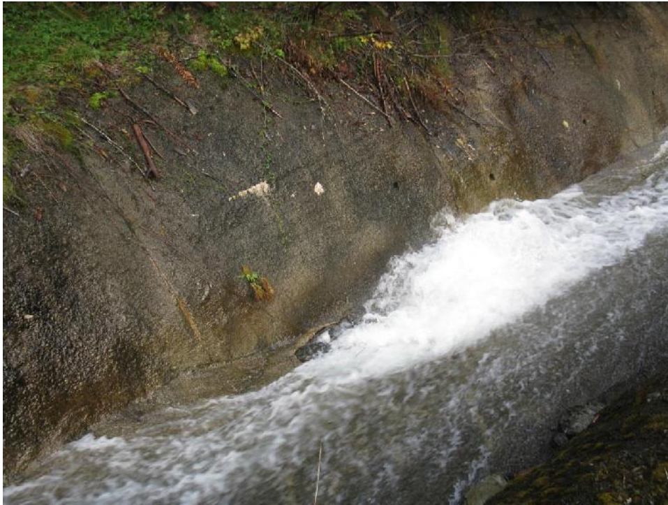
Photo 11 – Damaged shotcrete lining in the Lower Lynx Diversion Ditch.
