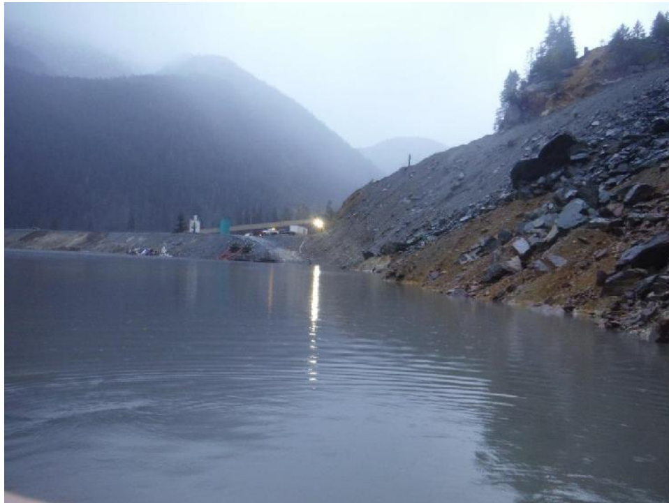
Photo 17 – Significant ponding of water in Lynx TDF on 2014-11-27, two diesel pumps present at the west arm. Photo taken from boat near pit highwall.
