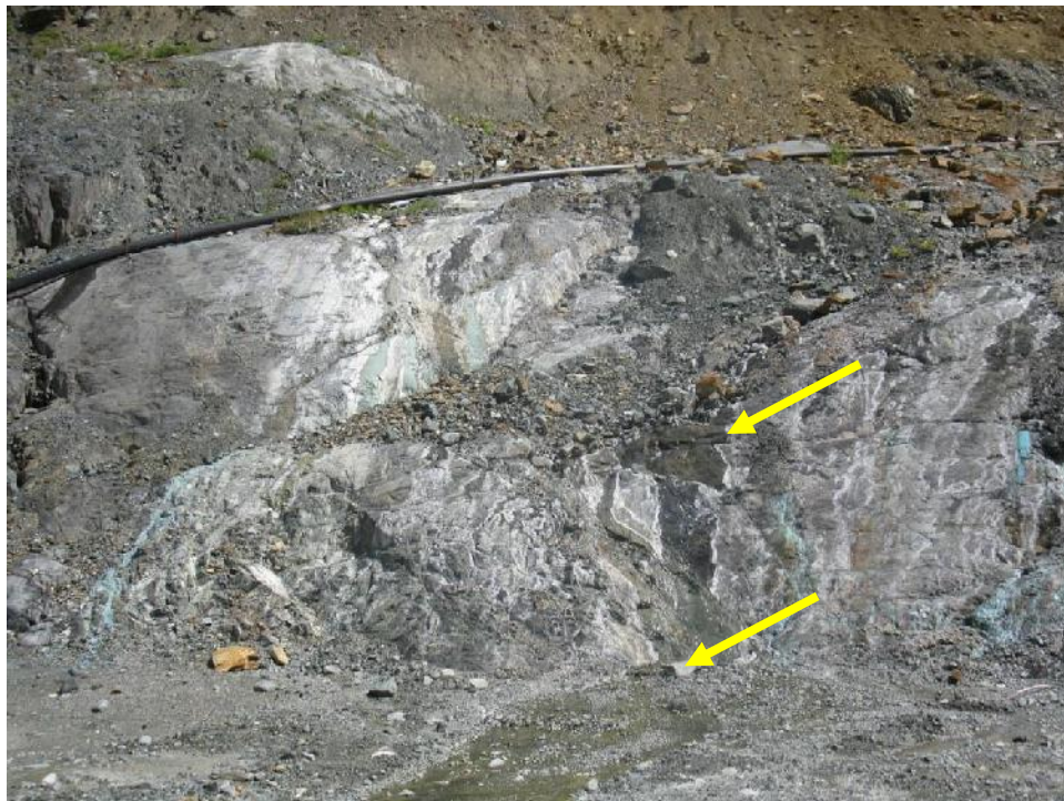
Photo 14 – Trace seepage entering Lynx Pit at rock wall above the springs drain, looking north.
