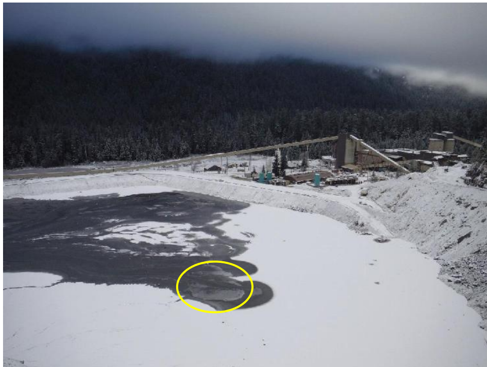
Photo 12 – Overview of Lynx TDF, looking southwest (recurrent depression in paste circled).
