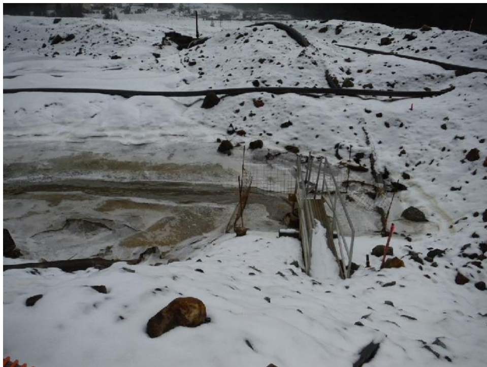
Photo 6 – Strip decant structure.
