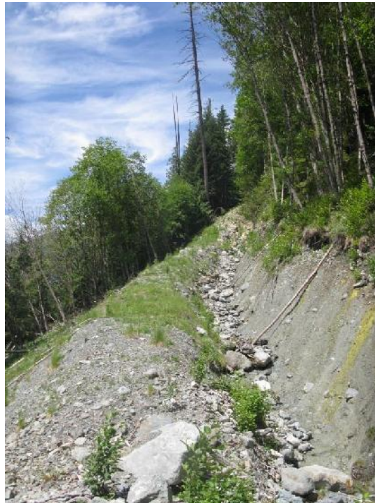
Photo 19 – Alder Reach with some rock debris along invert, looking west.
