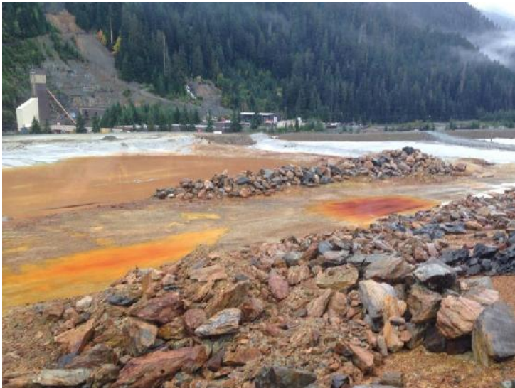
Photo 10 – Red ARD staining at the base of the Paste Berm and ponded water in the East Strip on the east side of the Old TDF spillway, looking southwest.
