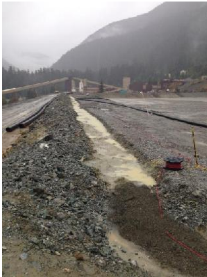
Photo 27 (left) – Trench in upstream half of Lynx Dam crest to route piezometer wires. Photo 28 (right) – Cracking at the contact of the Zone J core and the upstream dam shell.
