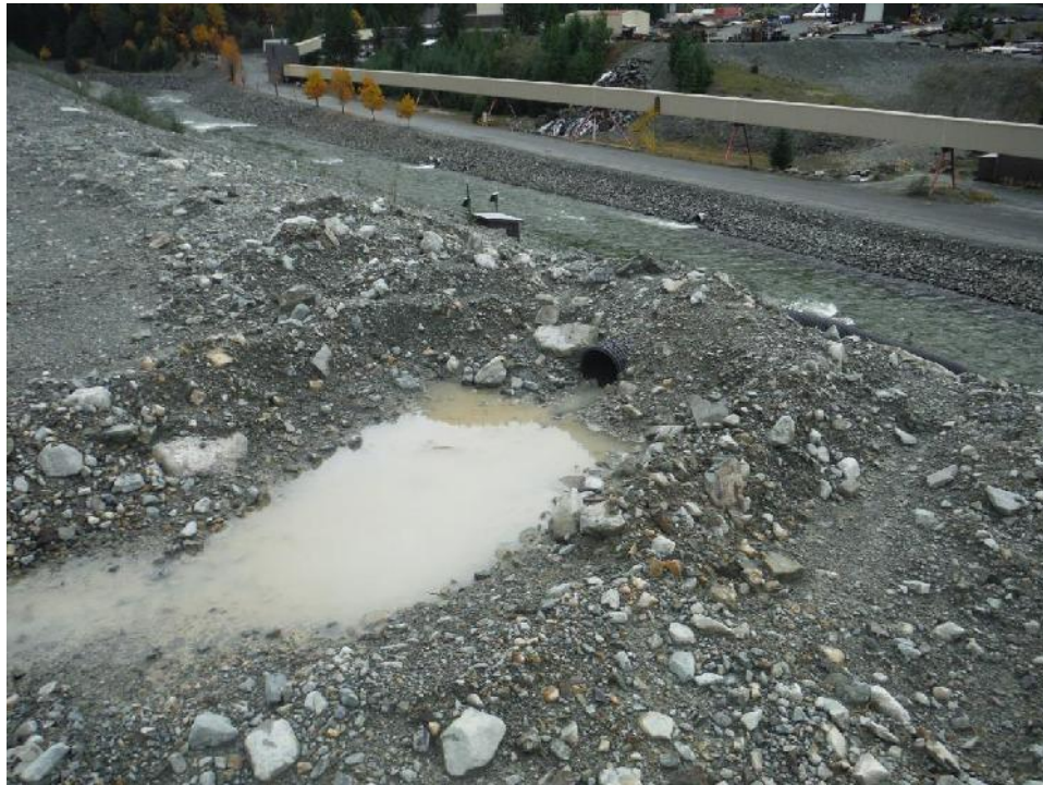
Photo 21 – Ditch and drainage pipe on top of the Seismic Berm downstream face, looking southeast near Instrument Plane A (Hut A and Myra Creek in background)
