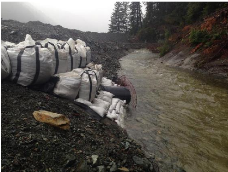
Photo 18 – Temporary water diversion upstream of the Lower Lynx Diversion Ditch (near Cascade Reach), looking west.
