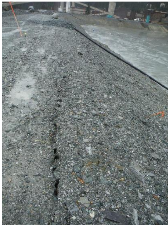
Photo 26 – Tension crack on the south arm downstream crest of Lynx Dam, approx. Sta. 3+50.
