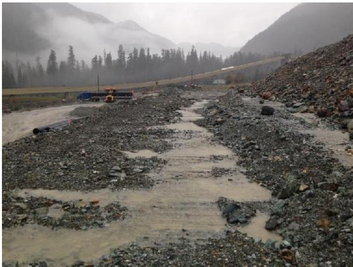
Photo 37 – Seepage and surface runoff on Lynx Dam mid-level bench, looking west.
