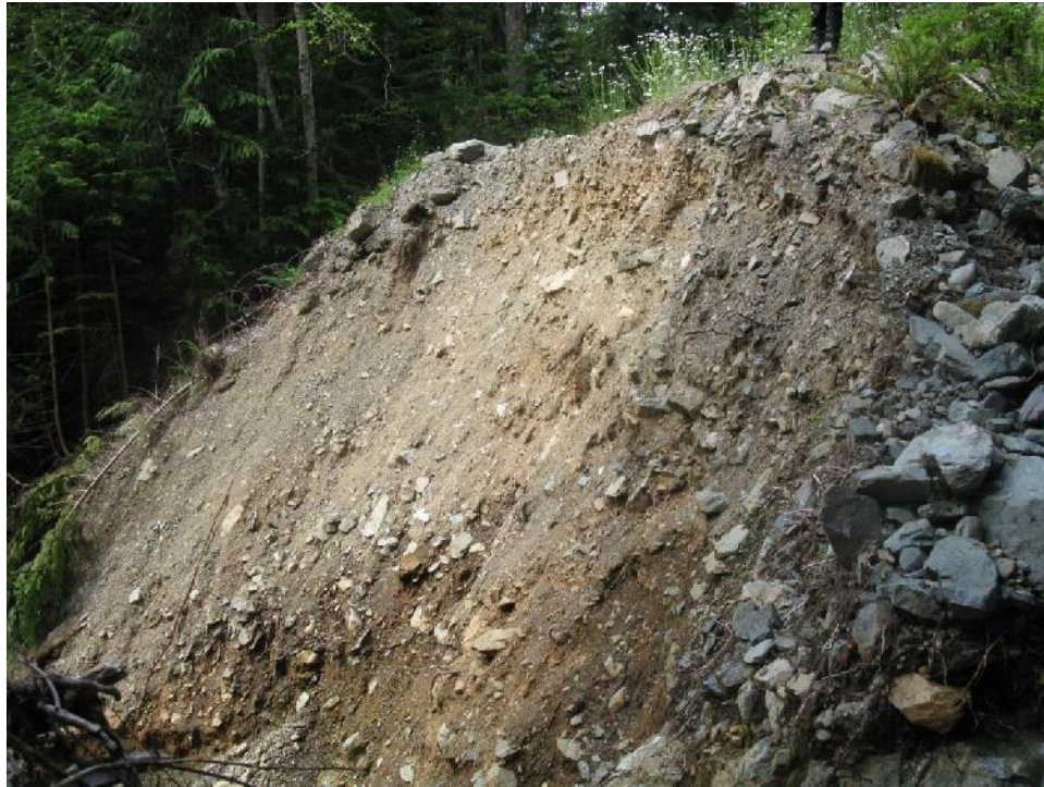
Photo 45 – Headscarp of failure area looking south from the diversion channel.
