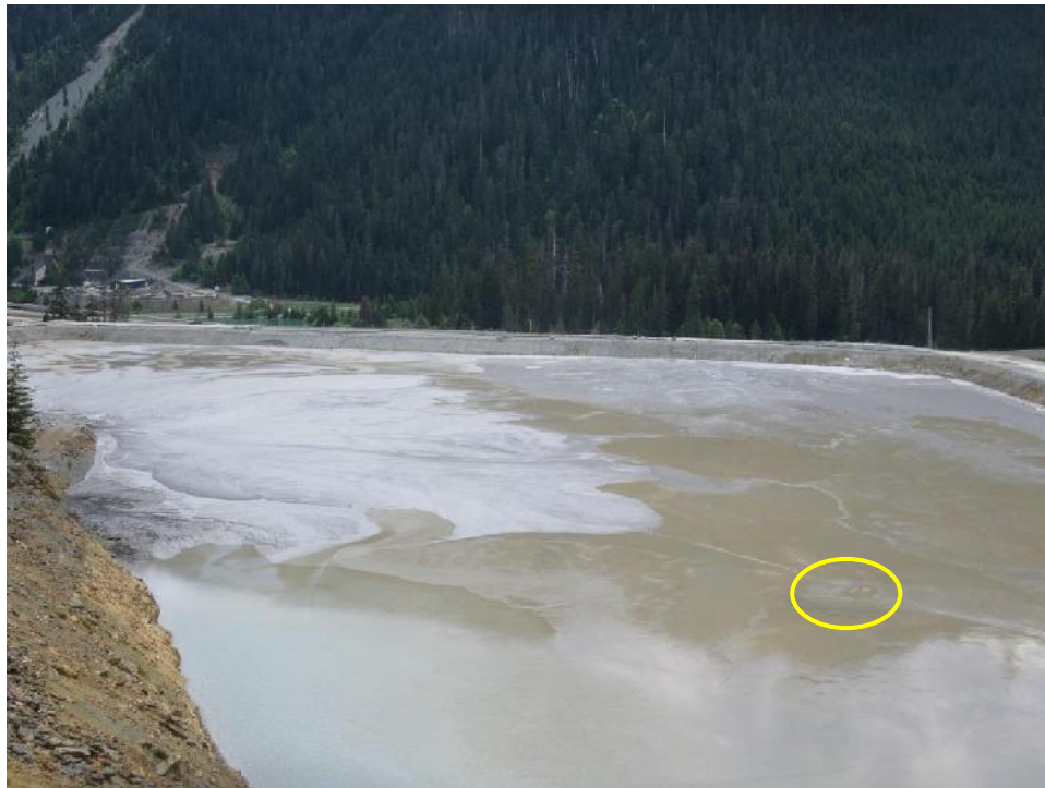
Photo 21 – Overview of eastern portion of Lynx TDF, looking south/southeast. Recurrent sinkhole marked with circle.
