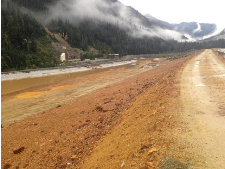
Photo 9 – Wet areas at the base of the Paste Berm and ponded water in the East Strip, looking west from the Paste Berm crest near Instrument Plane C.
