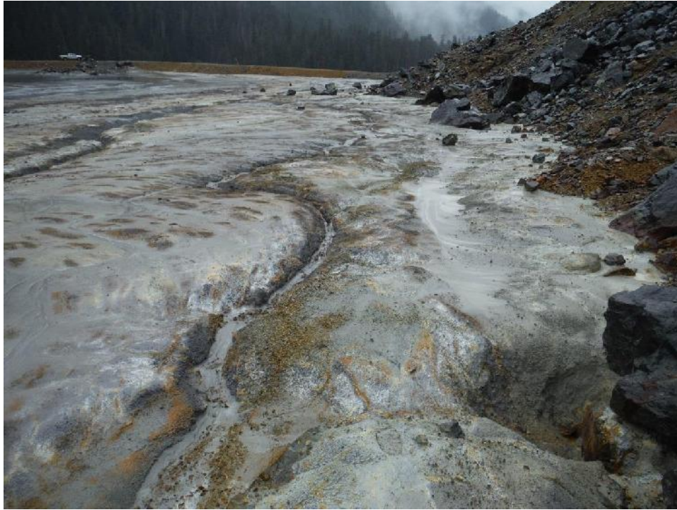
Photo 3 – Erosion holes and rills in the APA paste tailings at the Waste Dump #6 west side toe.
