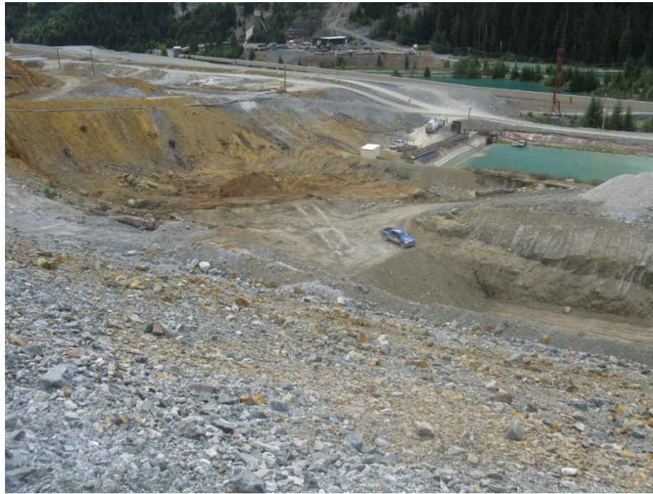
Photo 25: Toe area of Lynx Dam south arm. Phillips Reach sump has been taken out. Foundation panel construction ongoing (July 23, 2015).
