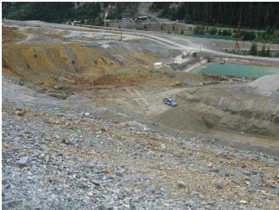
Photo 18 – General view of the southeast corner of Lynx Dam toe, looking southeast. The treed area around Phillips Reach sump was cleared and organics were removed.
