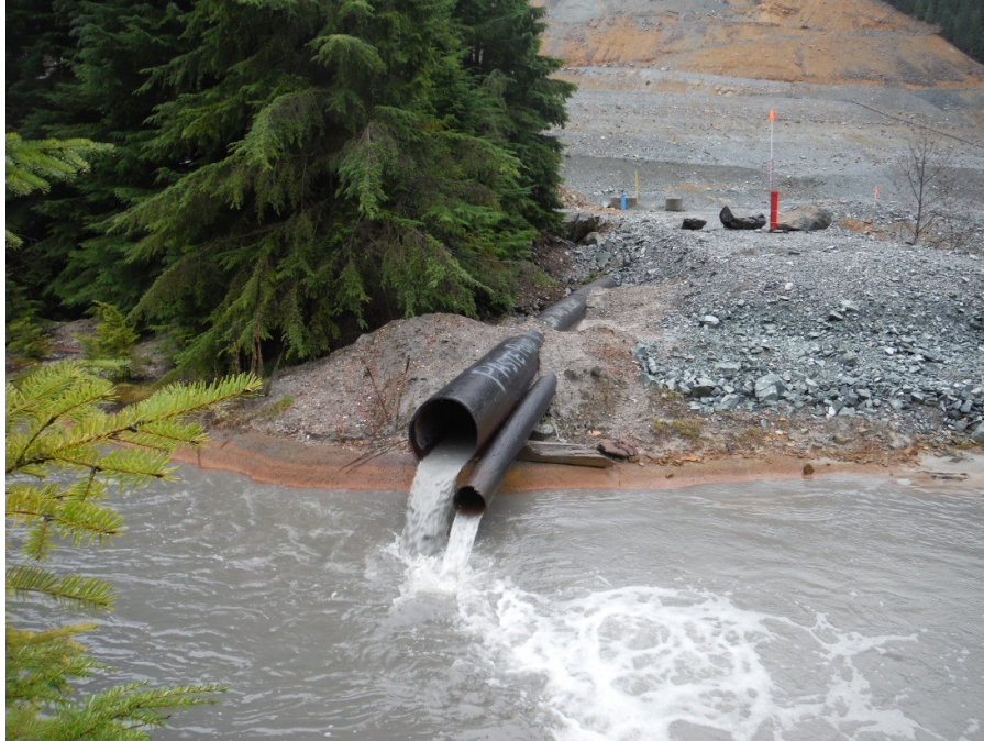
Photo 17: APA (large diameter) and RSA/Strip decant (small diameter) pipes discharging into Superpond 'In' channel (February 9, 2015).
