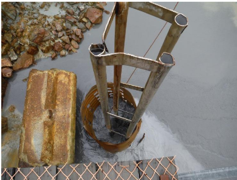
Photo 20 – Turbid water flowing into the RSA decant structure.
