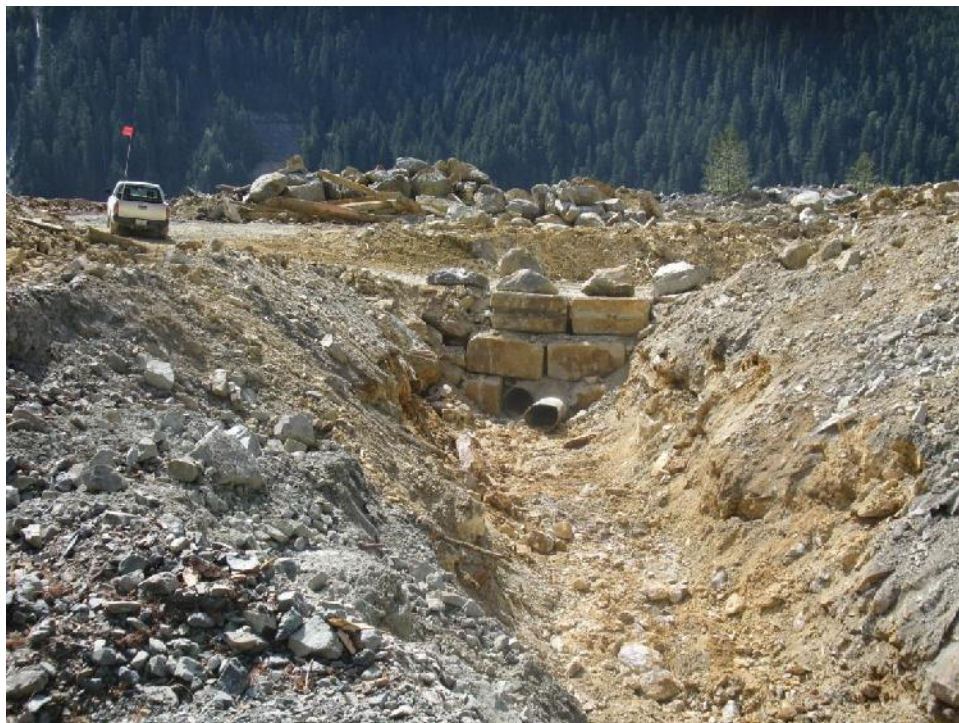
Photo 12 – Culverts across the access road at the head of the temporary water diversion for Lower Lynx Diversion Ditch upgrade works, looking south towards Waste Dump #6.
