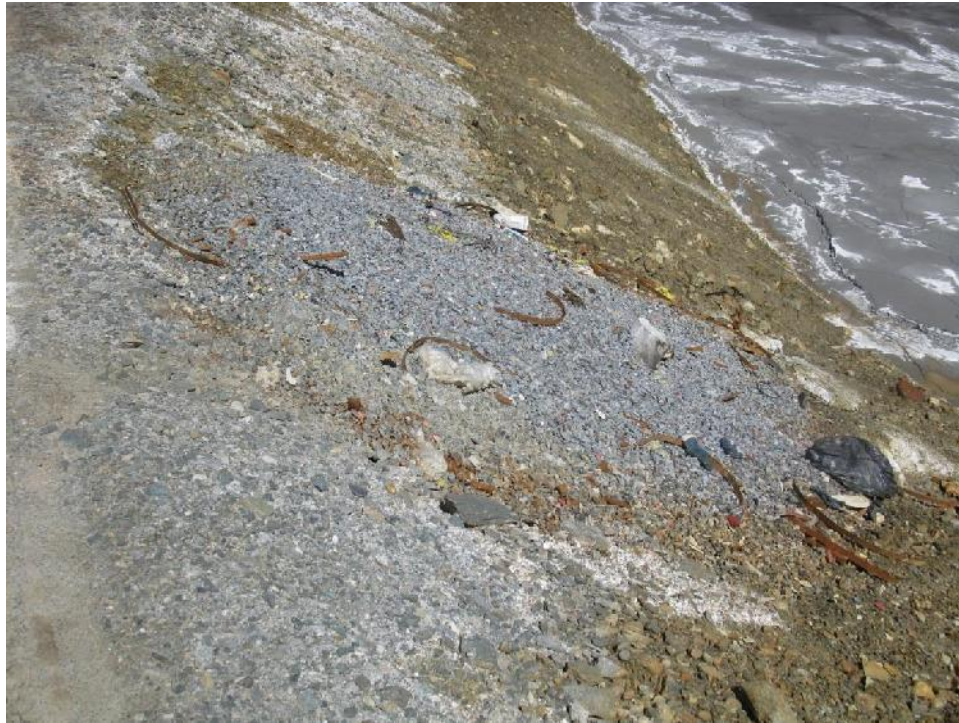
Photo 17 – Mine refuse on the upstream face of Lynx Dam west arm (southwest corner of the facility) (on 2015-06-16).
