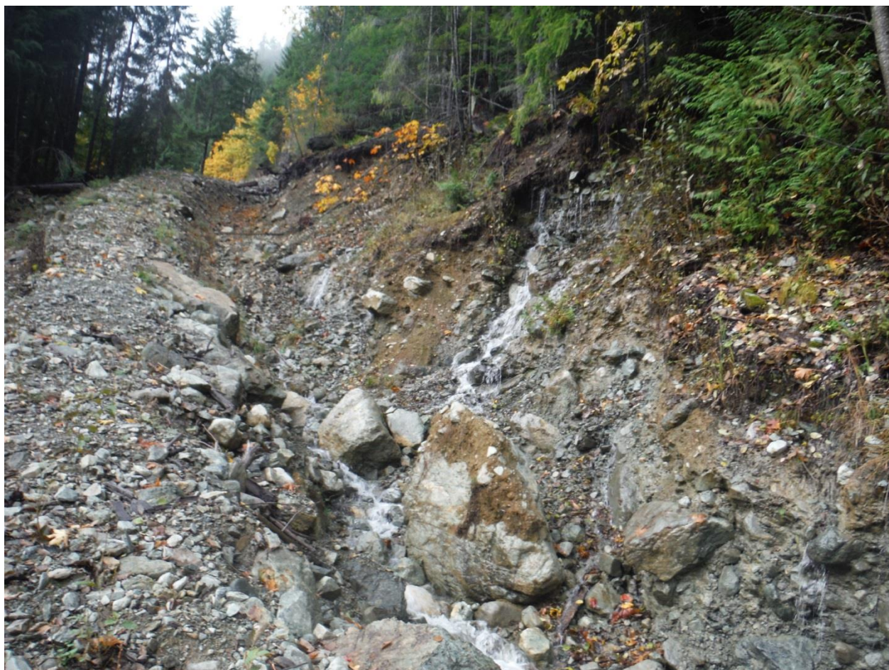
Main source of water at about 1+05, in coarse colluvium, October 2014. A drainage swale will be required at this location or slightly below.
