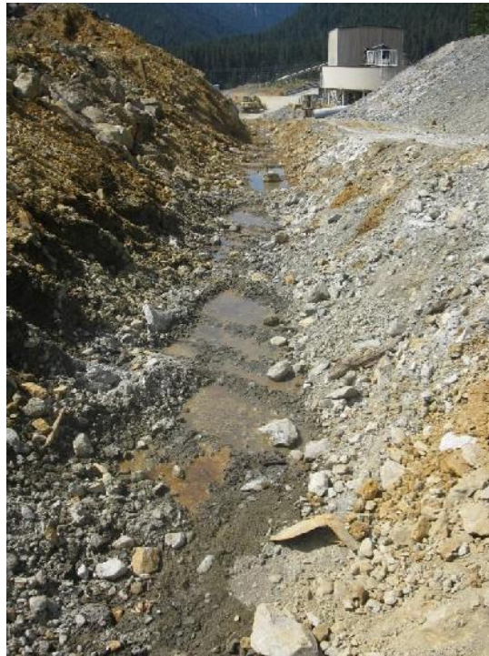
Photo 13 – Construction diversion along the access road for Lower Lynx Diversion Ditch, looking west towards Paste Plant. Seepage appears to be draining from the waste dump.
