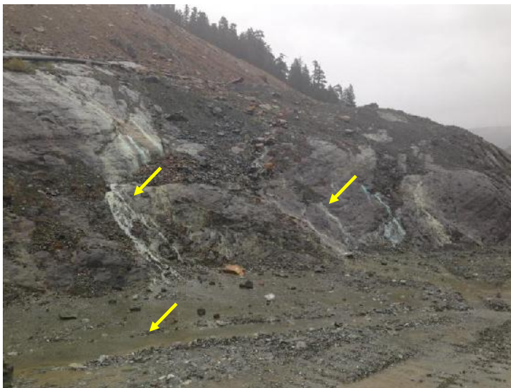
Photo 29 – Springs and surface runoff coming from the rock wall at the back Lynx Pit, looking northeast. Water reporting on the top of Lynx Springs platform.
