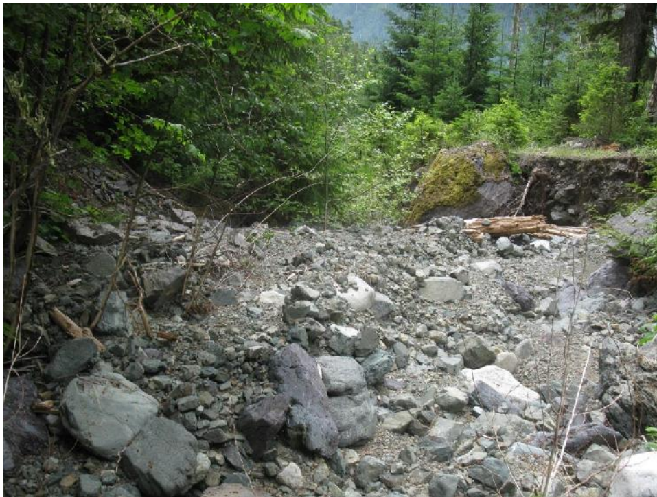
Photo 28 – Debris in the Upper Lynx Diversion Ditch just below the culvert section, looking downstream. Debris and erosion of the ditch is from the torrented stream in Photo 36 & 37.
