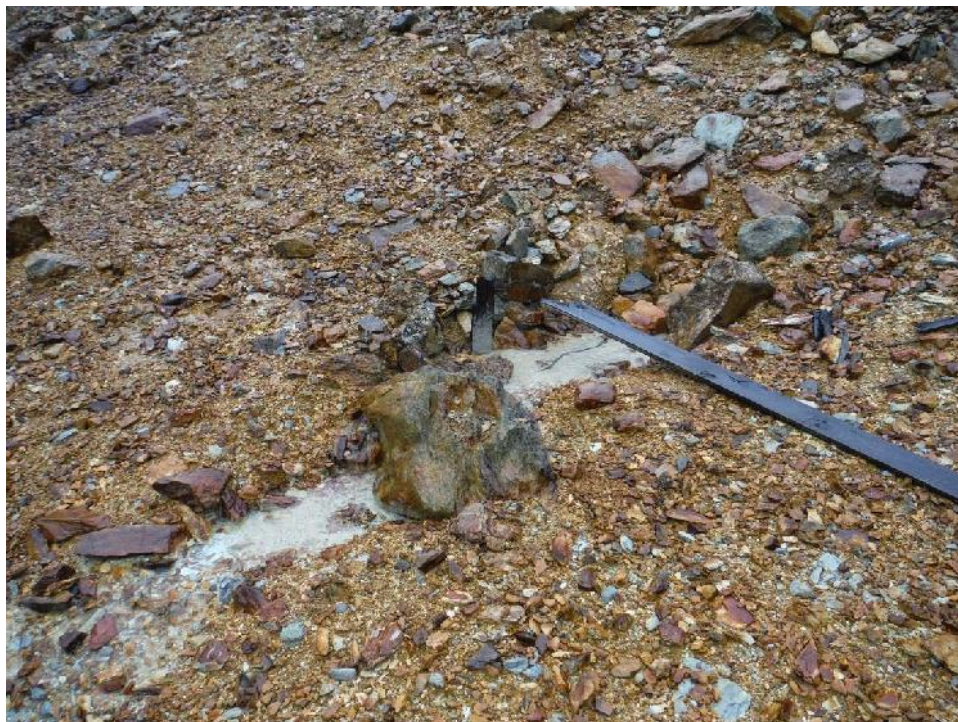
Photo 4 – Close-up view of the discrete seepage source along the east arm of the Paste Berm (photo taken on 2014-11-27).
