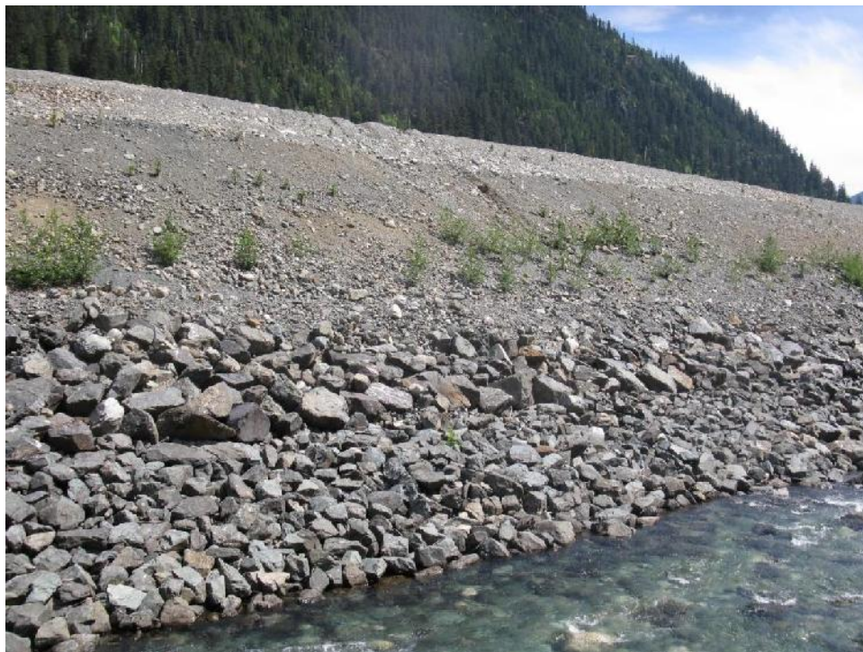
Photo 16 – Series of erosion rills on the Seismic Berm downstream face.
