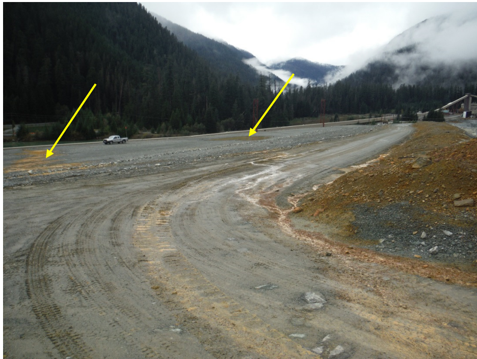
Photo 5: Areas of ARD seepage on the Seismic Berm caused by runoff from the access road between the West Strip and the RSA, looking southwest (October 23, 2014).
