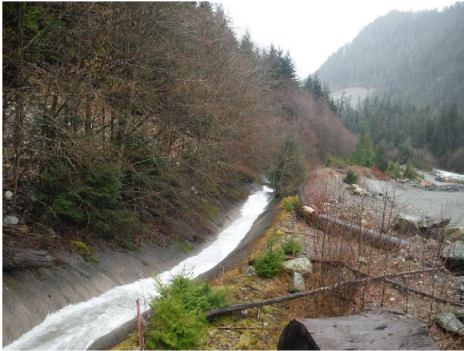
Photo 9 – Shotcrete lined section of Lower Lynx Diversion Ditch, about 50 m upstream of Alder Reach.
