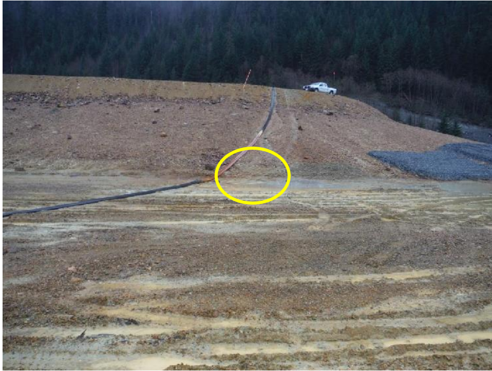
Photo 13 – Southeast corner of the Paste Berm, looking north. The base of the Paste Berm is soft and saturated due to poor drainage and distributed seepage.
