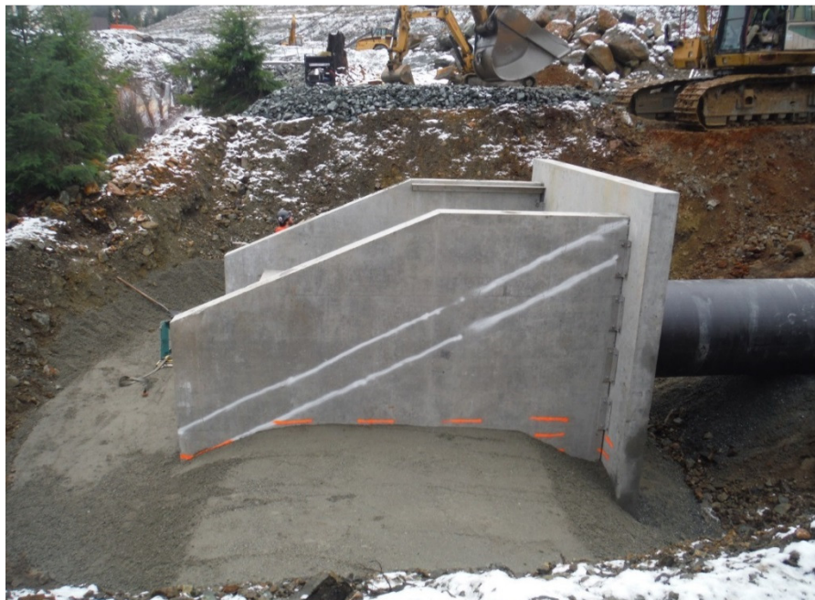
Photo 56: Energy dissipater at the end of the decant pipeline (December 15, 2015).
