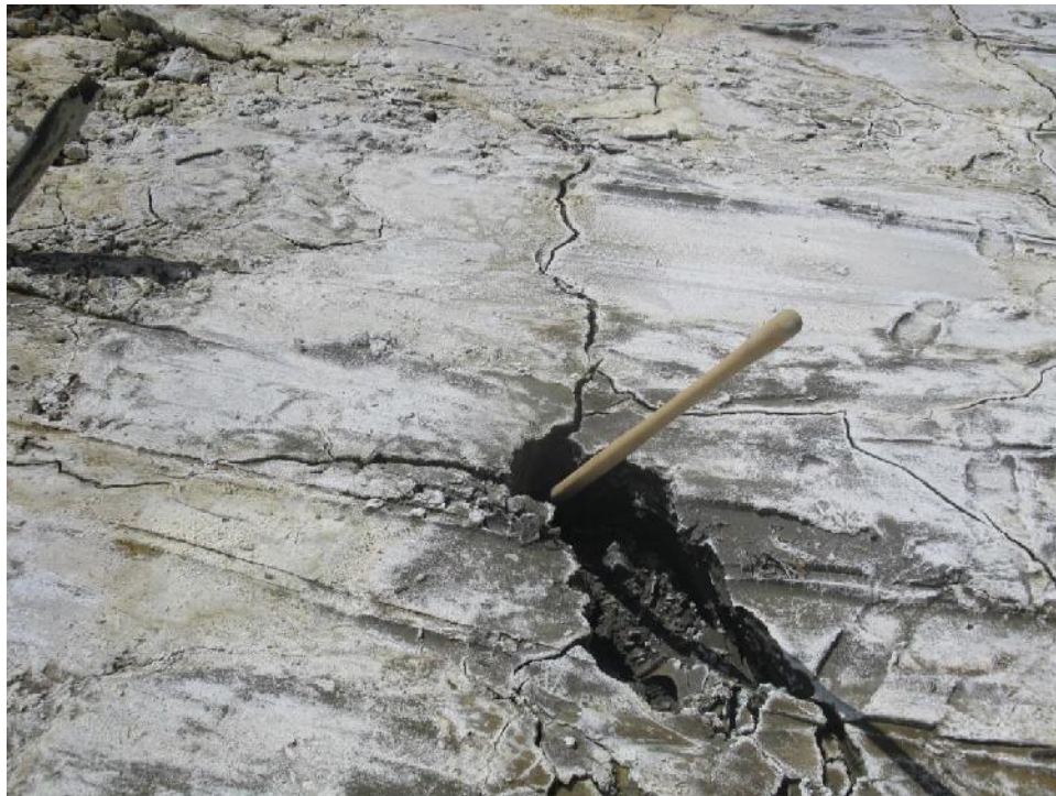
Photo 4 – Hole in the invert of the access road ditch. Shovel inserted into hole for scale.
