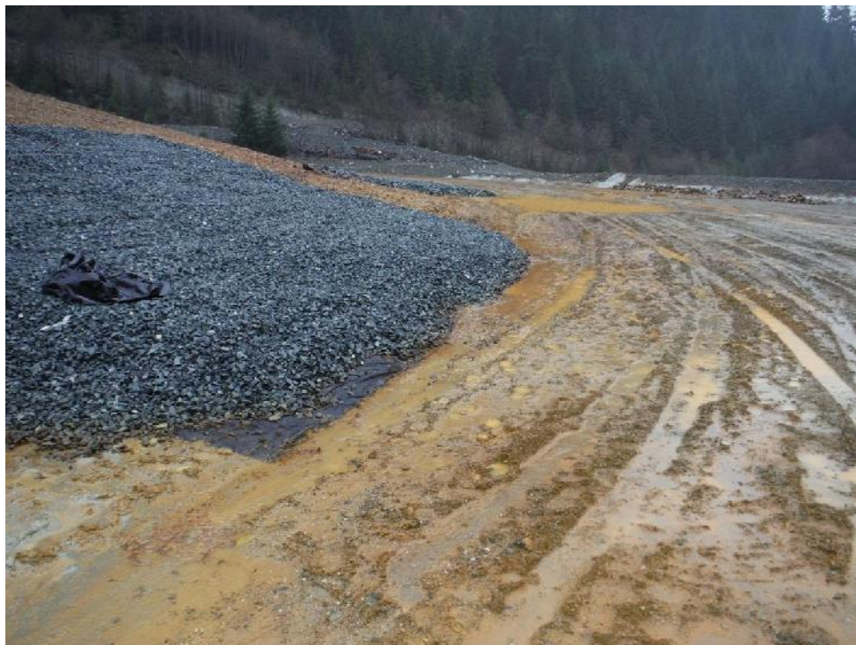
Photo 10 – Saturated soil and water pooling in ruts at the base of the Paste Berm, looking northeast.
