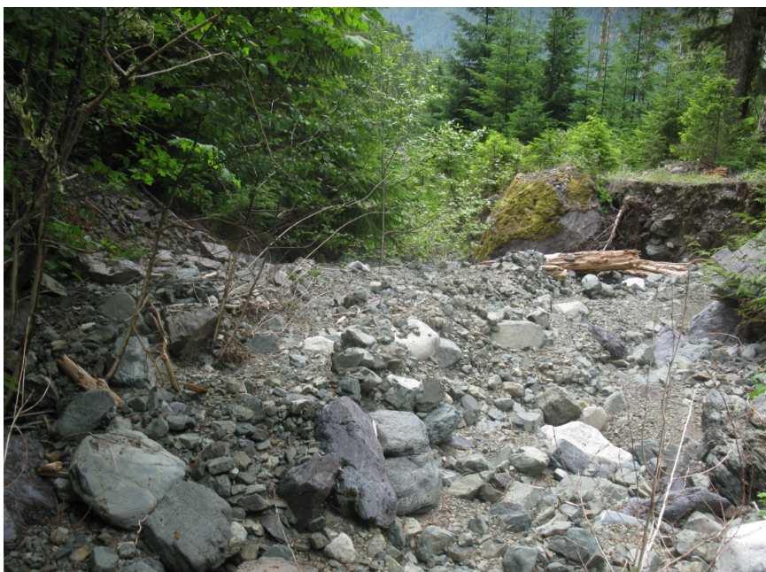
Photo 52: Debris blocking the Upper Lynx Diversion Ditch, looking downstream (June 17, 2015).
