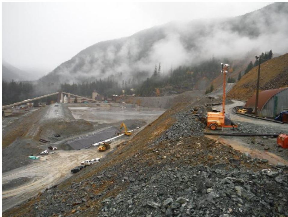
Photo 28 – Section of Lynx Springs Drain going through Lynx Dam east arm under construction, looking west.
