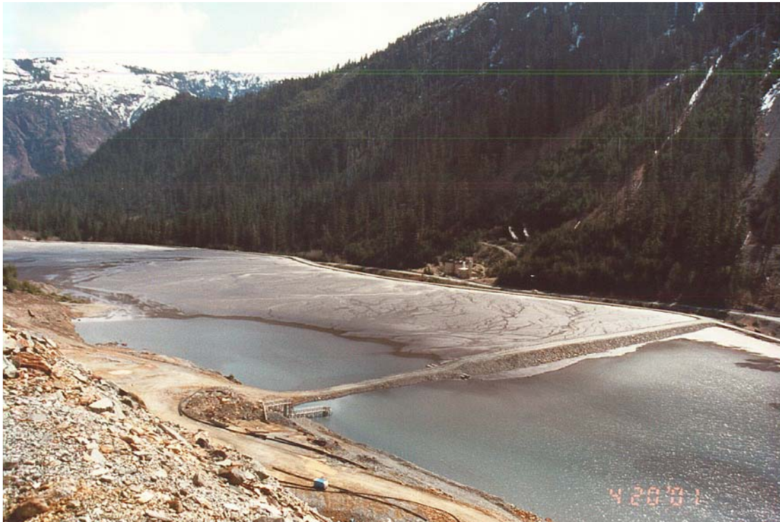
Photo 2 – Boliden Myra Falls Operation – Tailings ponds. Under permit with the Ministry of Environment Lands and Parks, the water is treated by lime addition and settling prior to discharge to Myra Creek
