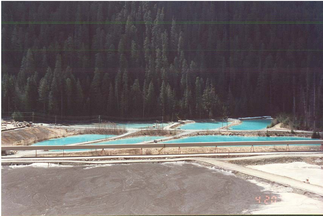
Photo 4 – Boliden Myra Falls – Six Myra solids settling and polishing ponds
