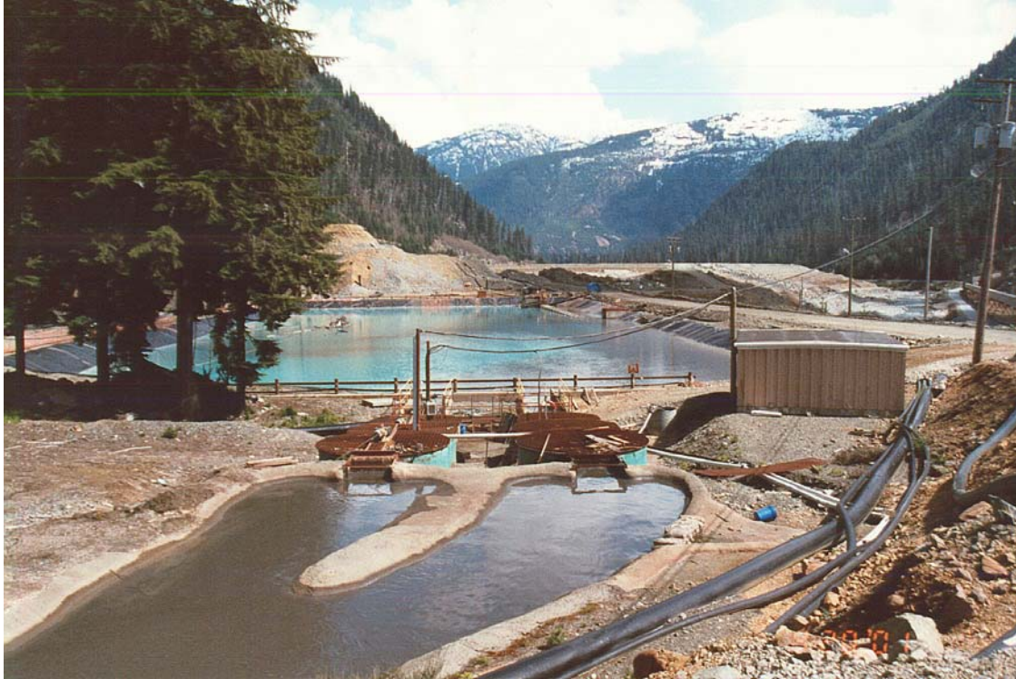
Photo 3 – Boliden Myra Falls operation – Mine drainage and tailings ponds water treatment and super pond
