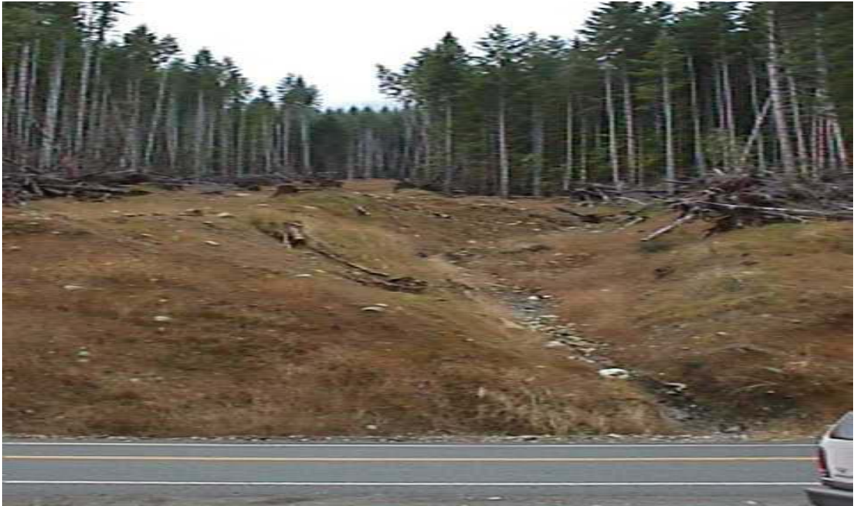
Photo 13 - Slope failure of unknown origin reseeded by landowner
